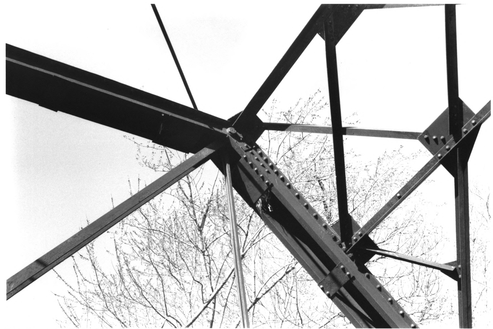
Bridge no. 90980 Co. Rd. 190 over the north fork of Crow River Meeker Co. Oia 208-4415
