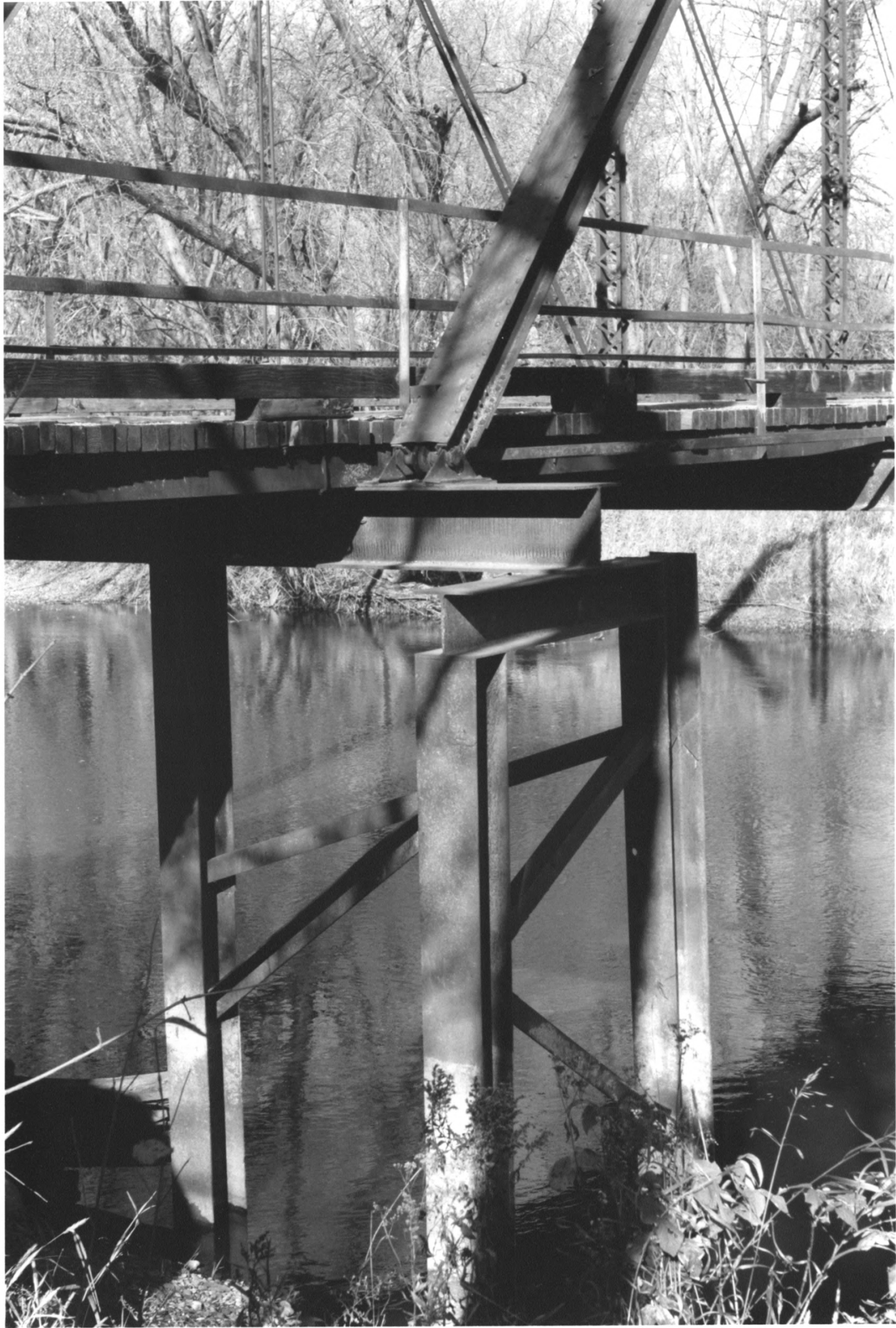
Bridge No. 90980 Co. Rd. 190 over The north fork of Crow River Meeker Co.
