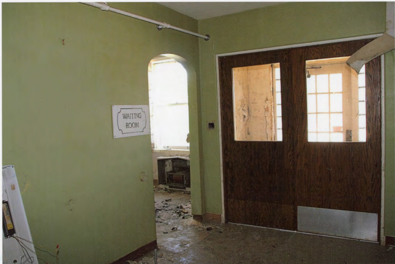
St. Thomas Hospital, Colby, Thomas County, KS
