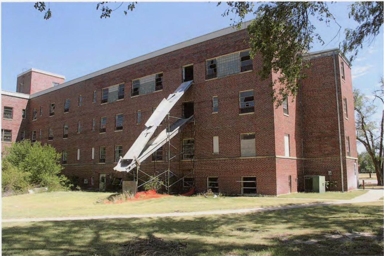
St. Thomas Hospital, Colby, Thomas County, KS
