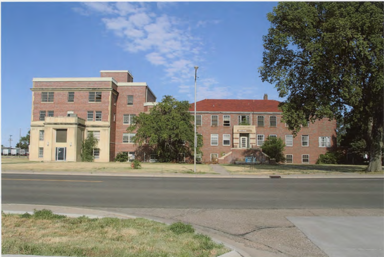
St. Thomas Hospital, Colby, Thomas County, KS
