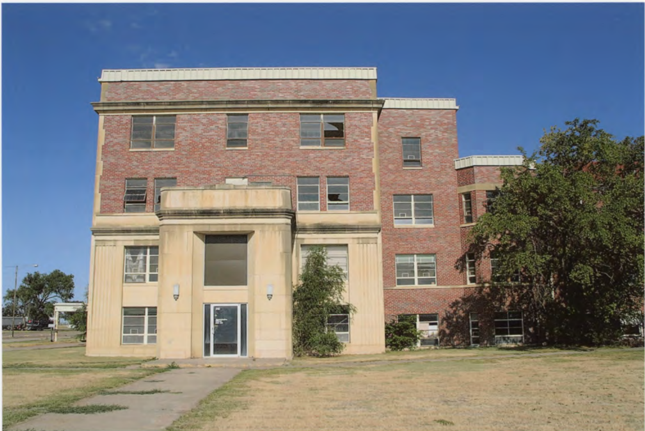
St. Thomas Hospital, Colby, Thomas County, KS
