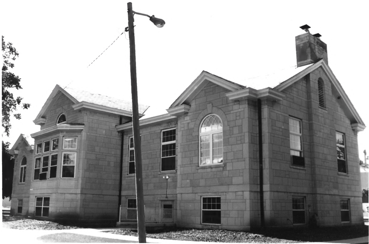
#7 WITTEN MEMORIAL BUILDING, NEWTON CO. INDIANA
