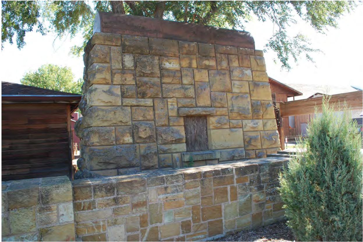
Tool Storage building, looking east-southeast 12 of 13
