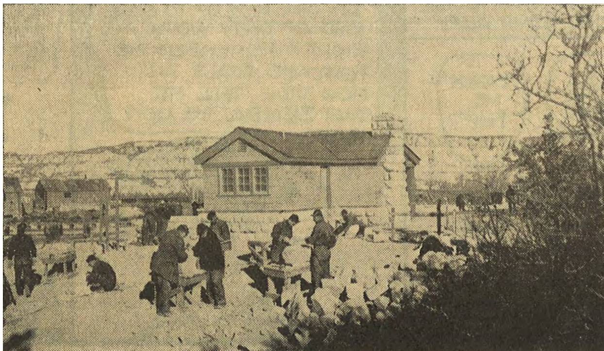
An undated newspaper clipping "Rock Shaping Crew At Work" on file in the ND State Archives shows men shaping stone for the contact station at the Chateau de Mores.
