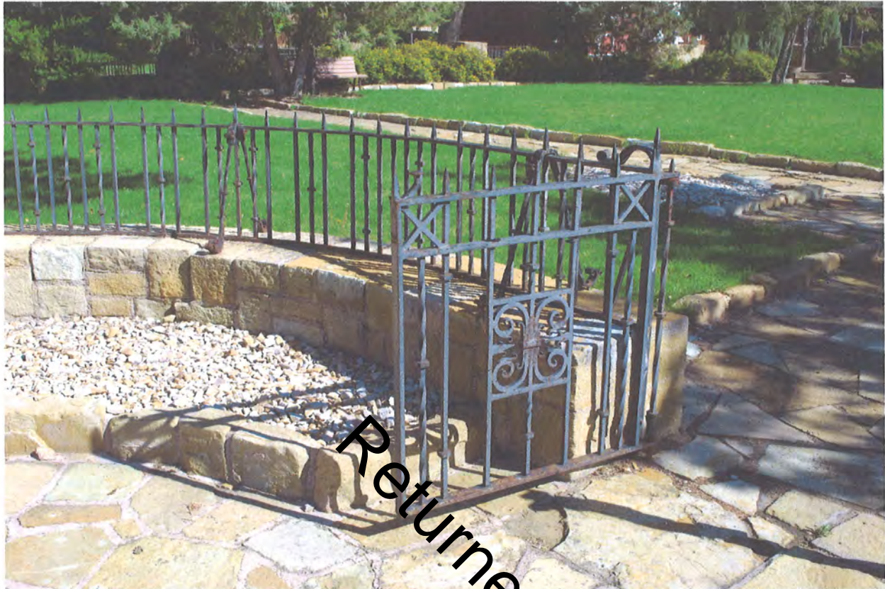
Gate detail, looking northeast 4 of 13
