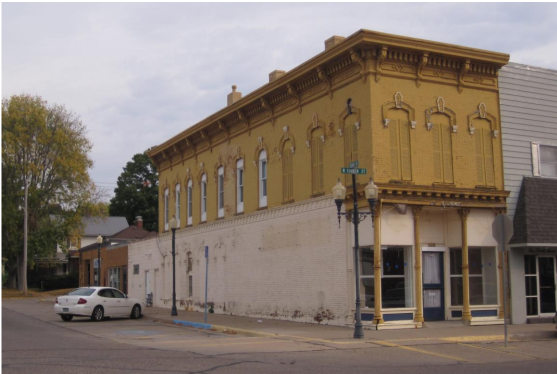
Figure 6 The 1876-1877 Star Drug Store (129 4 th St. W.) is a corner building with both elevation cornices intact as well as several original chimneys. Tallgrass Historians LC, 2015
