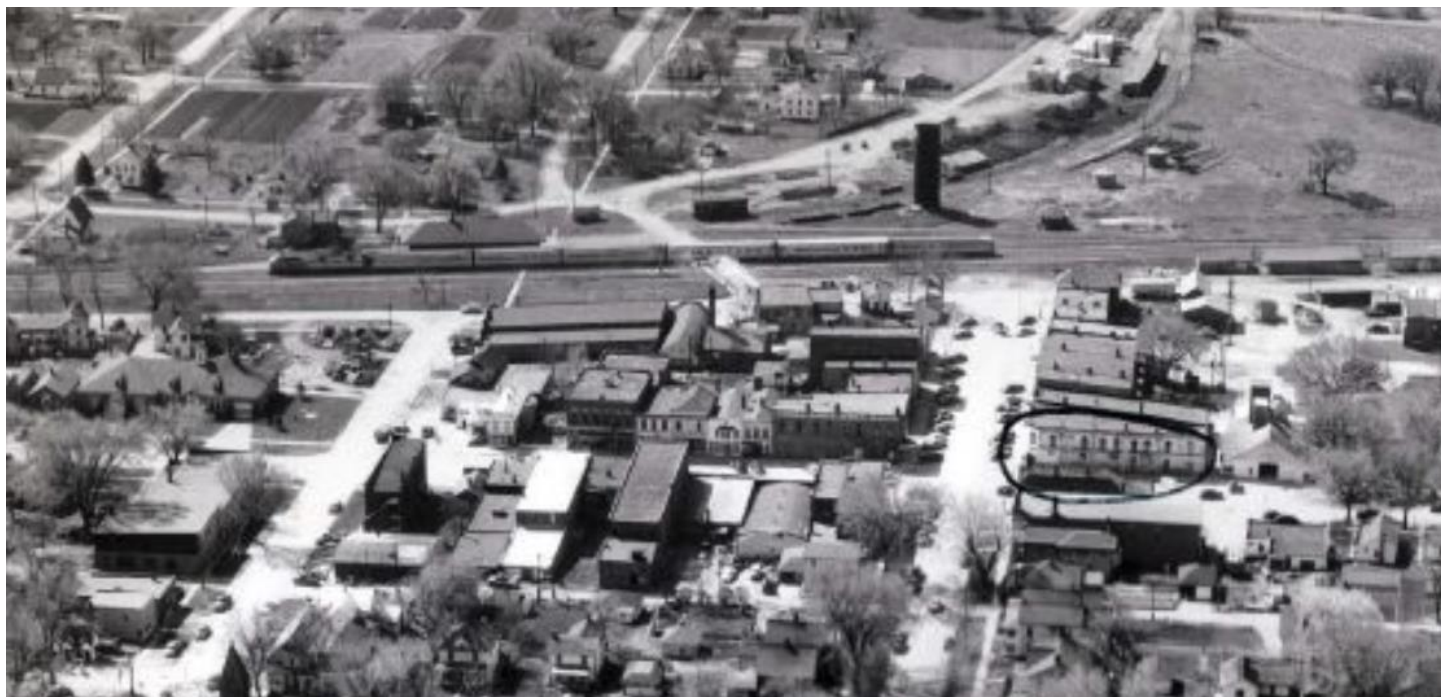
Figure 23 Circa 1953 aerial view of the commercial district and the Rock Island railroad depot (behind train), tracks, and standpipe (nonextant), looking south. The WPA-funded town hall is center left. The circle around 325 Cedar Street (C.B. Strong's Dry Goods; Lamp's Groceries and Dry Goods) is on the original photo. That Cedar Street building is covered completely by metal siding now. A similar 1953 view but taken after the plane had circled around to the south of the town is seen in Fig. 12. Provided by the Wilton Development Corporation
