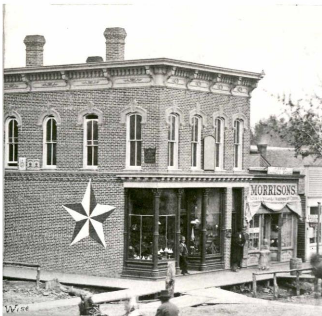
Figure 16 Star Drug building, ca. 1880. The lower, windowless side wall accommodated the interior placement of shelving, bins, and counters. Provided by the Wilton Development Corporation
