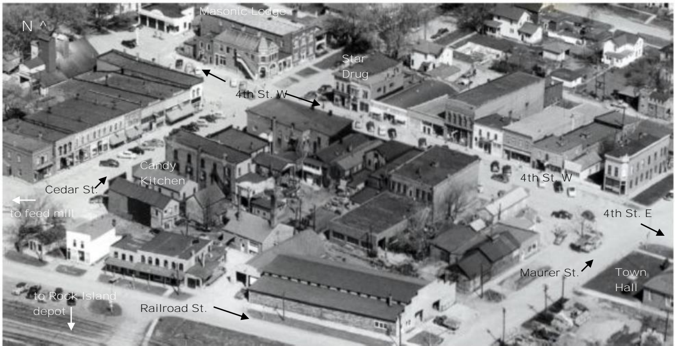
Figure 12 1953 aerial view of the Wilton commercial district, looking northwest. The east end of the district beyond Maurer Street is not visible in this photograph. A number of the buildings seen here, especially along Railroad Street are nonextant, replaced by cheese factory buildings shortly after this photo was taken. See Fig. 23 for a similar 1953 view taken from the north side of town looking toward the south. Provided by the Wilton Development Corporation
