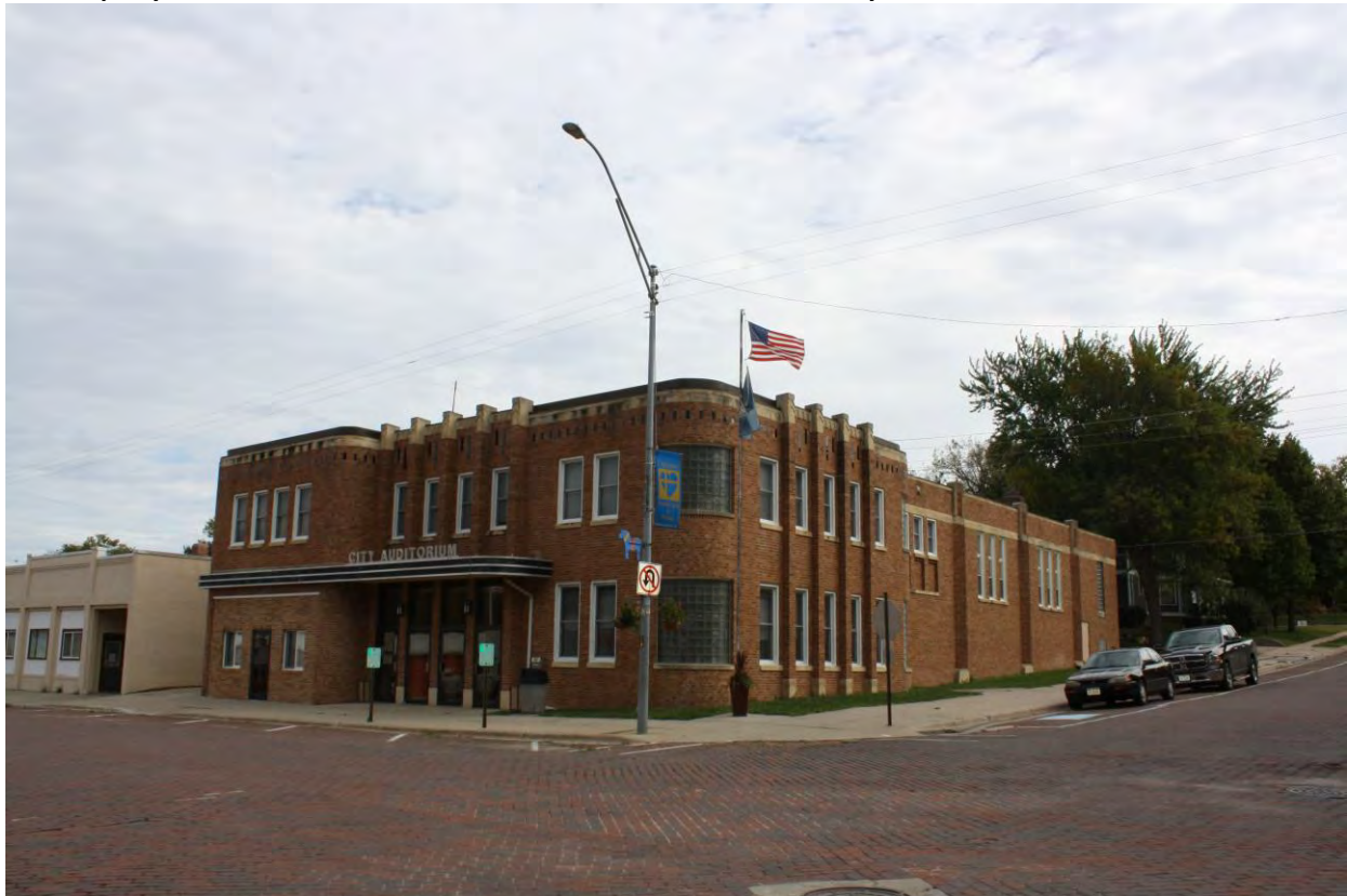
2. View showing west and south elevations at intersection of Oakland Avenue and 4 th Street; view northeast.
