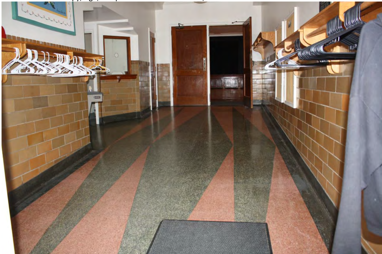
7. Interior corridor leading to auditorium showing terrazzo floors and looking east.
