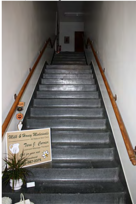
13. Interior terrazzo stair leading to second floor library, community room, and balcony. View looking east.
