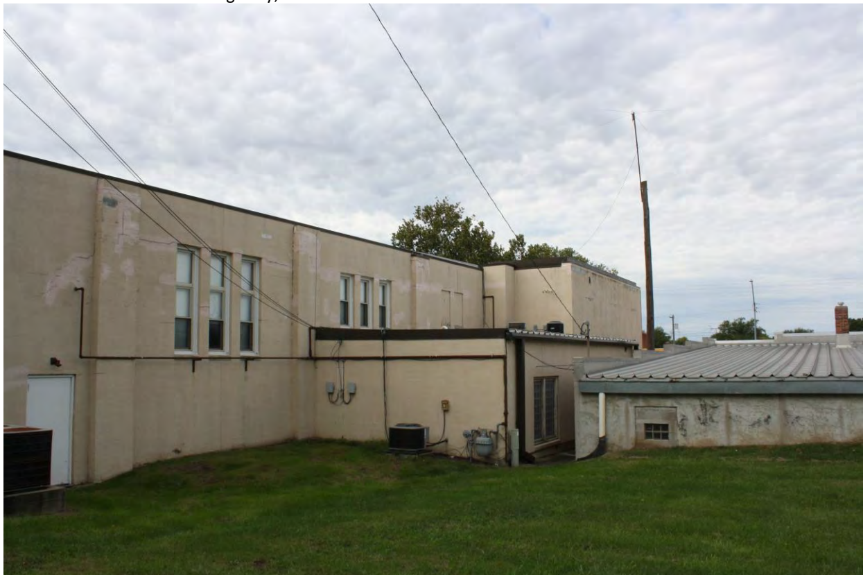
5. View of north elevation; view southwest.
