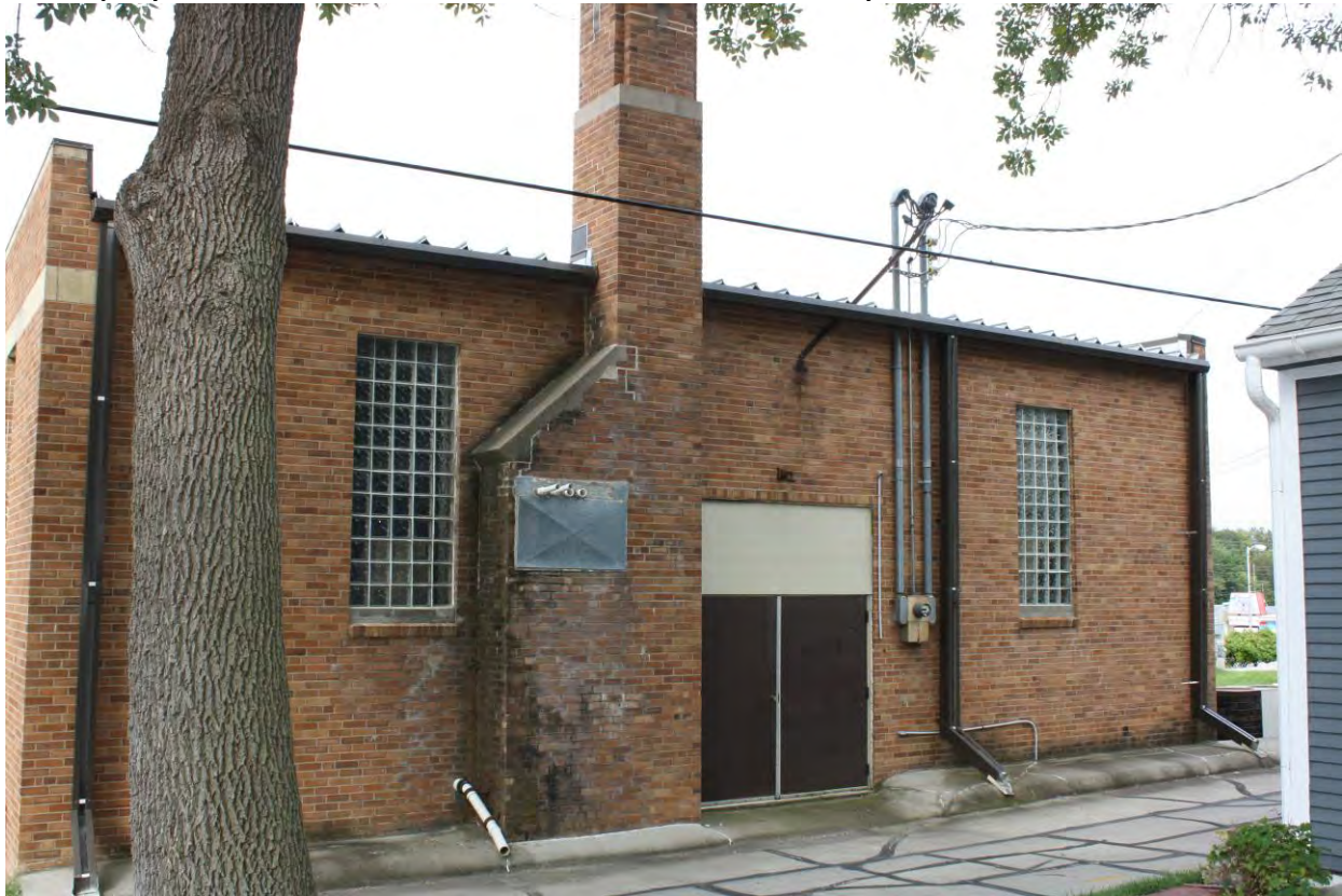
4. View of east elevation facing alley; view west.
