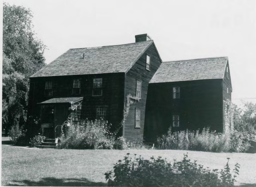
Balch House, 1639-50 West (Rear) Elevation and South End (Right)
