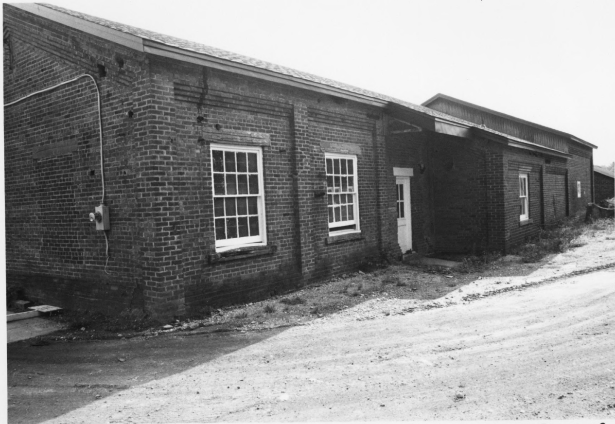
STERLING HILL MINE
