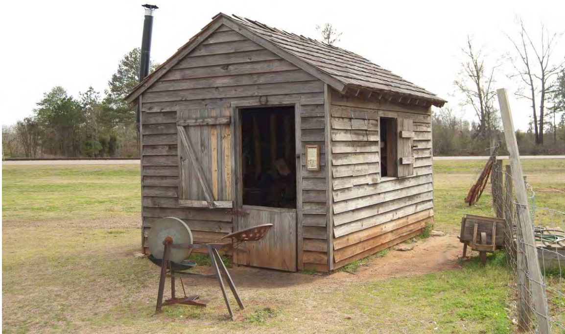
Photo BF-40: Blacksmith Shop (No LCS) Photo TJC
