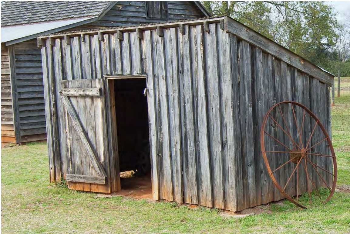
Photo BF-41: Pump Shed (No LCS) Photo TJC
