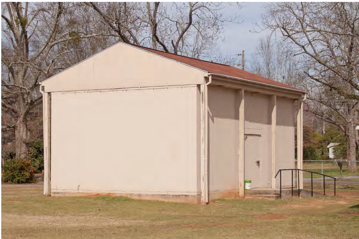
Photo PH-13: Bally Building (No LCS) Photo TJC
