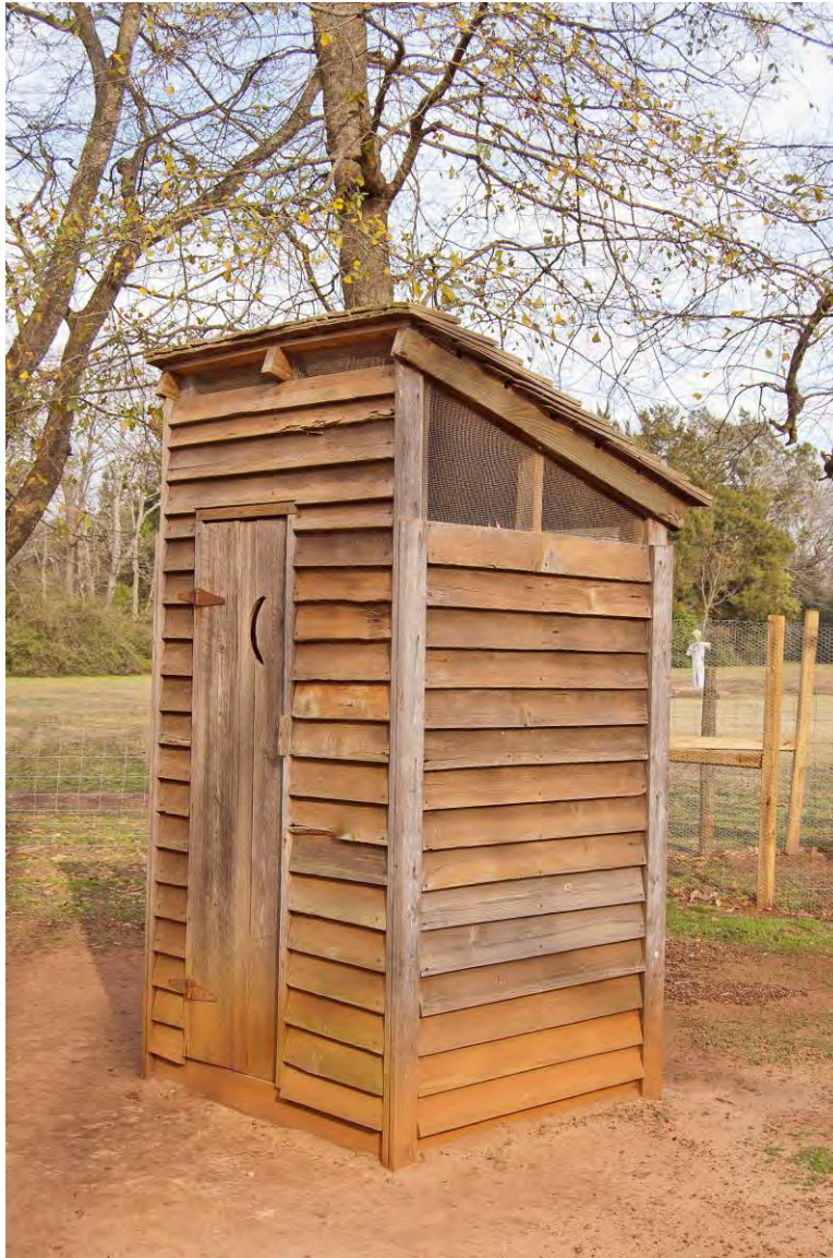
Photo BF-33: Privy (No LCS) Photo TJC
