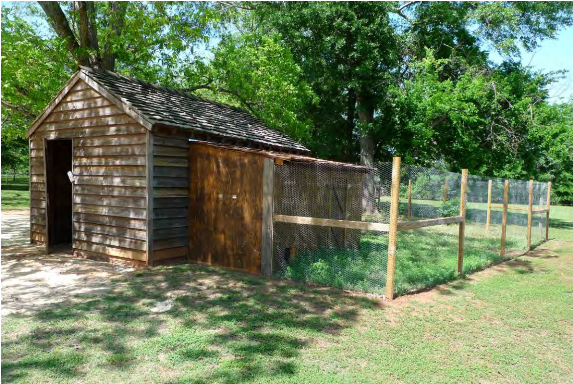
Photo BF-34: Chicken Coop/Smoke House (No LCS) Photo TJC
