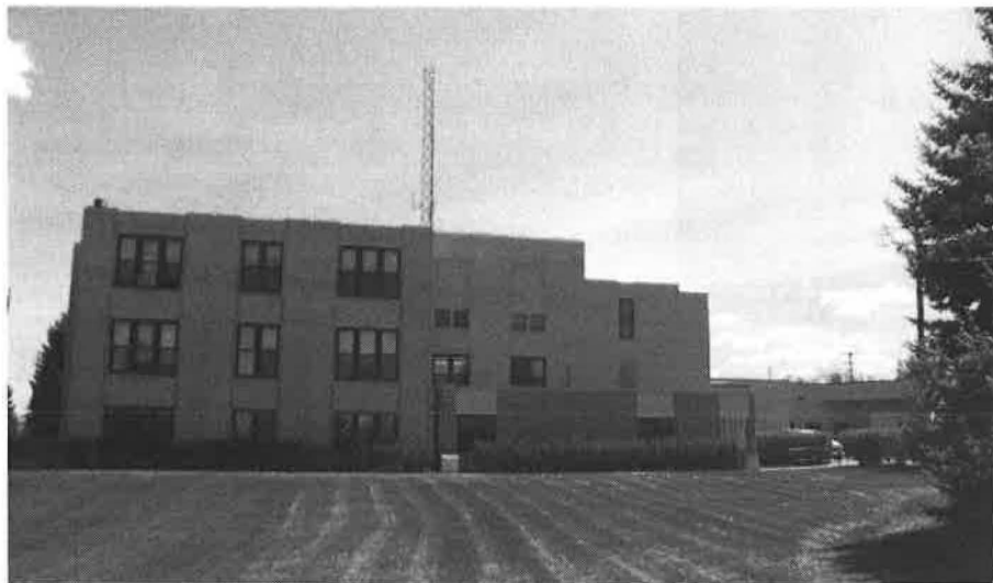
MT_GlacierCounty_GlacierCountyCourthouse_005 Glacier County Courthouse, west elevation, view to the east.
