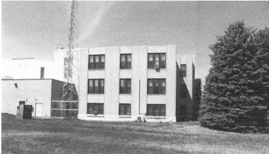
MT_GlacierCounty_GlacierCountyCourthouse_003 Glacier County Courthouse, east elevation, view to the west.
