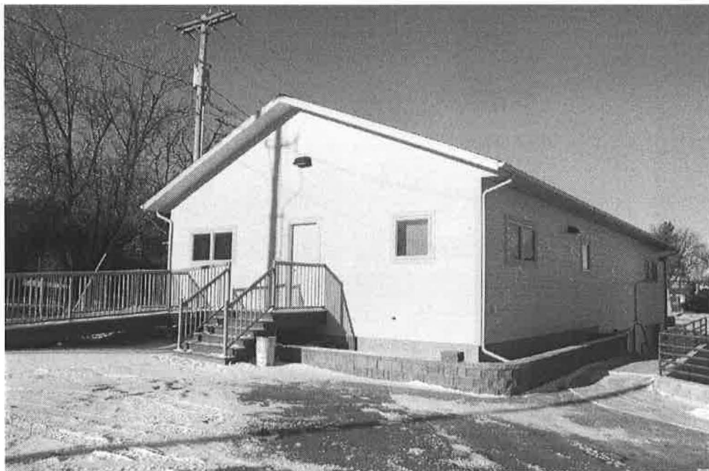
MT_GlacierCounty_GlacierCountyCourthouse_014 Sheriff's office, east and north elevations, view to the southwest.
