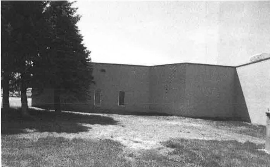
MT_GlacierCounty_GlacierCountyCourthouse_009 Glacier County Courthouse, east and north elevations of detention center addition, view to the south-southwest.
