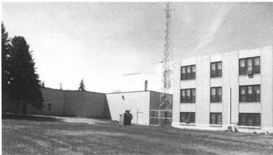
MT_GlacierCounty_GlacierCountyCourthouse_004 Glacier County Courthouse, east elevation and overview of detention center addition, view to the southwest.
