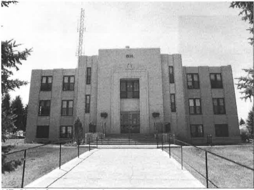
MT_GlacierCounty_GlacierCountyCourthouse_001 Glacier County Courthouse, north elevation, view to the south. MT_GlacierCounty_GlacierCountyCourthouse_001
