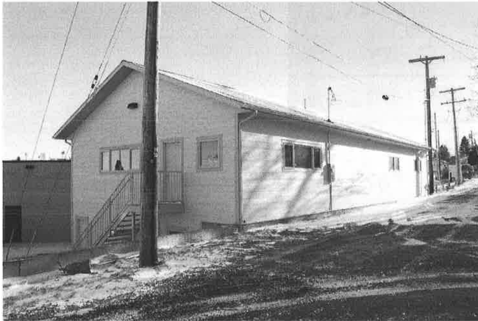
MT_GlacierCounty_GlacierCountyCourthouse_015 Sheriff's office, west and south elevations, view to the northeast.
