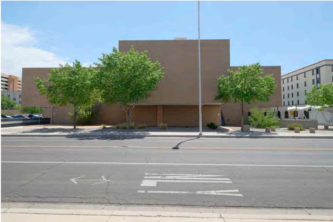
5. Rear (west) elevation with landscaping from 6 th Street, photographer facing east.
