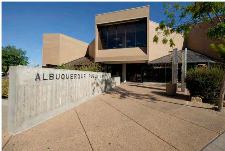
10. Main entrance with entrance sign, photographer facing northwest.
