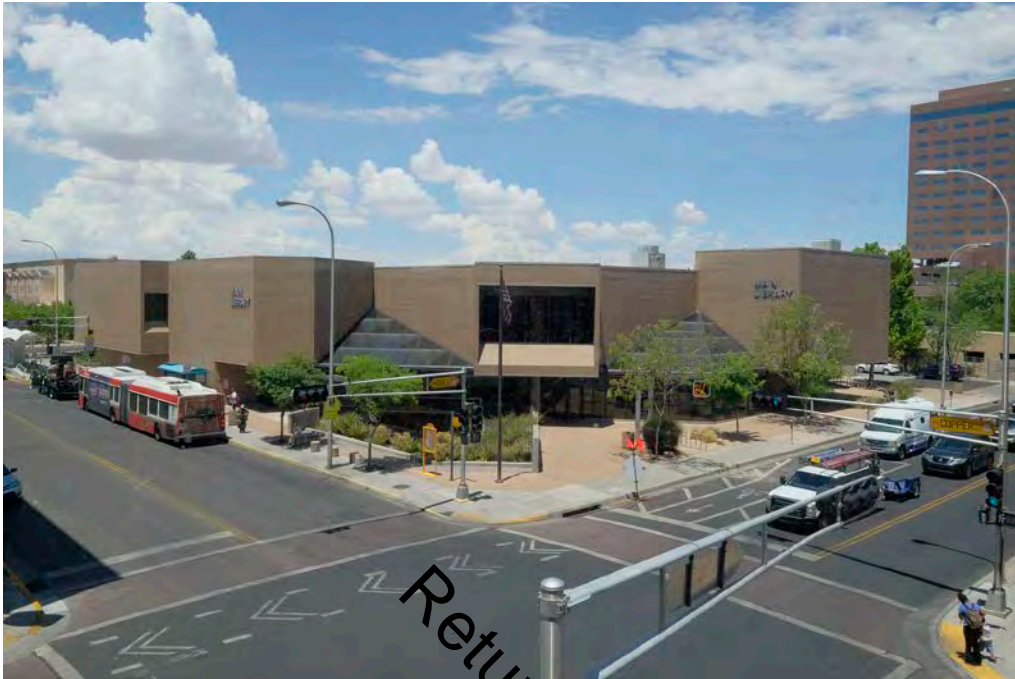
1. South and east sides, photographer facing northwest.
