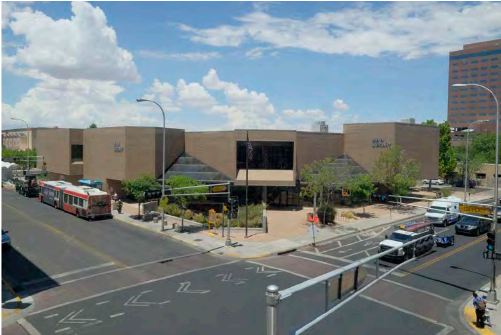
1. South and east sides, photographer facing northwest.
