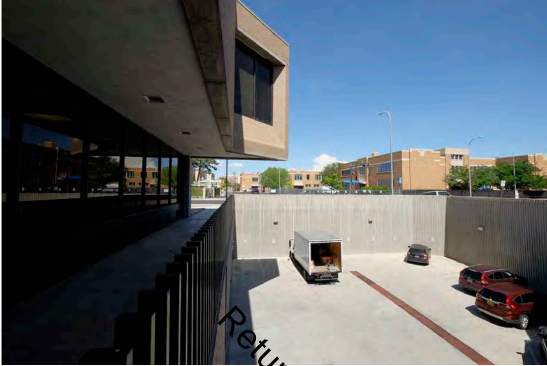
31. Lower level, northwest service court, photographer facing west.
