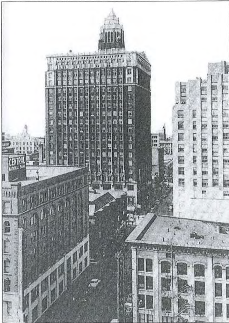
Figure 4: The Equitable Building, looking southwest; ca. 1931 (Long 1988, 49)
