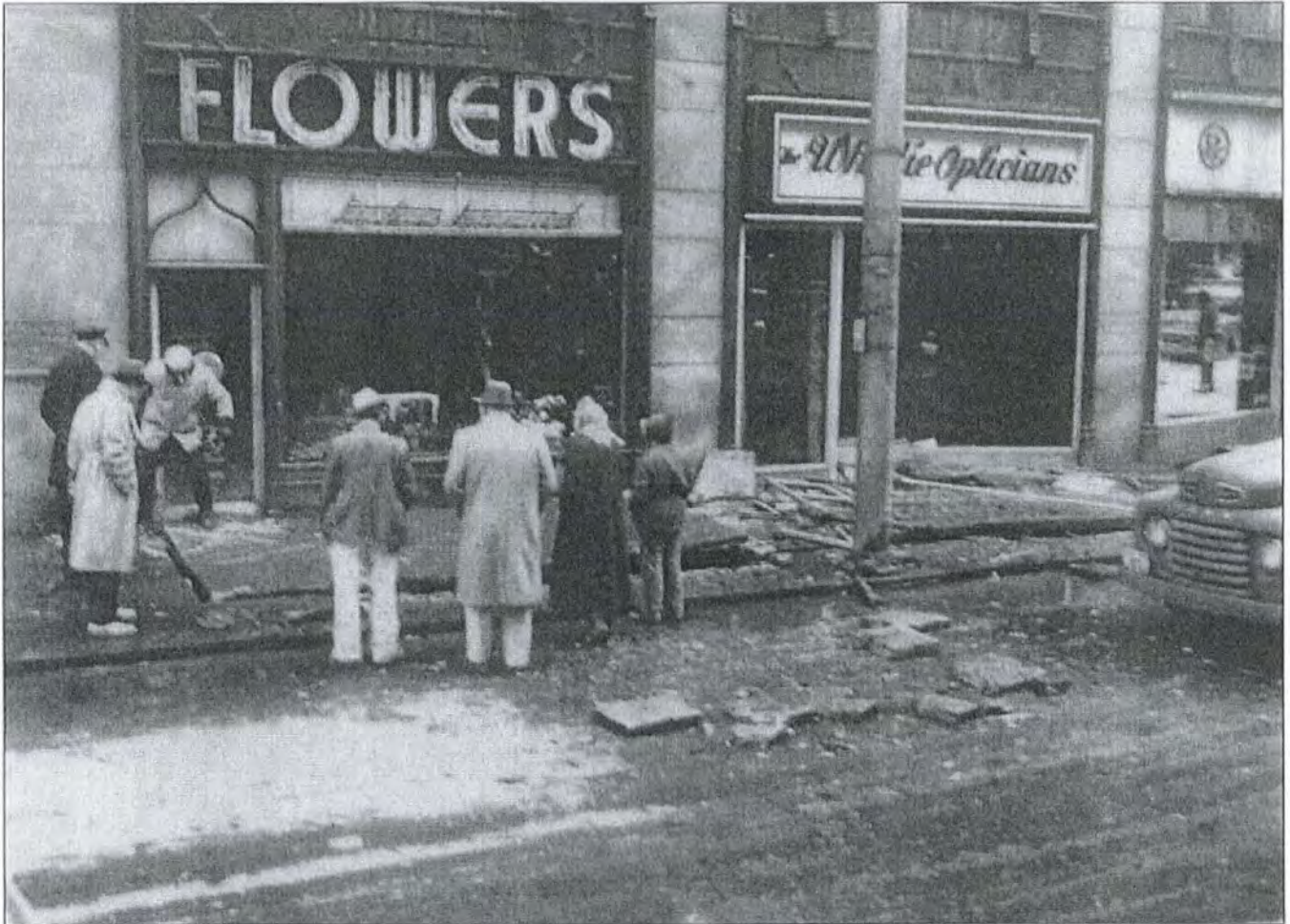
Figure 6: 1950s explosion at the Equitable Building shattered several Locust Street storefront's plate glass panels. The 'Flowers' storefront shows original materials, including a bulkhead, a door transom with ogee-shaped arch, and rectangular-shaped transoms above the storefront window. The 'Wylie Opticians' storefront already had been remodeled (unidentified newspaper clipping in offices of Ruhl & Ruhl Realty Company, Des Moines, IA)
