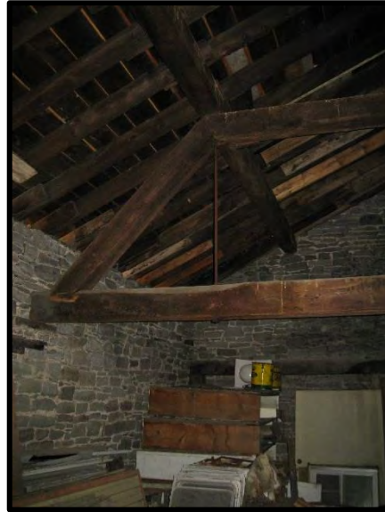
Figure 7. Truss system supporting roof.
