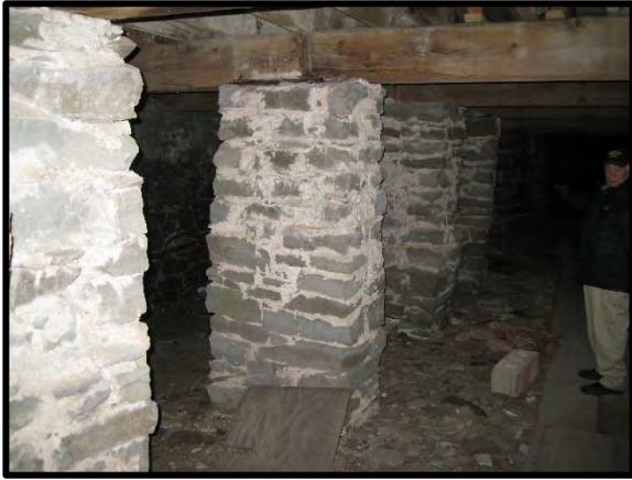
Figure 6. Basement piers; some of the supporting beams show circular saw marks.
