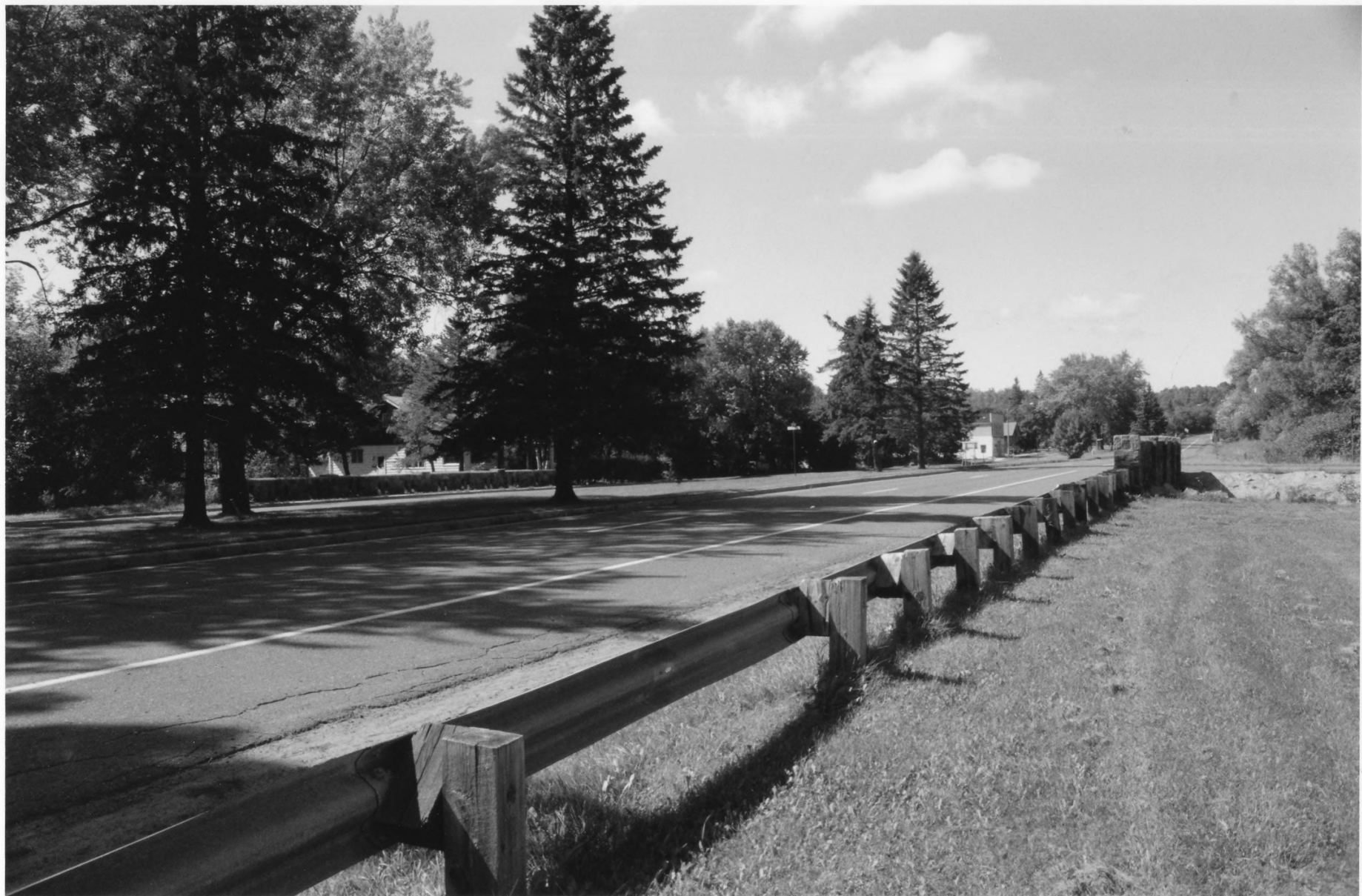
Bridge no. 5757 Mn Hwy. 23 over Mission Creek, Duluth St. Louis Co., Mn 013072-8
