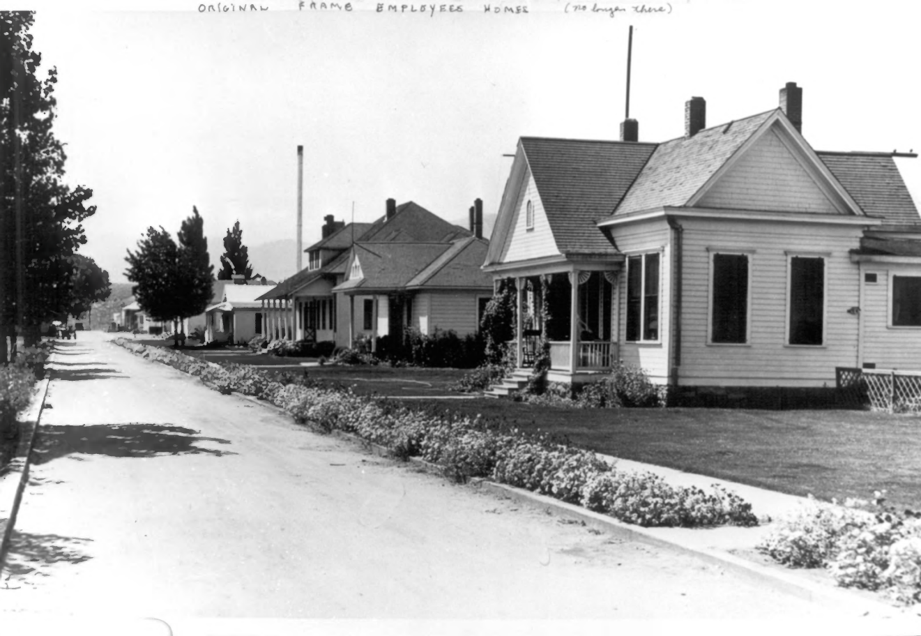
ORIGINAL FRAME EMPLOYEE HOME (no longer there)
