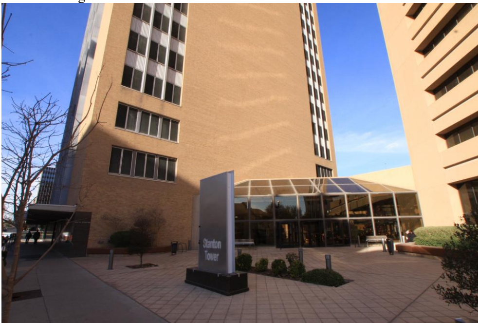
Photo 15 South elevation with hyphen Camera facing north
