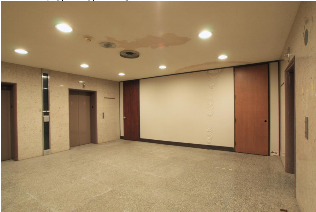
Photo 22 Fourth Floor, Typical Upper Lobby without Glass
