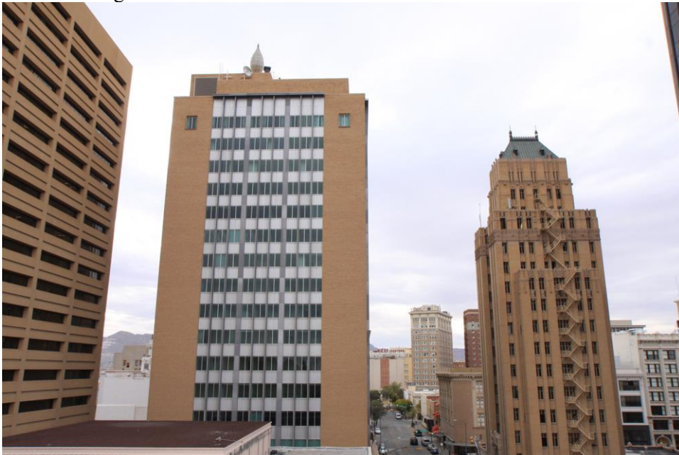
Photo 3 East Façade Camera facing west
