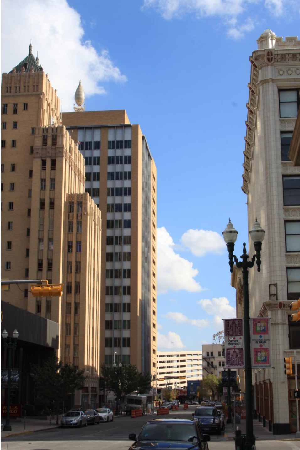
Photo 1 North Side, from Stanton Street Camera facing south
