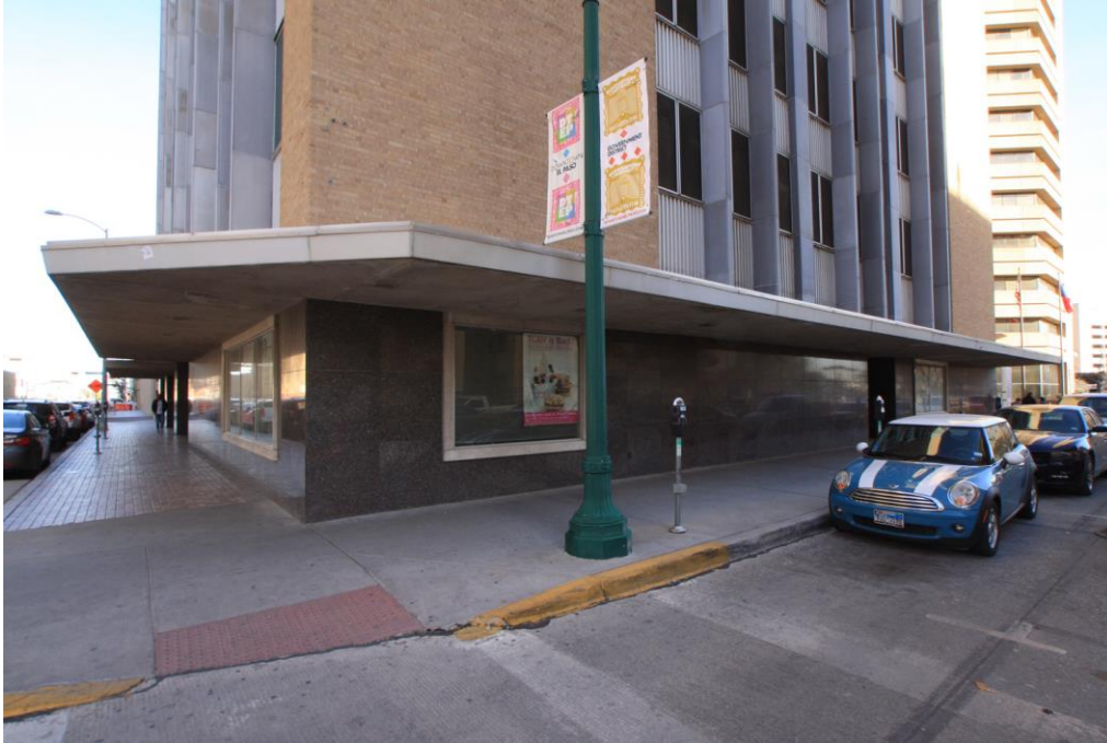
Photo 12 Ground floor at northwest corner Camera facing southeast
