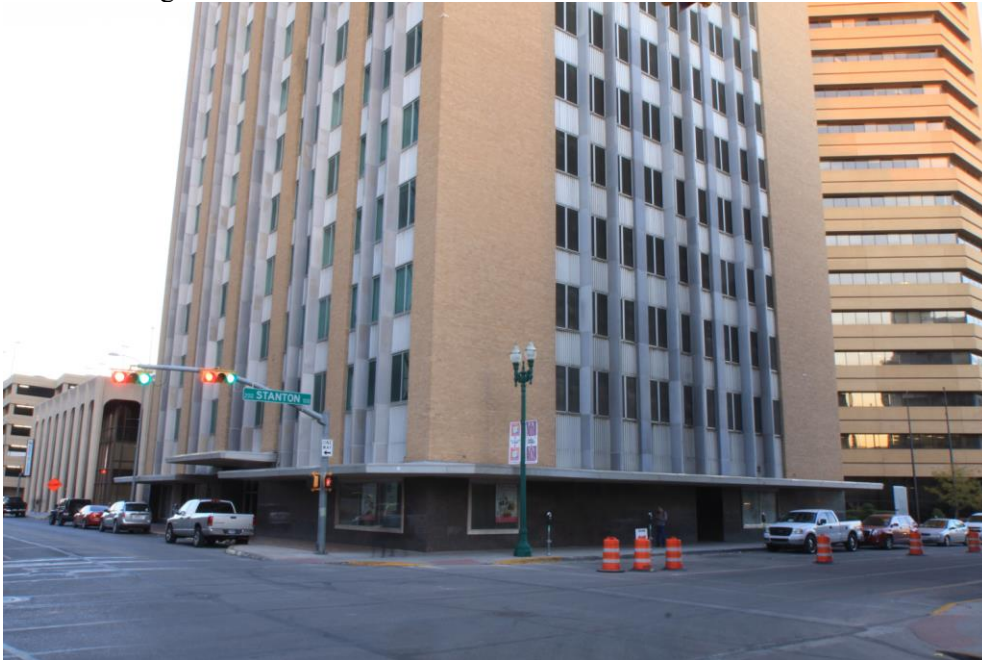
Photo 4 Northwest Corner Camera facing southeast
