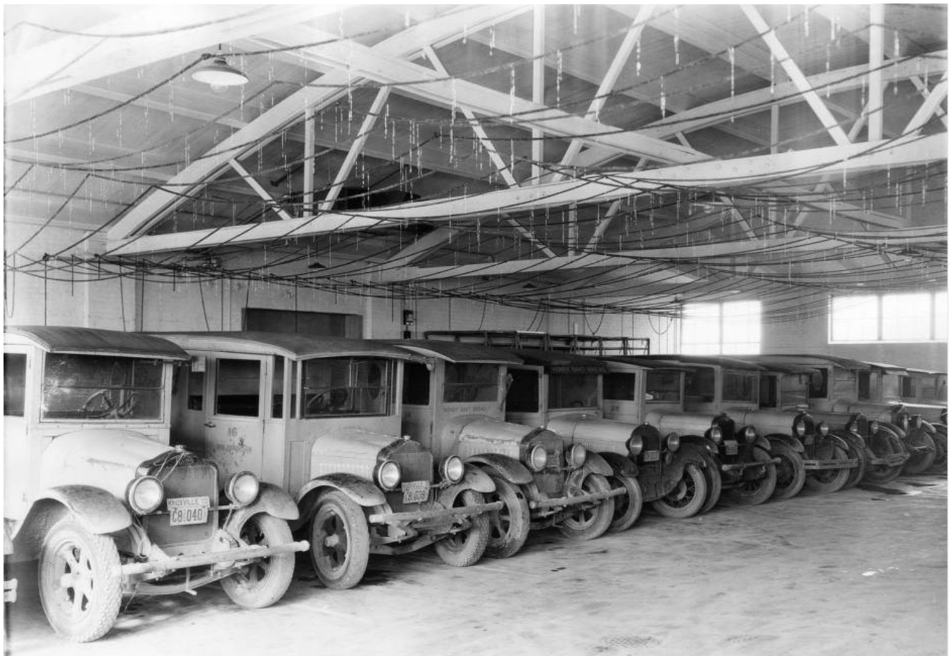
Figure 3. Undated photo of garage interior showing bowstring trusses and delivery trucks, collection of the author
