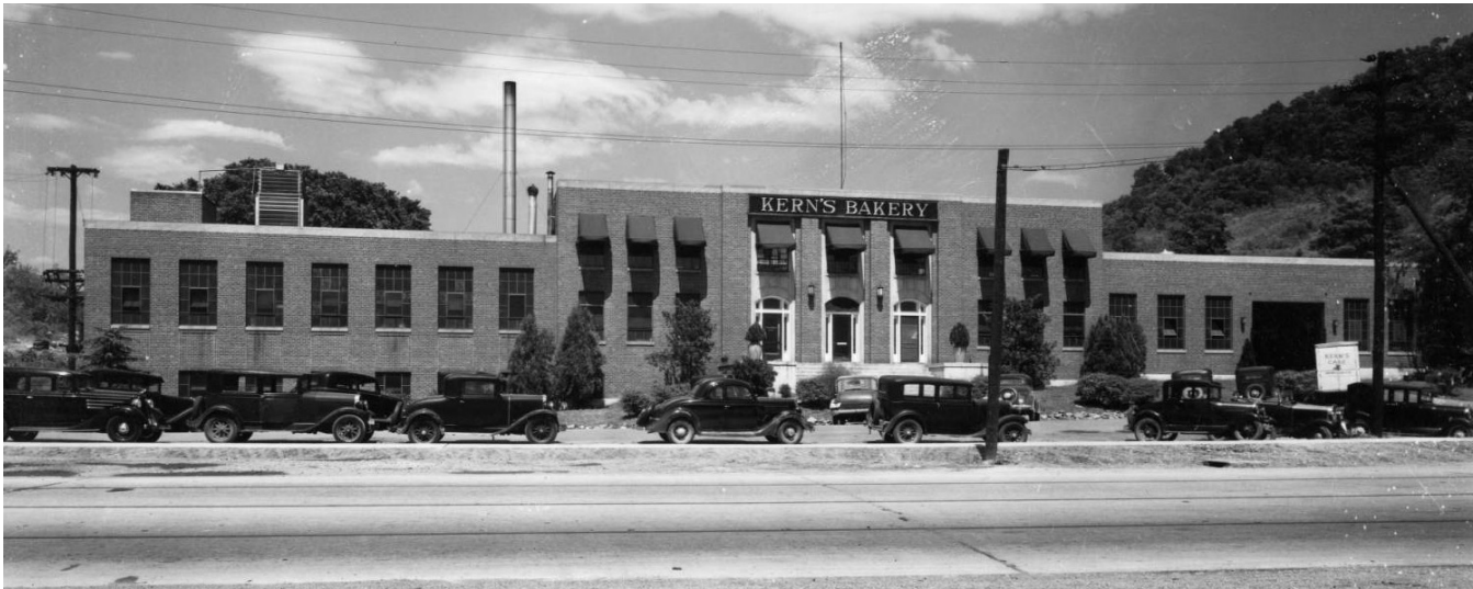
Figure 4. Photo c.1936 of Kern's from West, collection of the author
