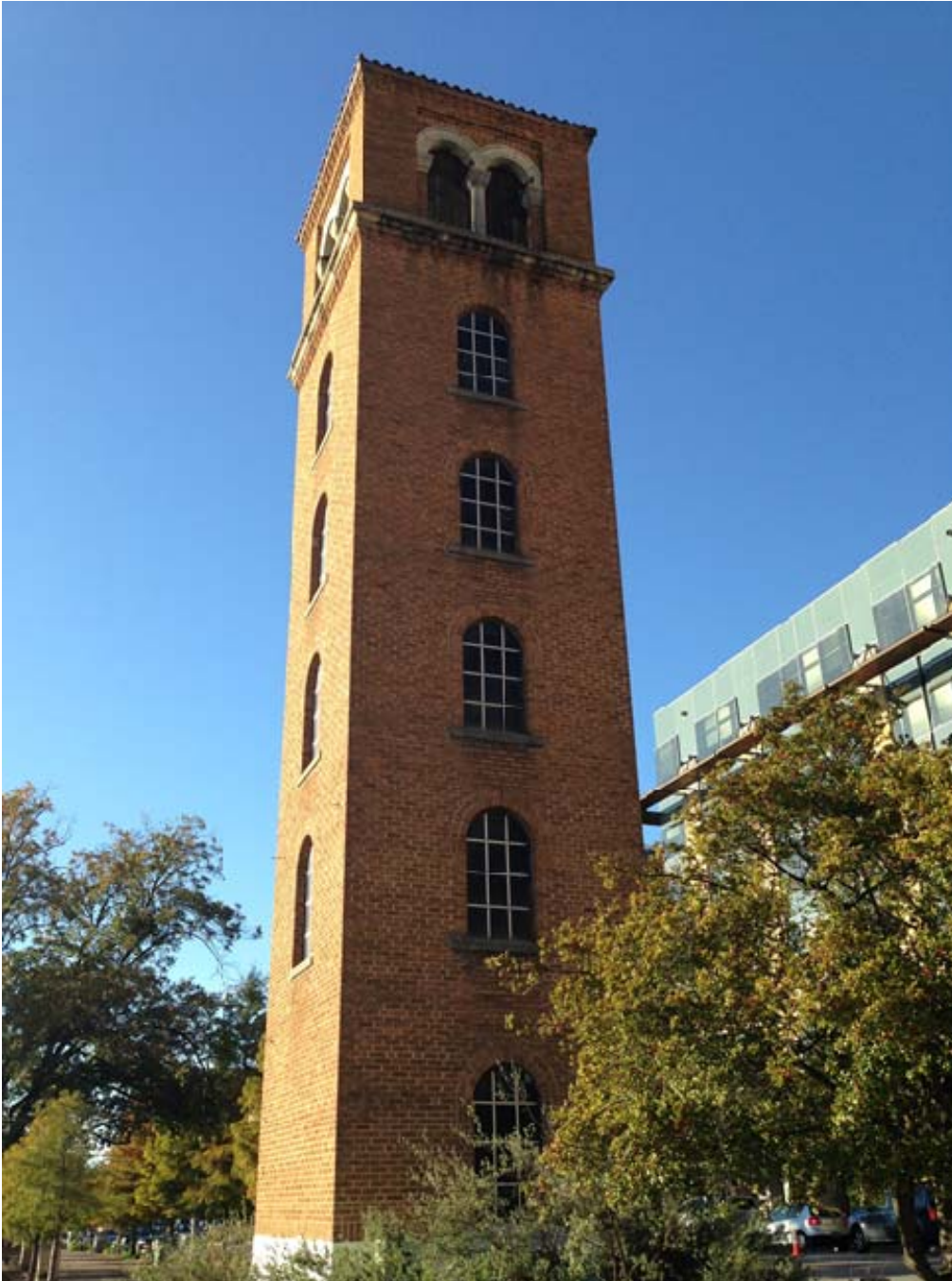
Photo 4: East façade. Camera facing west.
