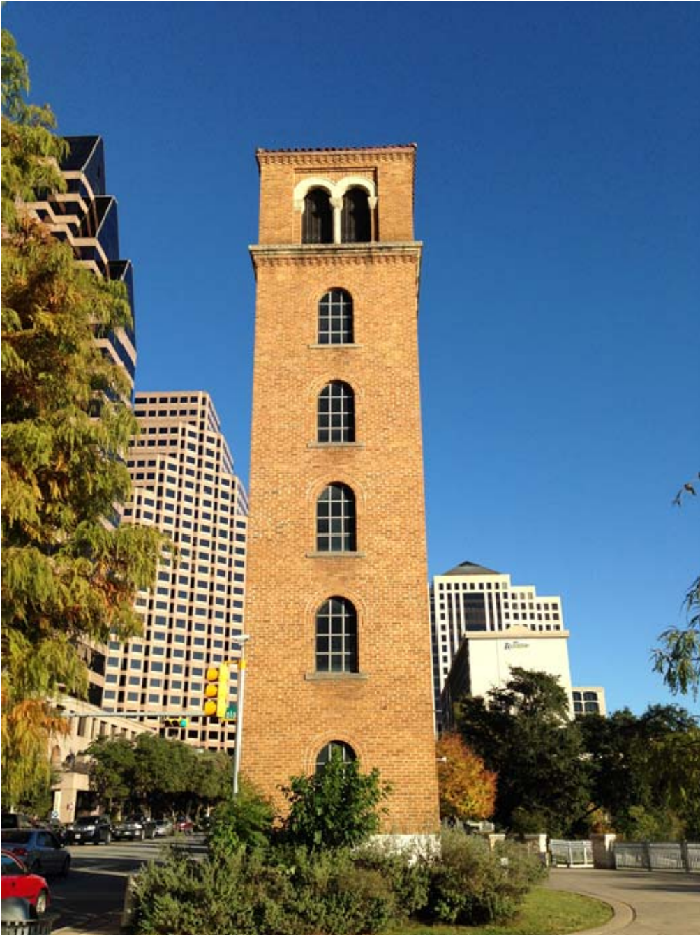
Photo 2: West façade. Camera facing east.
