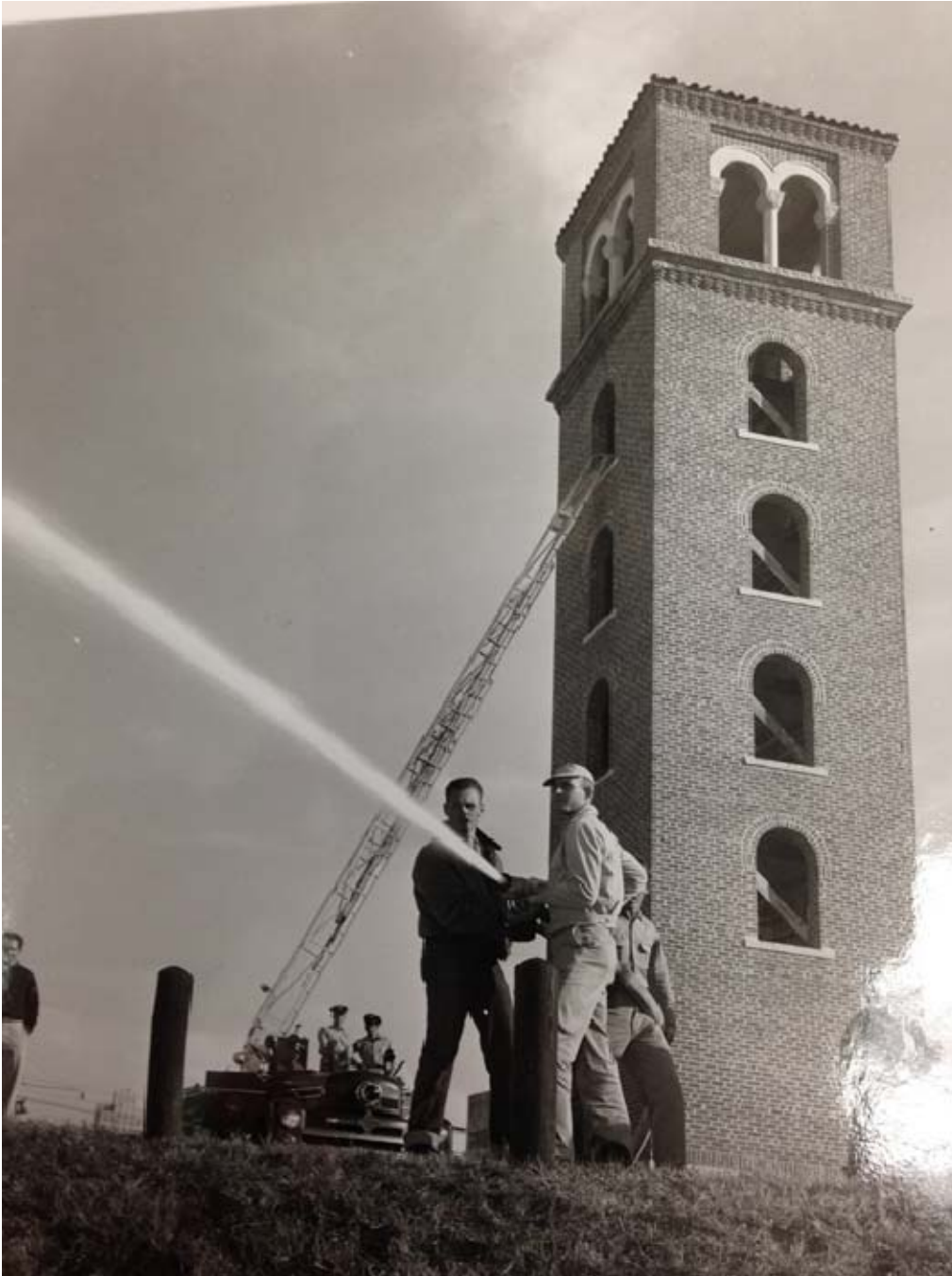
Figure 10: Testing the Hose (1954). Courtesy Austin Fire Museum.
