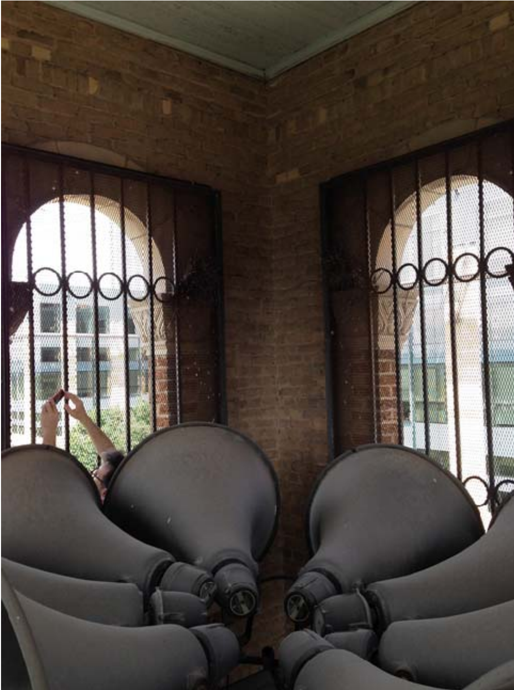
Photo 7: Sixth floor interior and carillon. Camera facing northwest.
