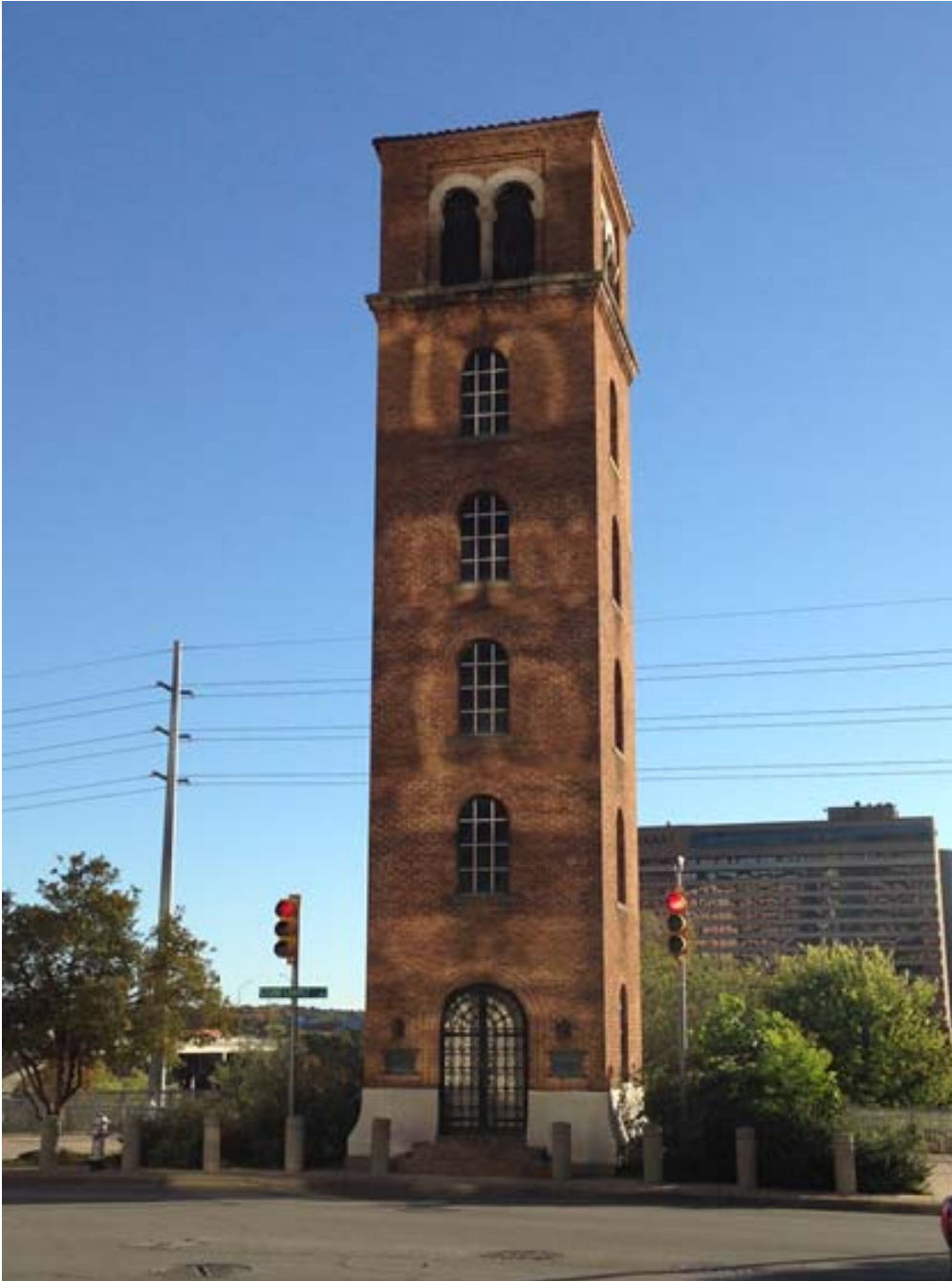
Photo 1: North façade. Camera facing south.
