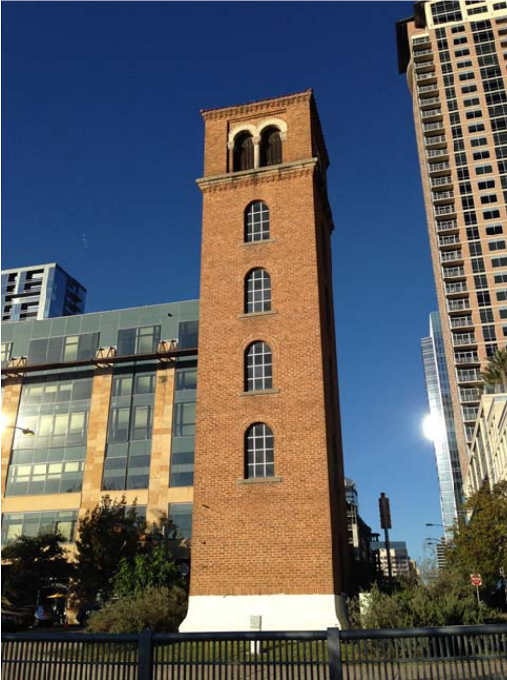
Photo 3: South façade. Camera facing north.
