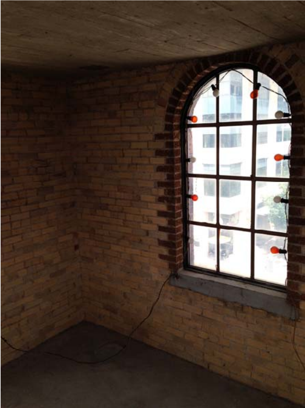
Photo 9: Third floor window. Camera facing northwest.
