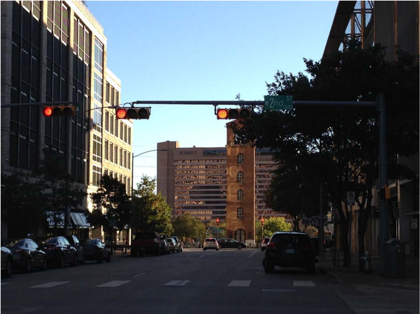
Photo 10: The north face of the tower, as seen from Colorado and 2 nd streets. Camera facing south, toward Lady Bird Lake.
