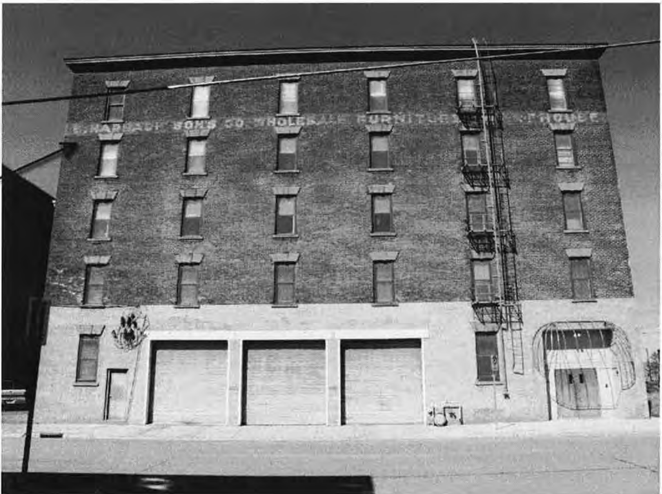
Figure 14: Warehouse, 300 SW Fifth Street, 2009
