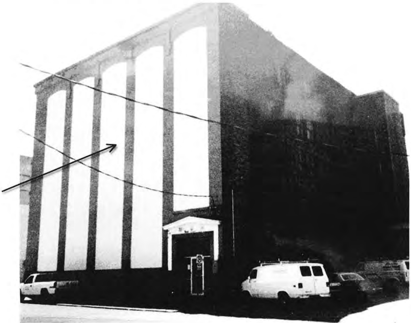
Figure 12: Factory building, 316 SW Fifth Street, circa 1992
