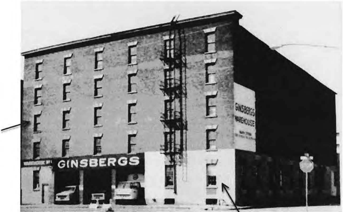
Figure 13: Warehouse, 300 SW Fifth Street, 1983
