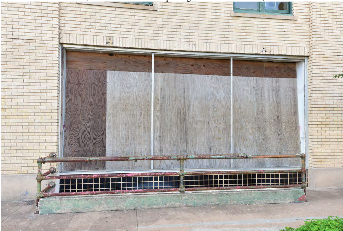
Photo 8. East elevation, detail of storefront opening and basement stair, view west.
