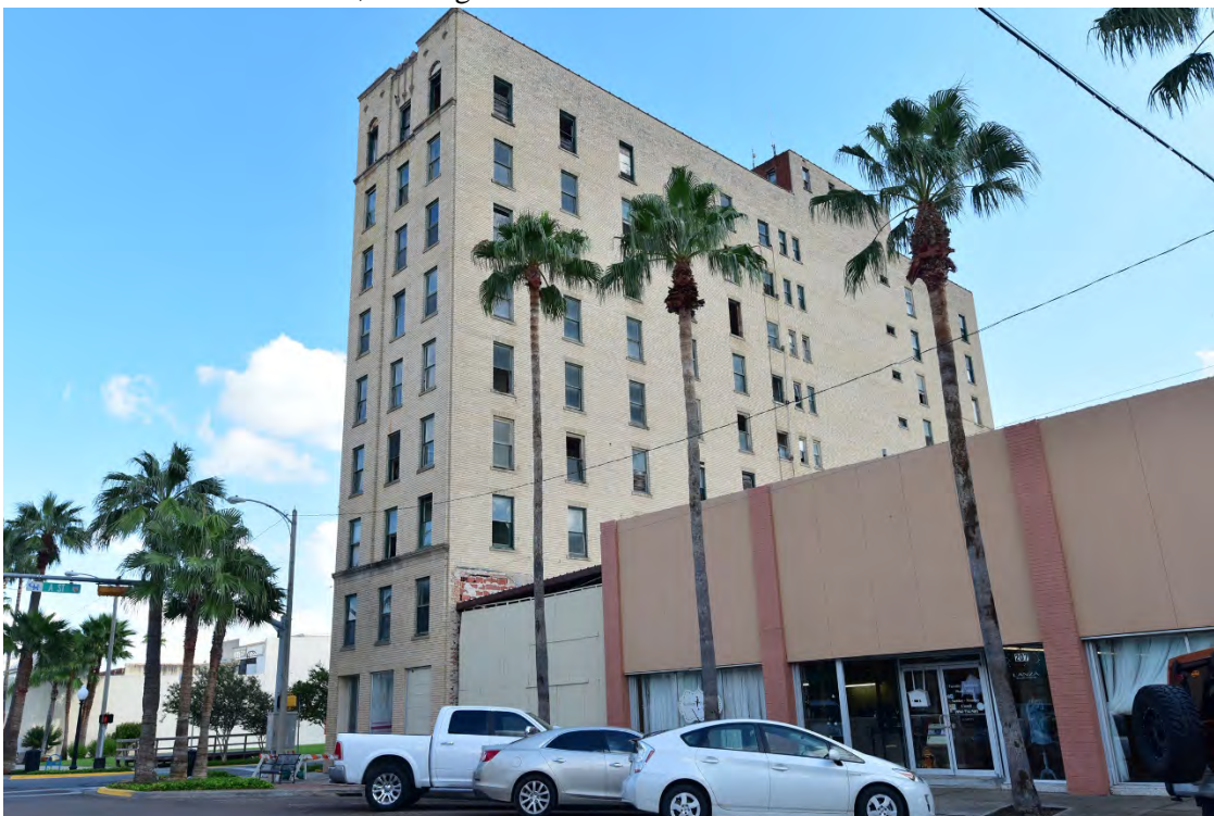
Photo 10—Jackson Avenue, looking northeast.
