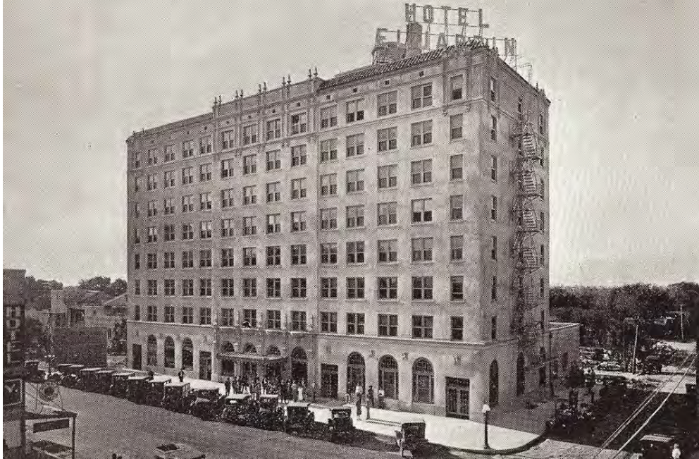
Figure 16. Historic photograph of El Jardine Hotel in Brownsville, just after completion. Source: Bronsbil Estacion blogpost, May 16, 2015. http://bronsbilestacion.blogspot.com/2015/05/el-jardin-gets-buyer-brownsville-herald.html .
