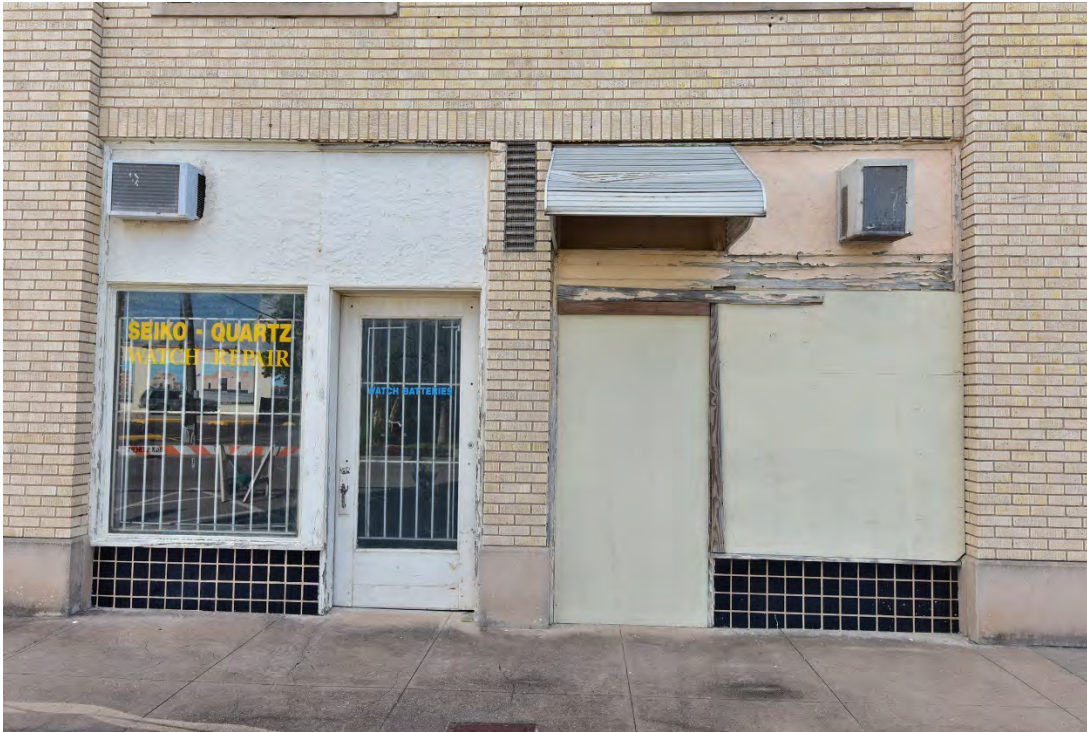
Photo 7. East elevation, view west showing first floor store openings.
