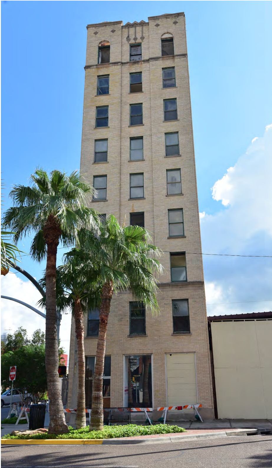
Photo 2—North elevation, view south.
