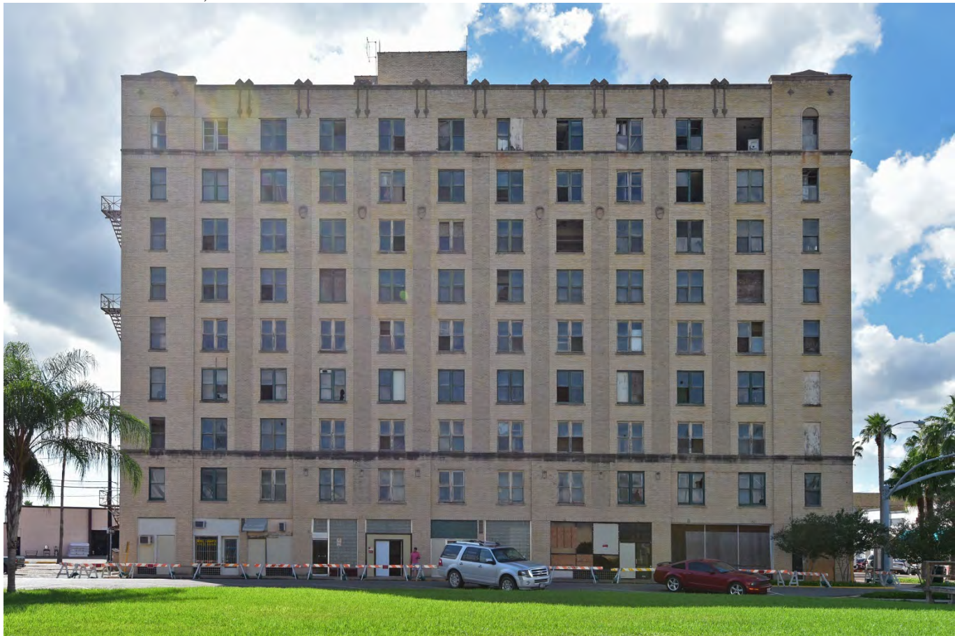
Photo 1—East elevation, view west.
