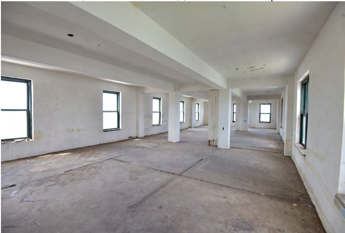
Photo 16—Sixth floor, view northwest. Floors 6,7, and 9 have no historic partitions.
