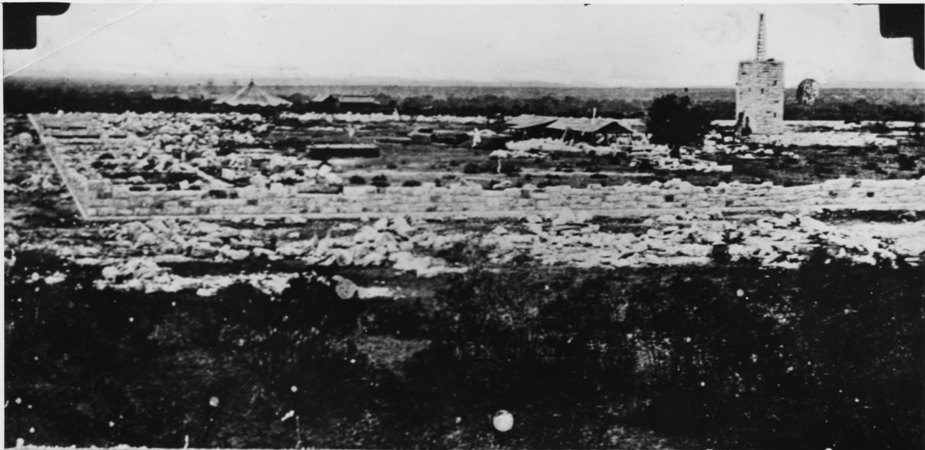
No. 3 1/2 - Commencement above foundation, looking N. W. Aug. 31. 76.
