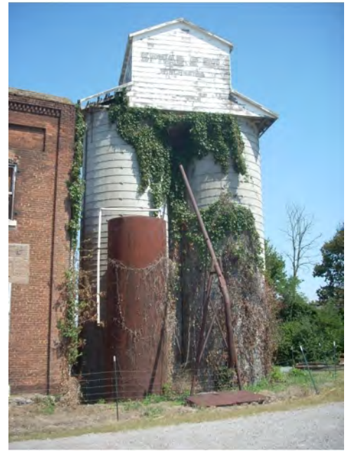
Photo 2: silos at east (rear) end of building
