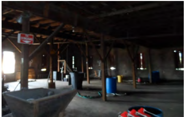
Typical Roof Framing-Post and Beam
