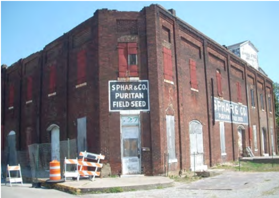
Photo 3, southwest corner entry building
