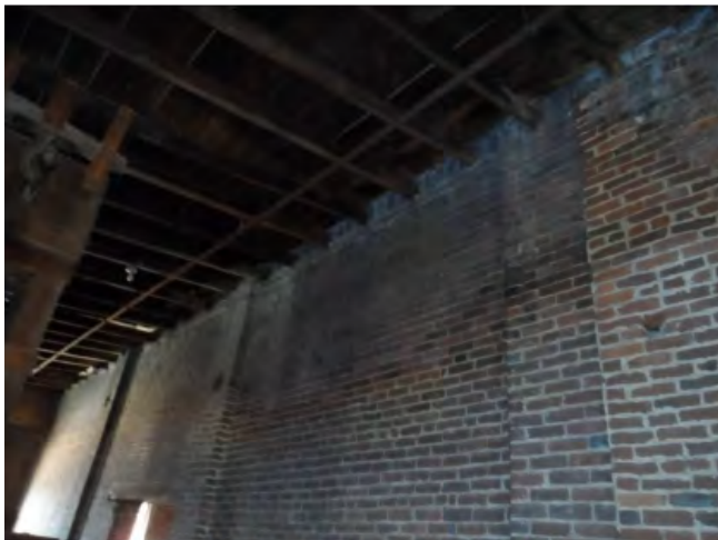
Typical Rafter Bearing on Exterior Walls
