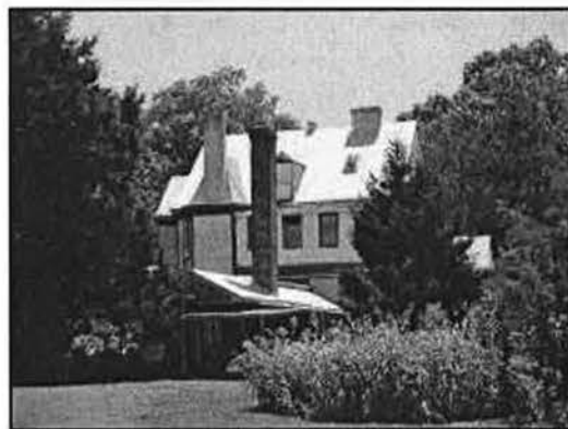
Remnants of Nickel's greenhouse at the back of 3001 Condie Street
