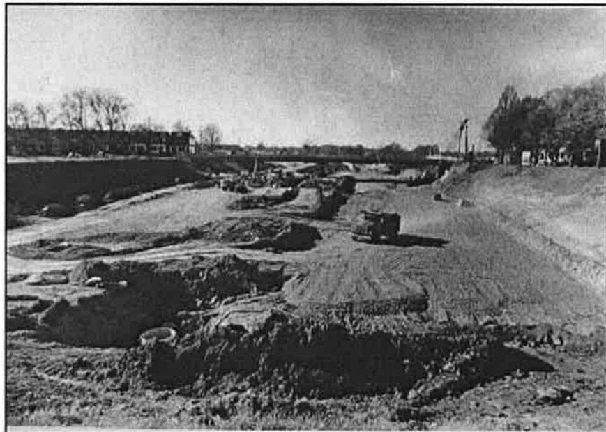
14. Construction of the Downtown Expressway, Looking West. Houses on the 500 block of S. Sheppard Street are visible in the left background and the Sheppard Street Bridge is at the center background. Source: The Valentine.
