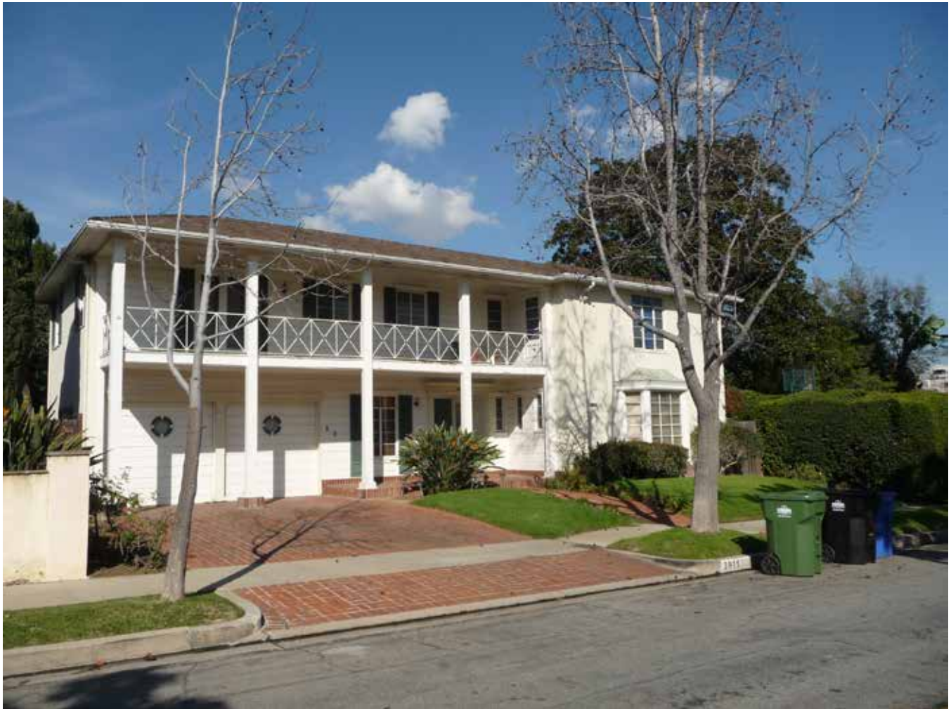
CA_Los Angeles County_View Park Historic District_21.TIF 3911 Olympiad Drive, Monterey Revival residence, facing northwest
