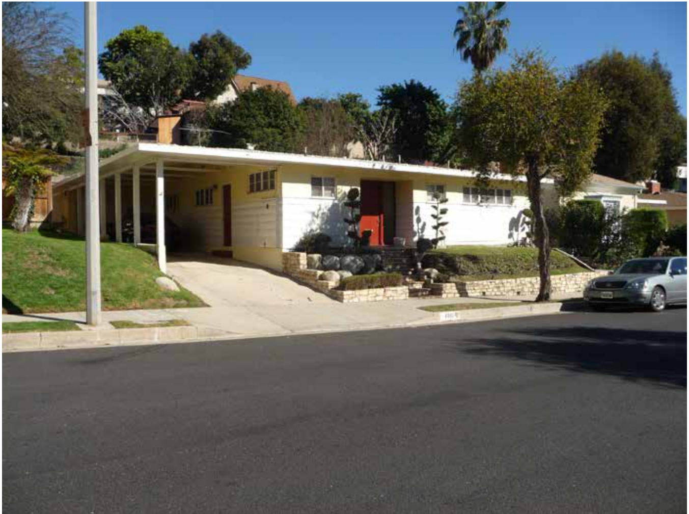
CA_Los Angeles County_View Park Historic District_32.TIF 4510 S Mullen Avenue, Contemporary Ranch residence, facing northeast
