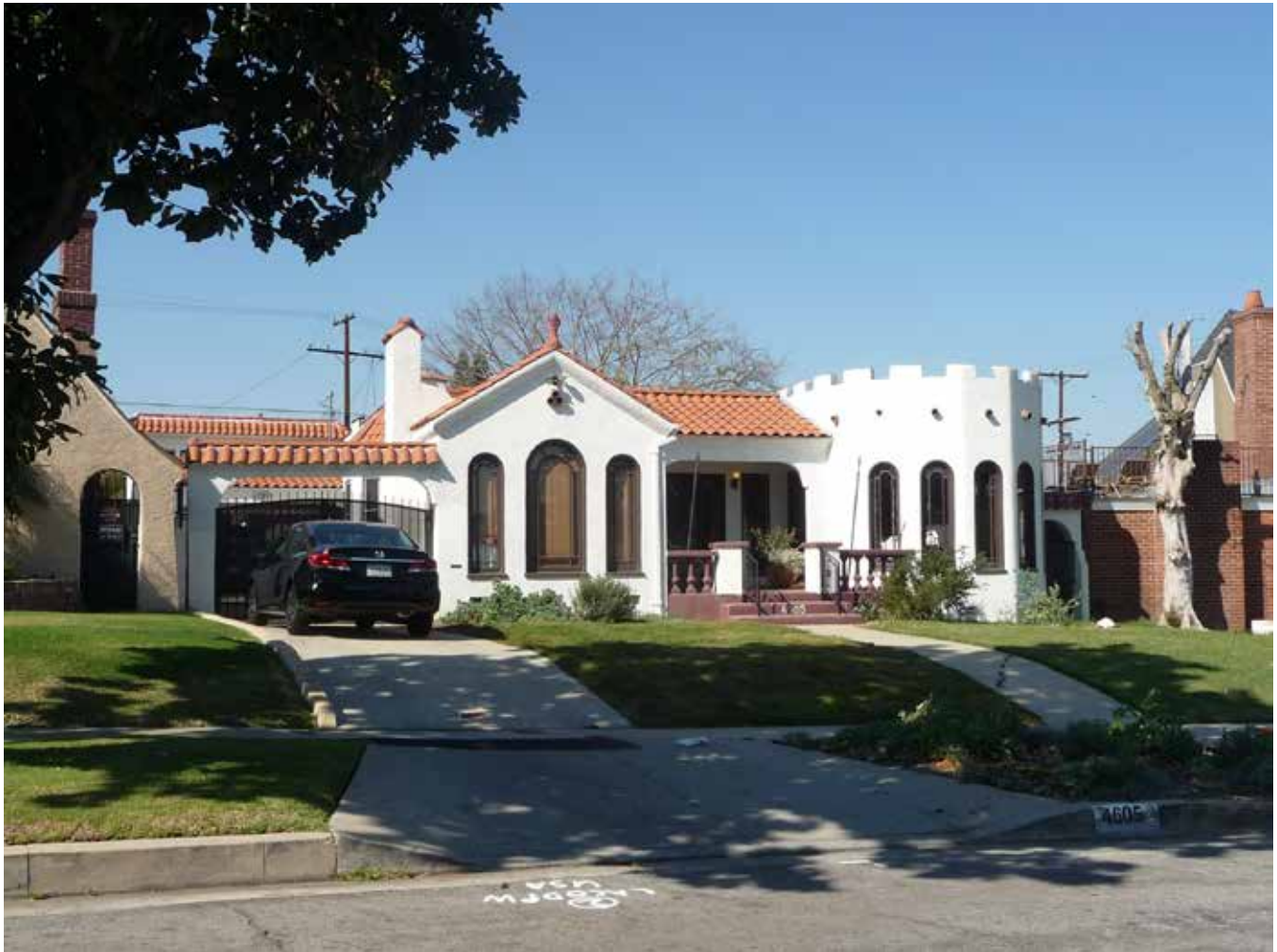
CA_Los Angeles County_View Park Historic District_14.TIF 4605 Brynhurst Avenue, Spanish Colonial Revival residence, facing northwest
