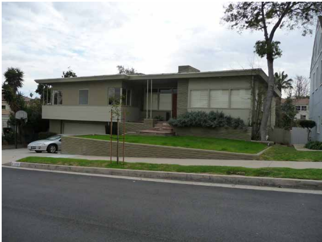
CA_Los Angeles County_View Park Historic District_27.TIF 3766 Monteith Drive, Contemporary Ranch residence, facing southwest
