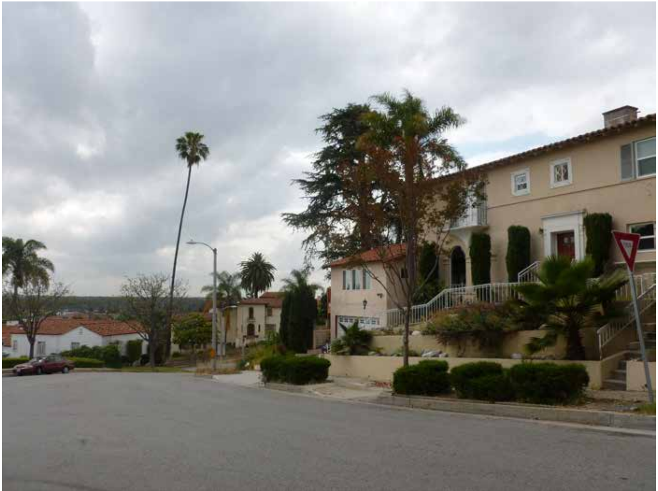
CA_Los Angeles County_View Park Historic District_05.TIF Aureola Boulevard and Palmero Boulevard, streetscape, facing southeast
