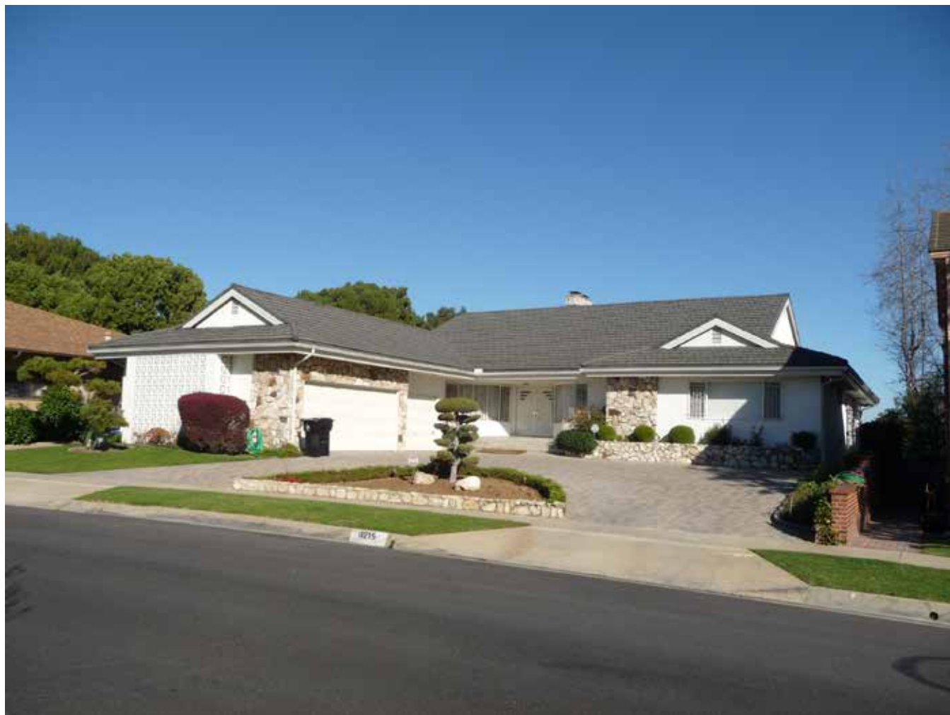
CA_Los Angeles County_View Park Historic District_23.TIF 4215 Enoro Drive, Oriental Ranch residence, facing east
