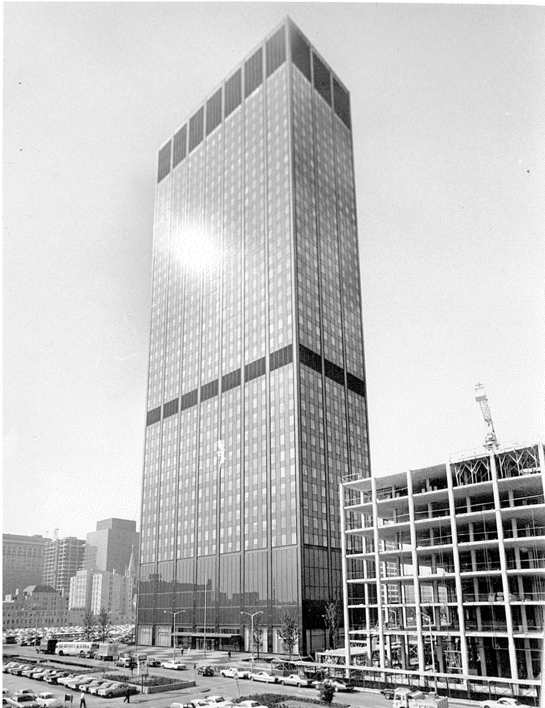
FIGURE 22 – Erievew Tower, East 12 th Street elevation with adjacent new construction, August 19, 1968, looking southwest; Photo CPL002394, Cleveland Public Library Photograph Collection.
