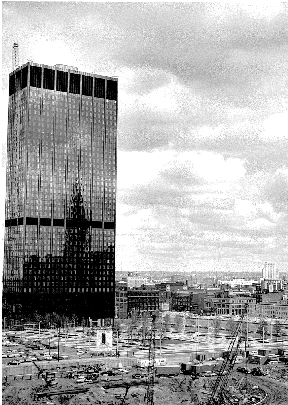
FIGURE 15 – Erievew Tower construction with federal building construction in foreground and existing buildings in background, November 6, 1964, view looking southeast; Photo 370, Cleveland Public Library Photograph Collection.
