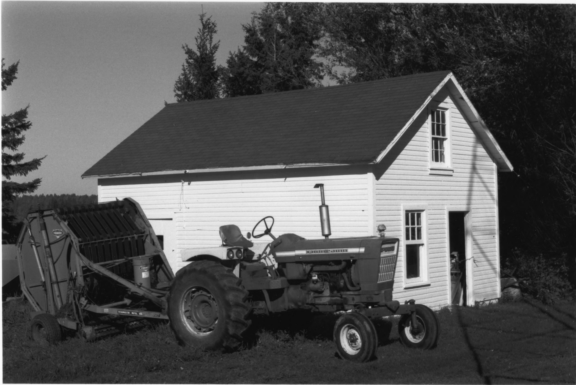
Warehouse, Flint Creek Farm Historic District St. Louis County, MN 09338 / 5
