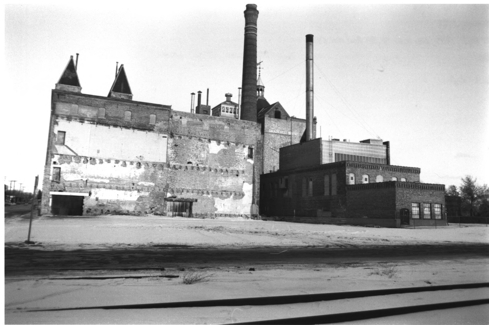
Rear of Brew House and Power Station, Minneapolis Brewing Company Historic District Hennepin County, MN
