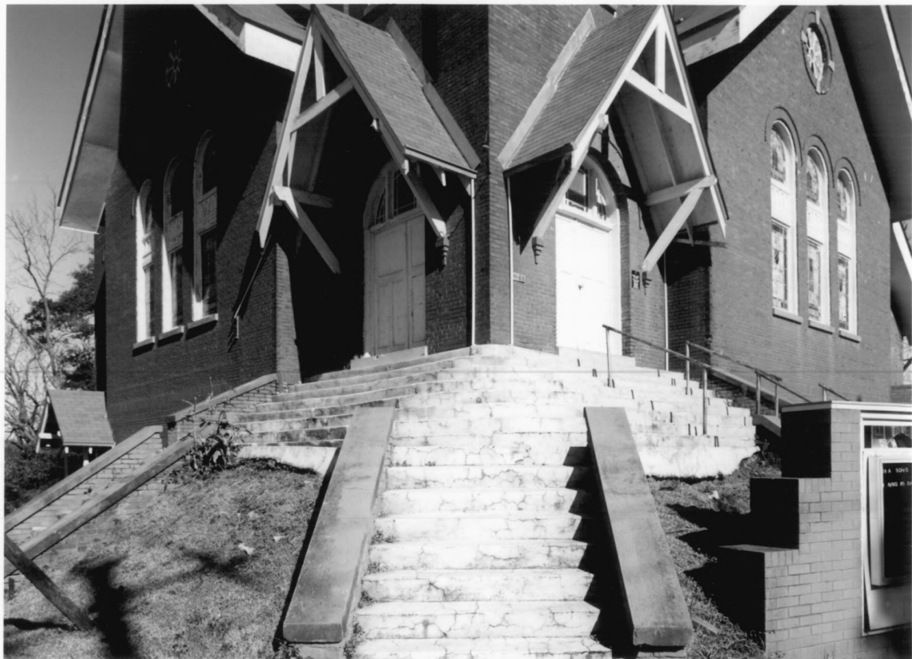
Campbell Chapel AME Church, Sumter County, Georgia 3 of 10
