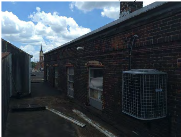
View from the adjacent roof, facing south
