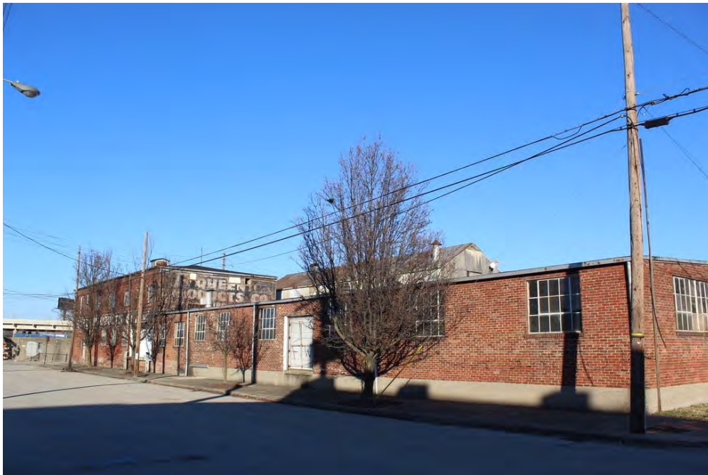
19 of 19: The side façade along North 13 th Street, facing north.
