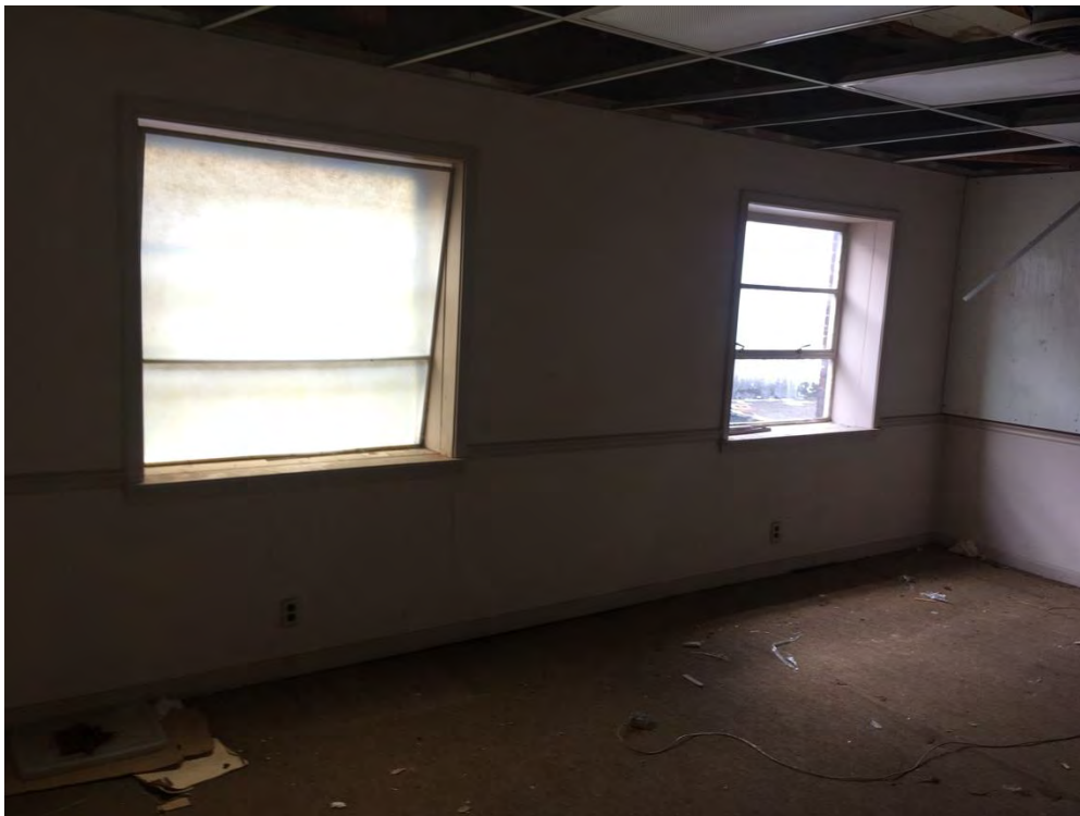
13 of 19: Rear office space on the second floor, facing southeast.
