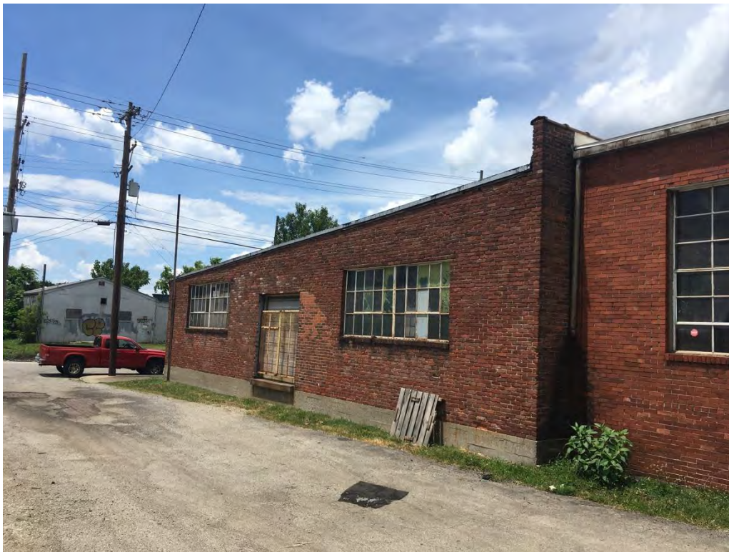
3 of 19: The rear façade, facing west toward 13 th Street.
