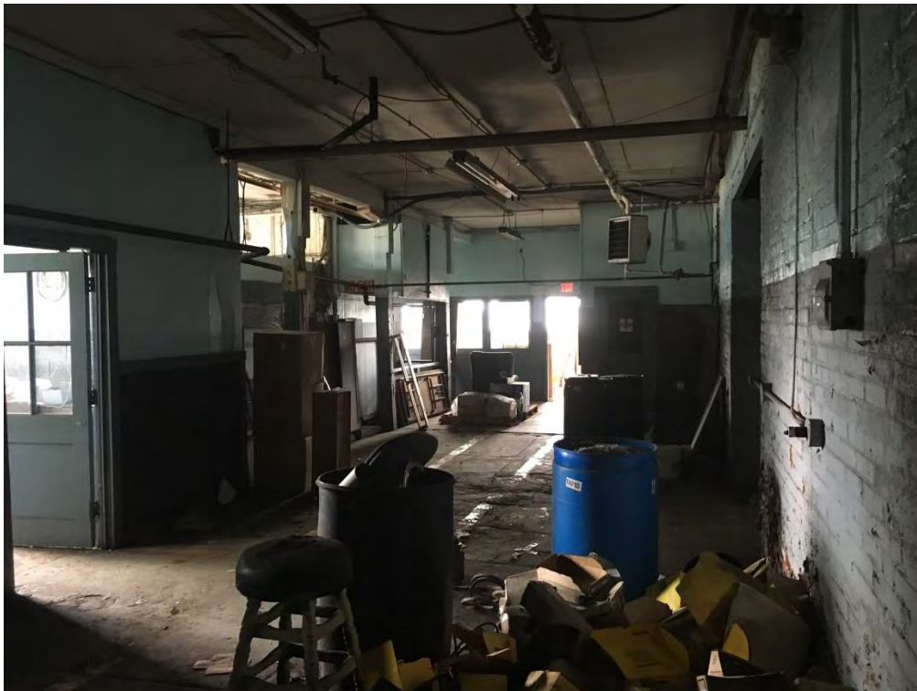
5 of 19: Warehouse space on the first floor, facing north, in the west portion of the building.
