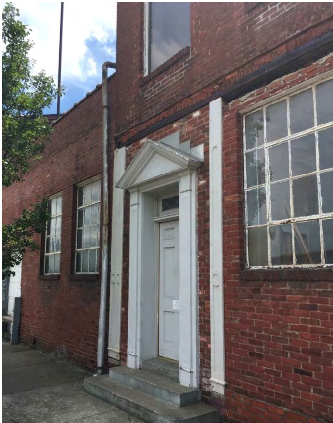
Existing front door with pilasters and pediment
