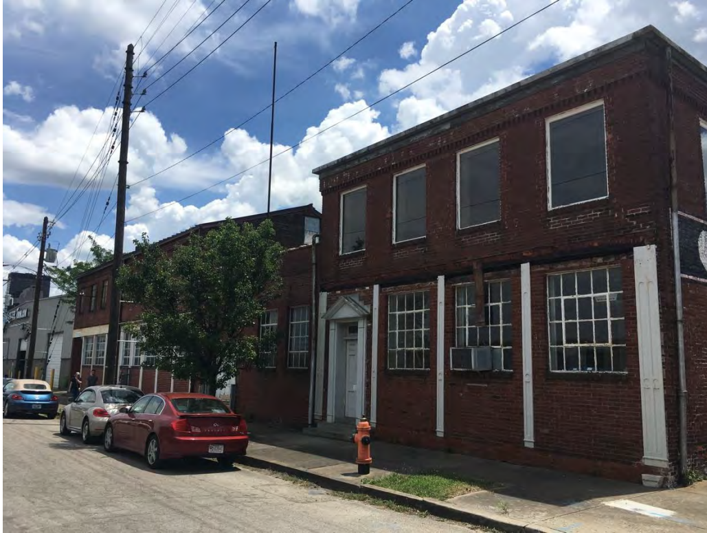
2 of 19: The front façade from Rowan Street.
