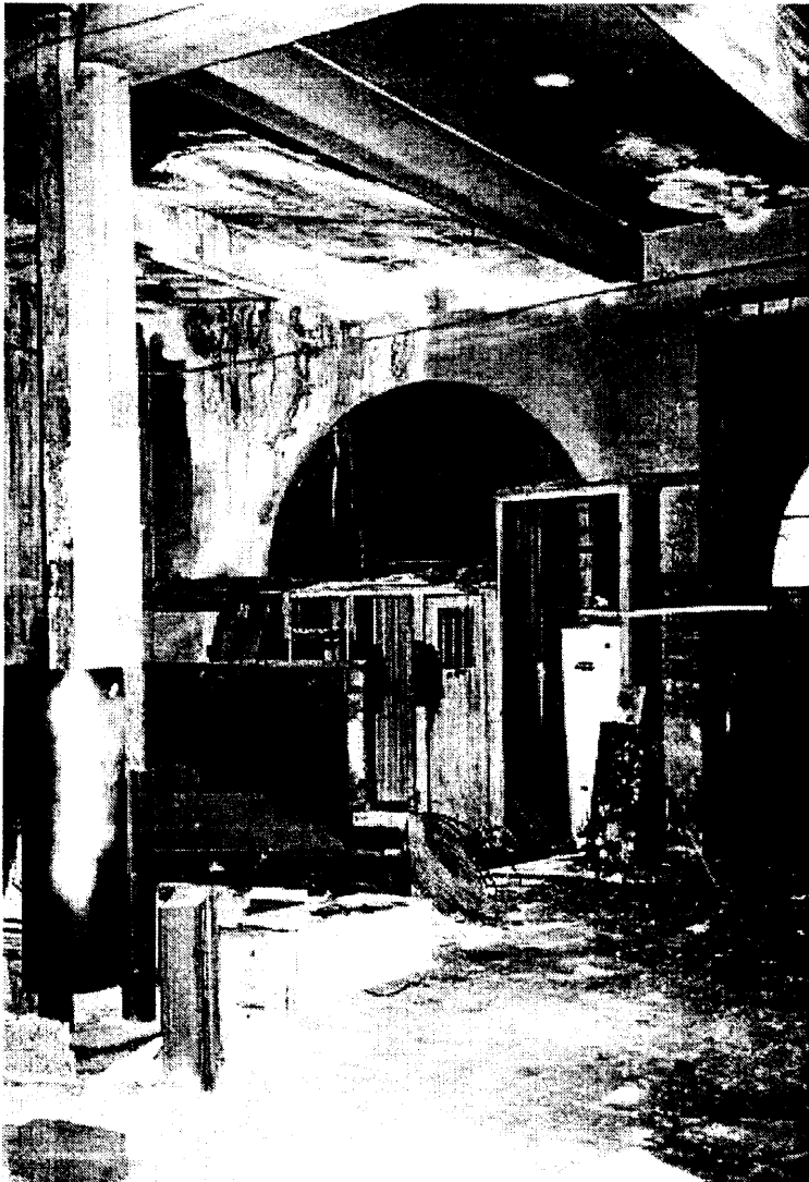
Photo 45: Storage room, facing northwest.
