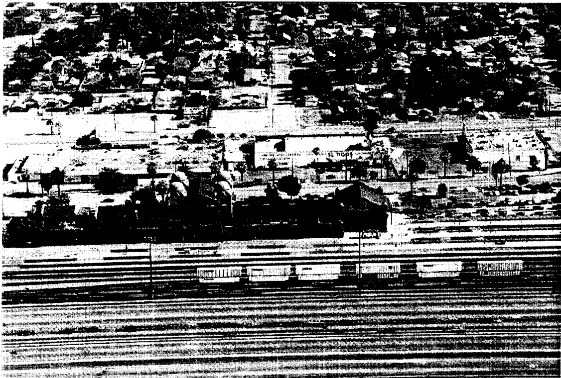
Photo 1: Aerial of north facade (track side) showing the contextual setting, facing south.
