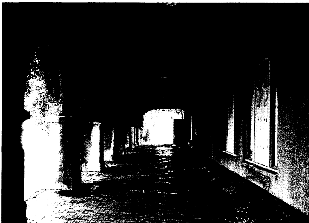
Photo 22: View through the covered arcade along the north facade, facing east. Note the boarded arched windows.
