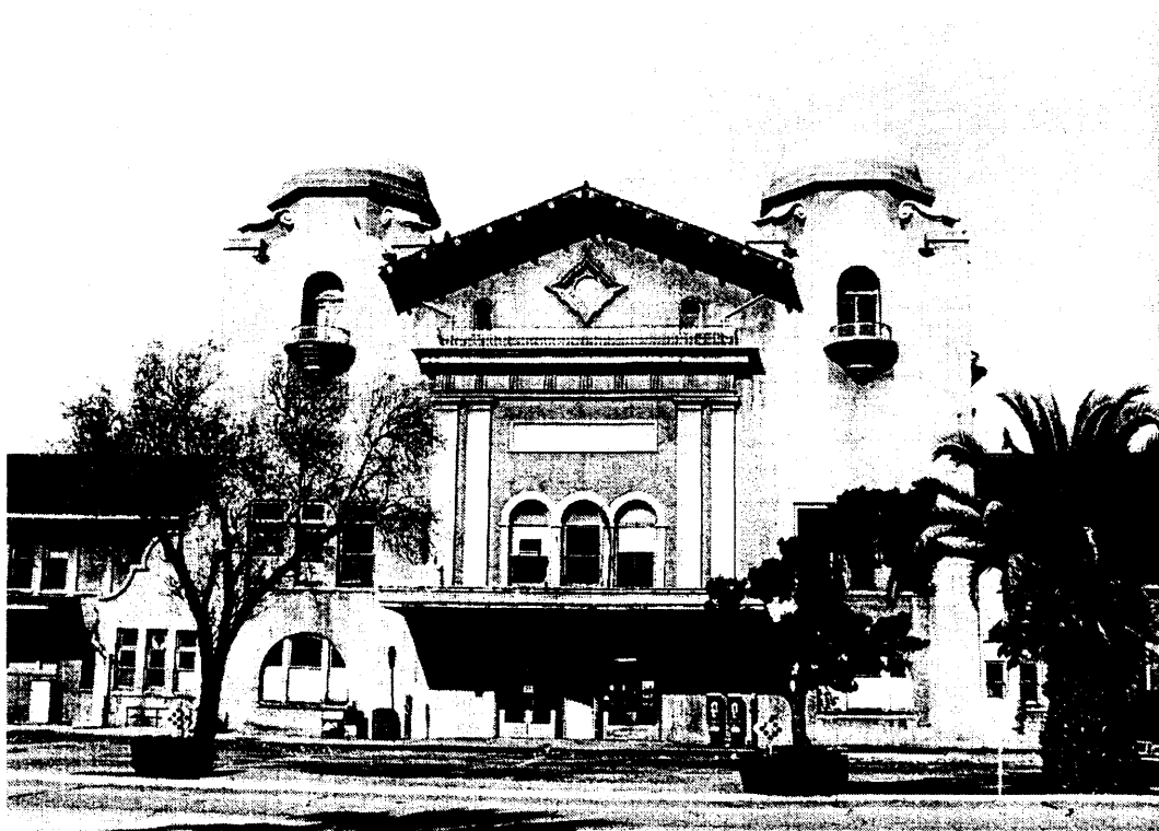
Photo 7: South facade of the main entry to the Depot, facing north.
