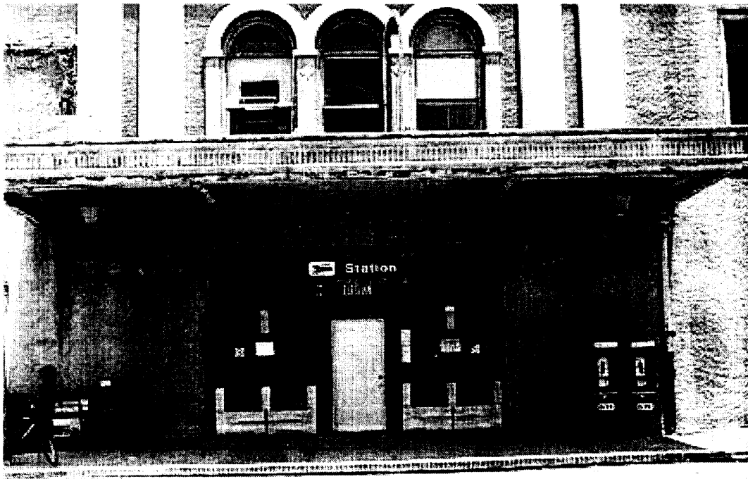
Photo 8: Entry doors into the Amtrak station, facing north.
