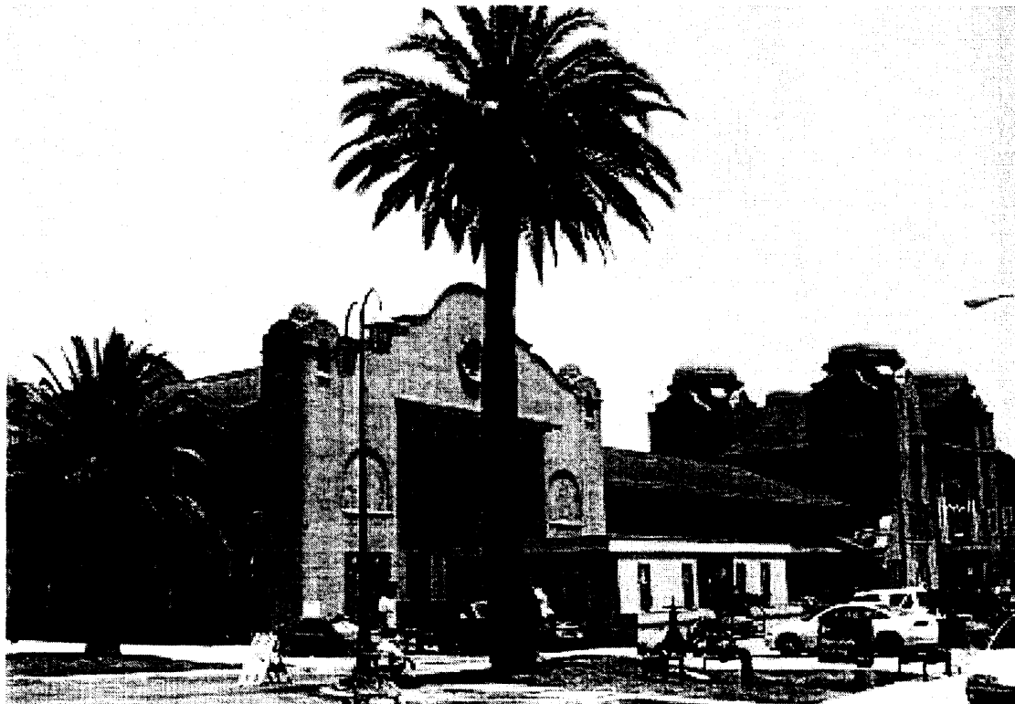
Photo 15: Southwest corner of the Depot facing northeast. Compare to Historical Photo C.
