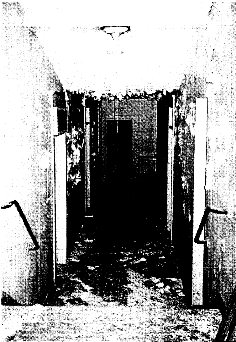
Photo 64: Water damage at corridor of the original residential spaces of the Harvey Girls, facing east.
