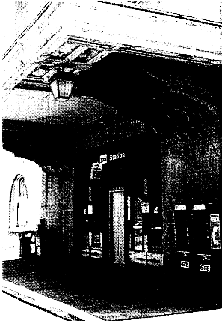
Photo 9: Entry doors into the Amtrak passenger lobby showing overhang, facing northwest.
