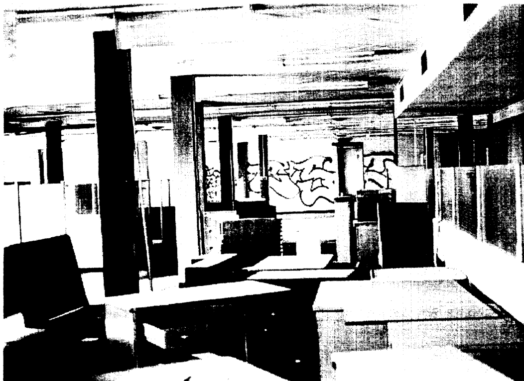
Photo 55: Open office area with circa 1940s metal partitions and furred down ceiling for HVAC, facing west.
