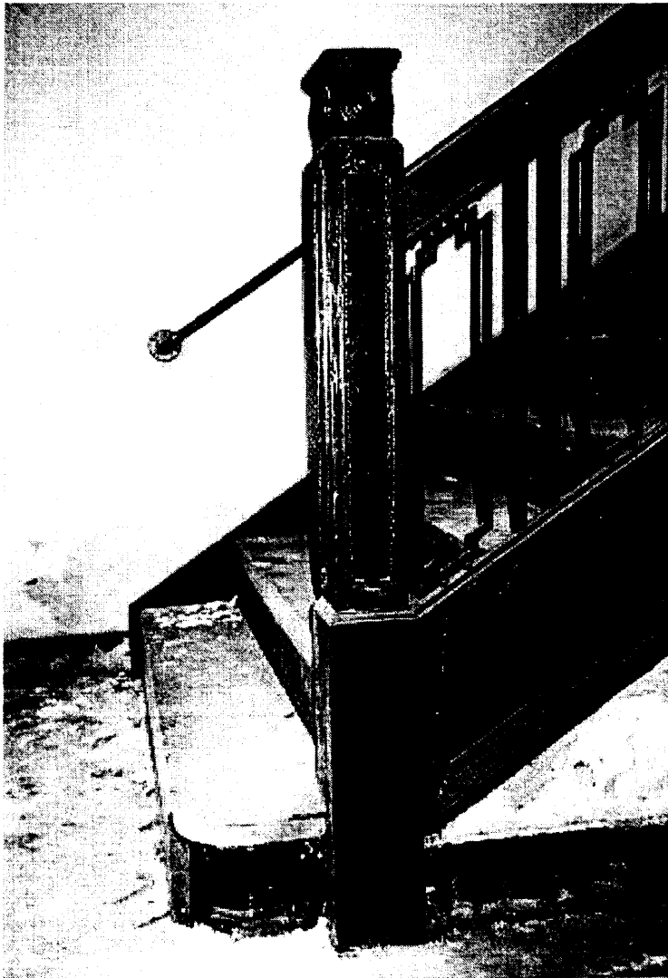
Photo 46: Extant original stair with metal newel post and railing at employee lobby, facing east. The original marble threads have been covered with a rubber molding.
