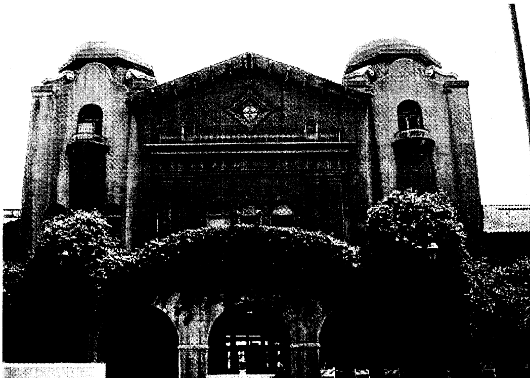
Photo 19: Main entrance at the north facade (track side), facing south.
