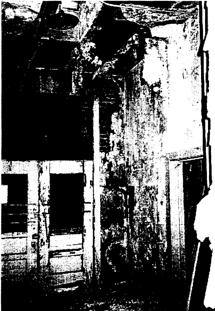
Photo 53: Water damage at plaster wall and ceiling in Harvey House corridor, facing east.
