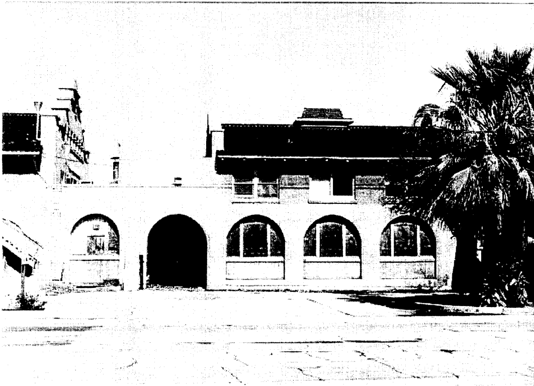
Photo 14: South facade showing Harvey House addition, facing north.
