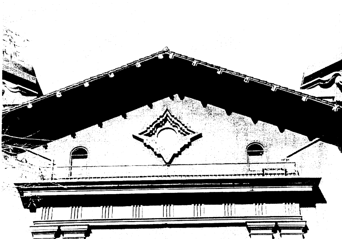
Photo 10: Detail of the false balcony and raking eave above Amtrak entry, facing north.
