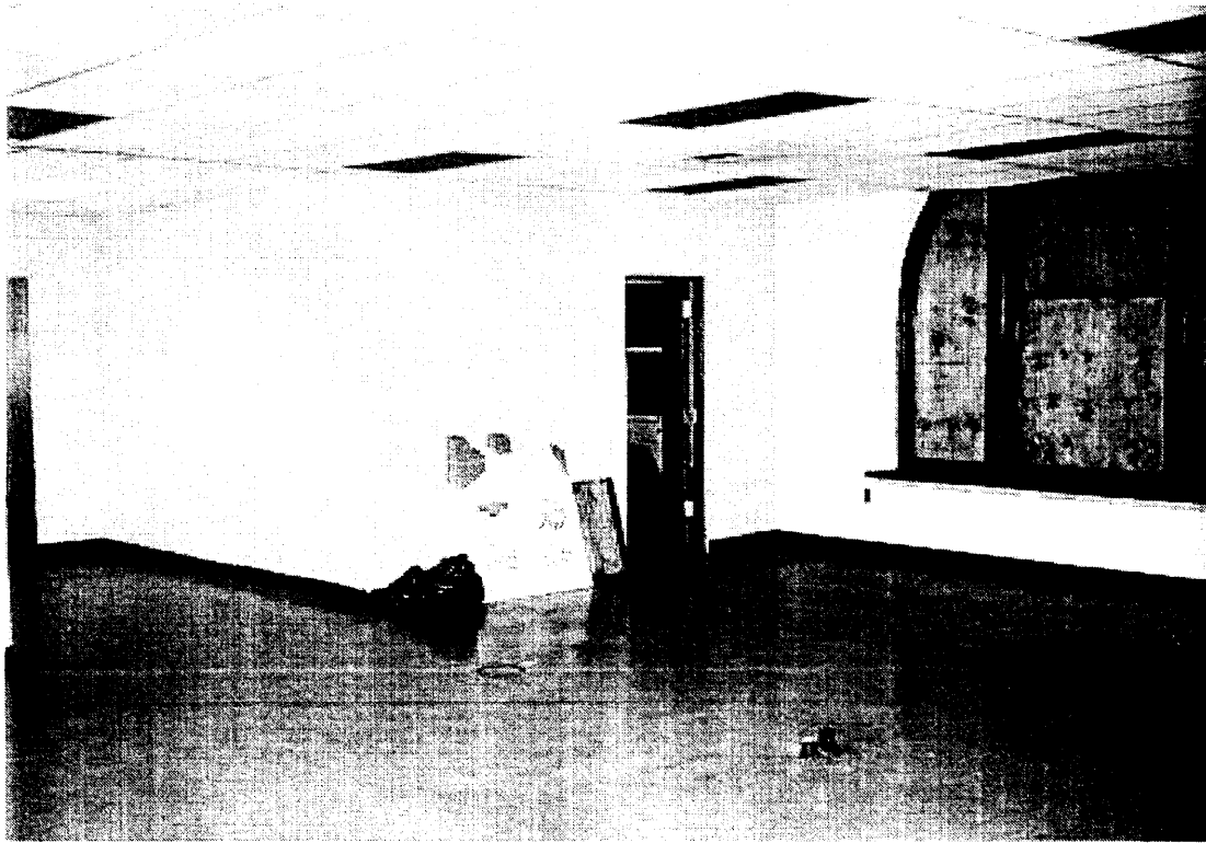
Photo 48: Suspended ceiling blocking view of arched window and temporary partition in original Harvey House, facing northwest.
