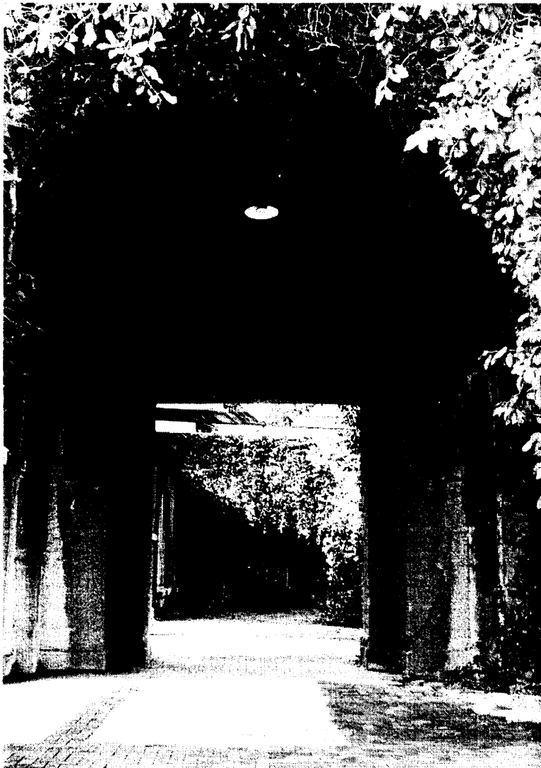
Photo 23: View through the covered north arcade, facing east.
