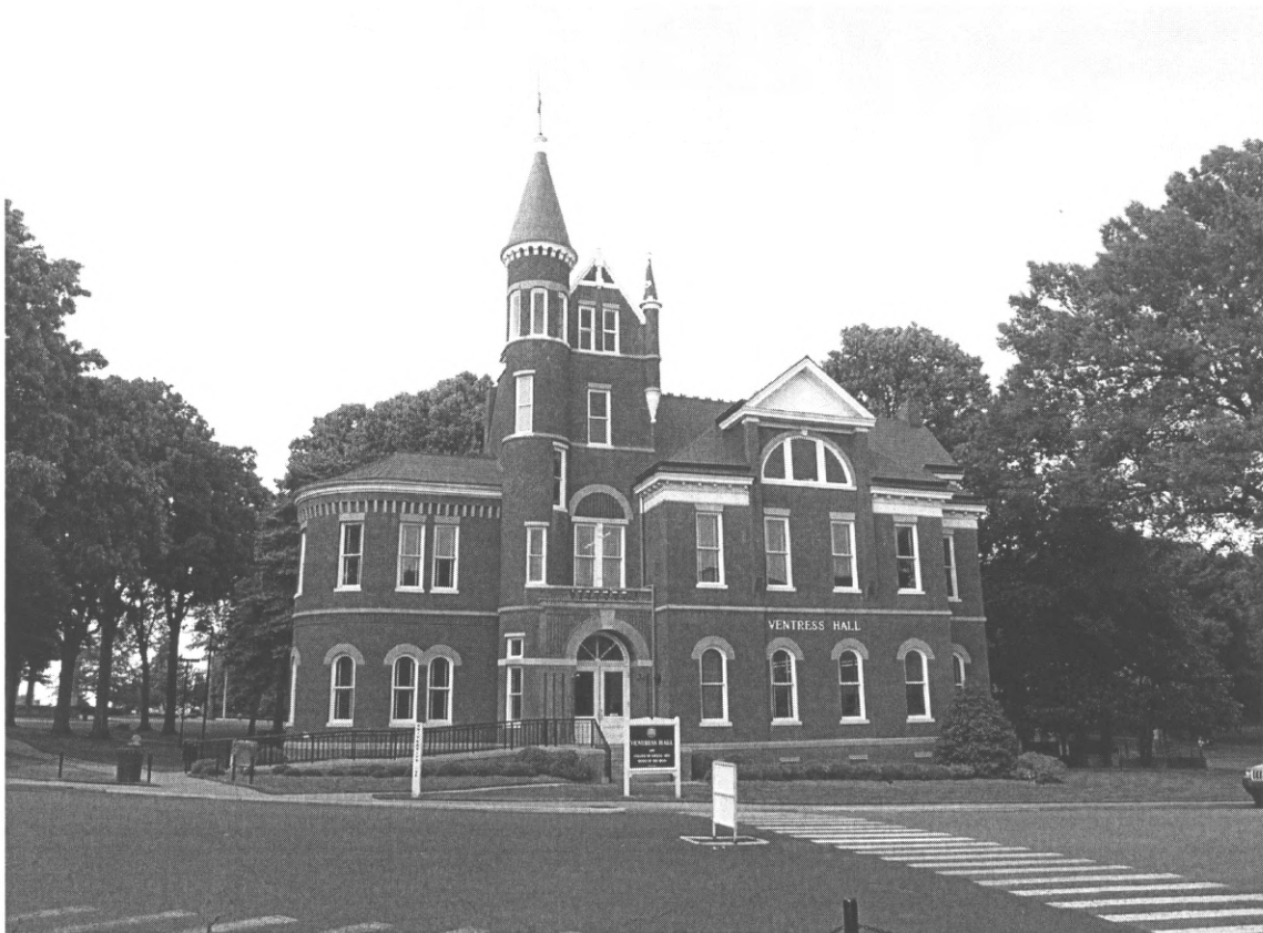
Ventress Hall, facing northeast. Photograph by Gene A. Ford, May 2005.
