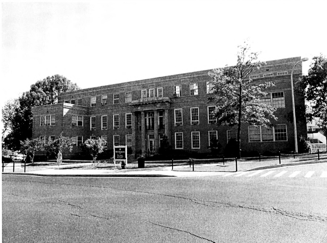
Old Chemistry building, facing south. Photograph by Gene A. Ford, May 2005.
