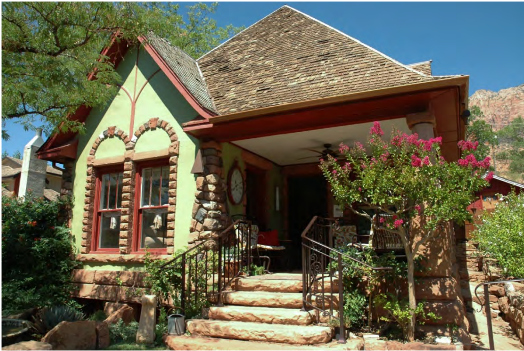
Photograph 3 East elevation of residence. Camera facing west.
