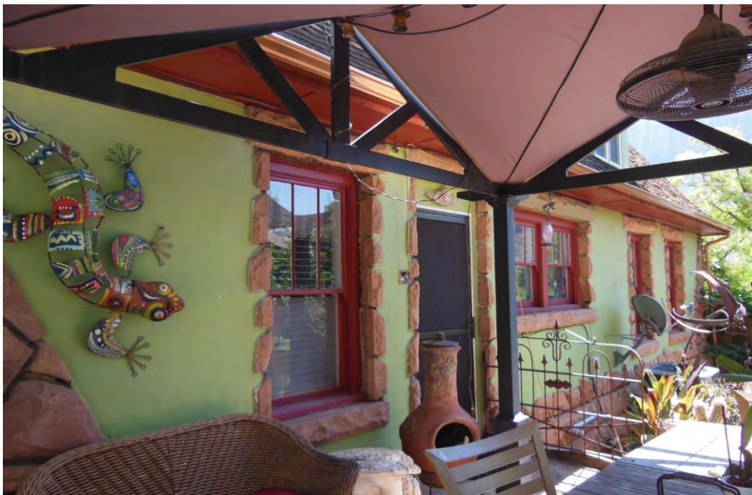
Photograph 6 South elevation of residence. Camera facing east.
