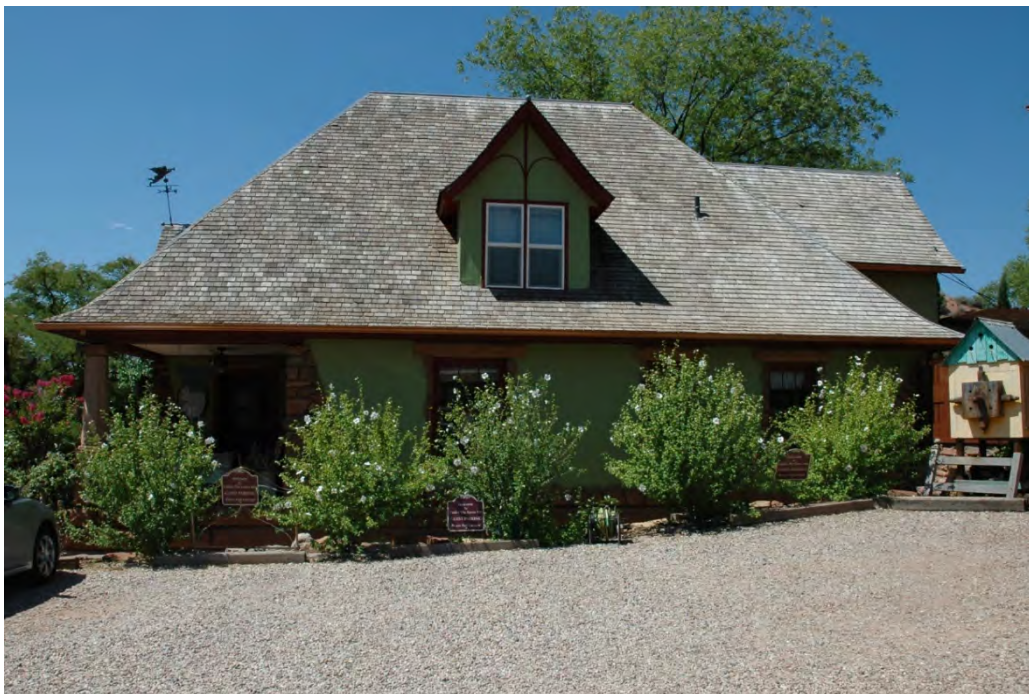
Photograph 4 North elevation of residence. Camera facing southwest.
