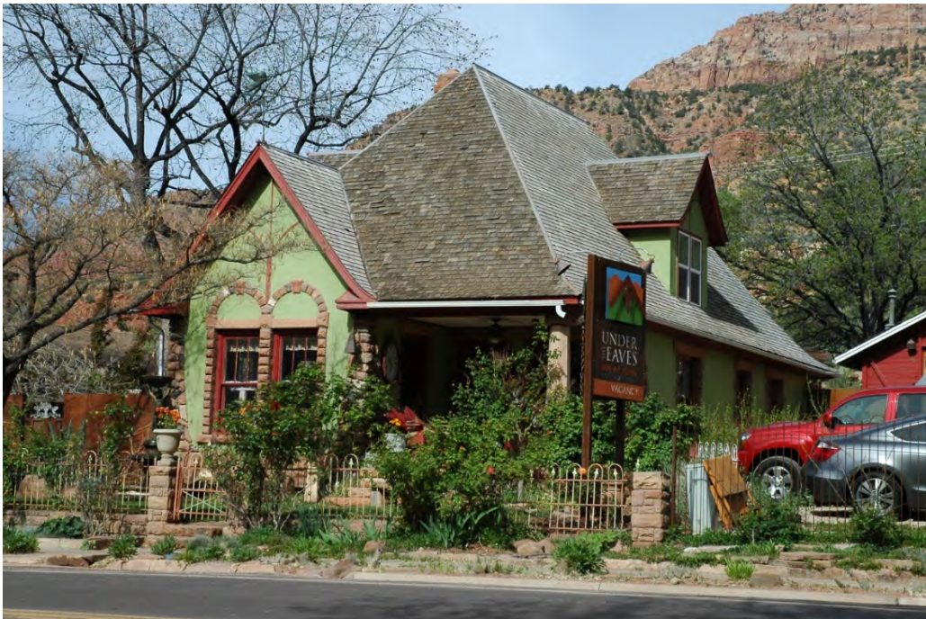
Photograph 2 East and north elevations of residence. Camera facing west.
