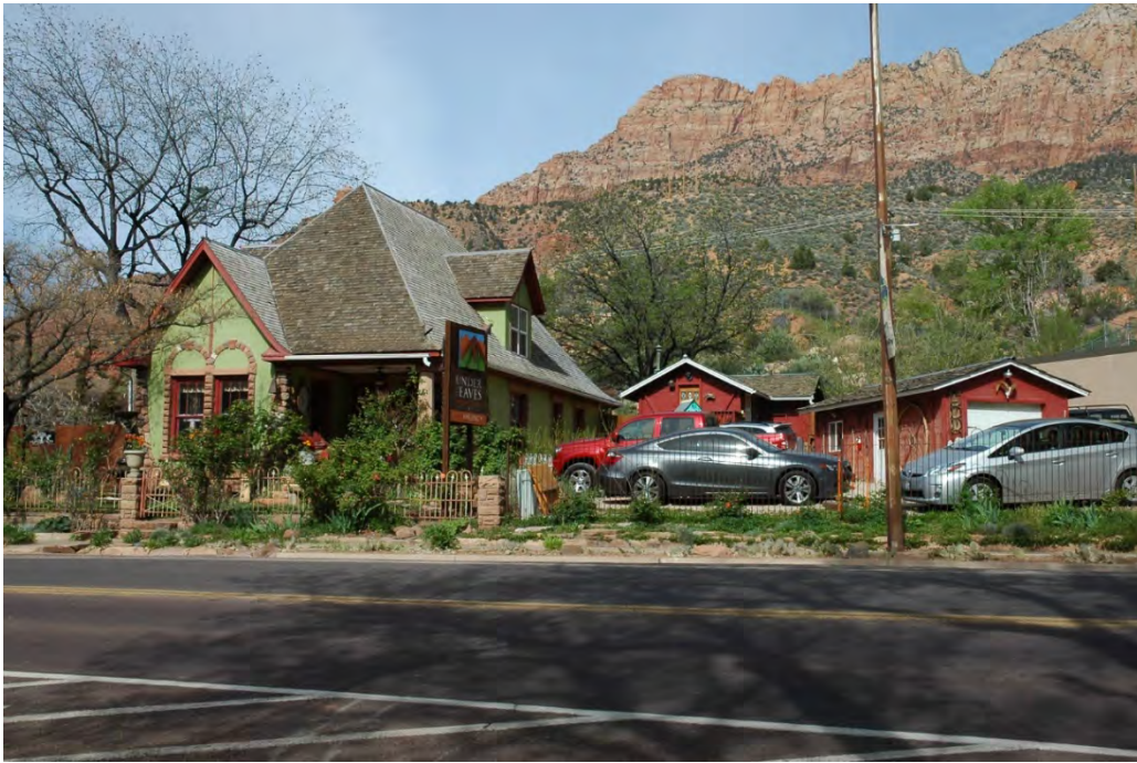
Photograph 1 View of residence, outbuildings and site. Camera facing west.
