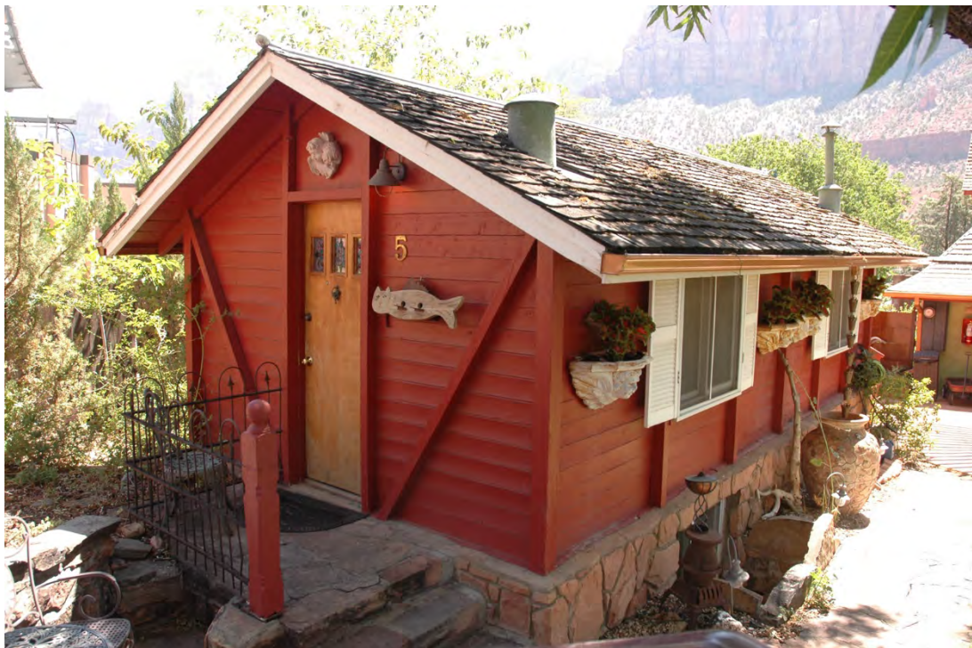
Photograph 18 North and west elevations of cottage. Camera facing southeast.
