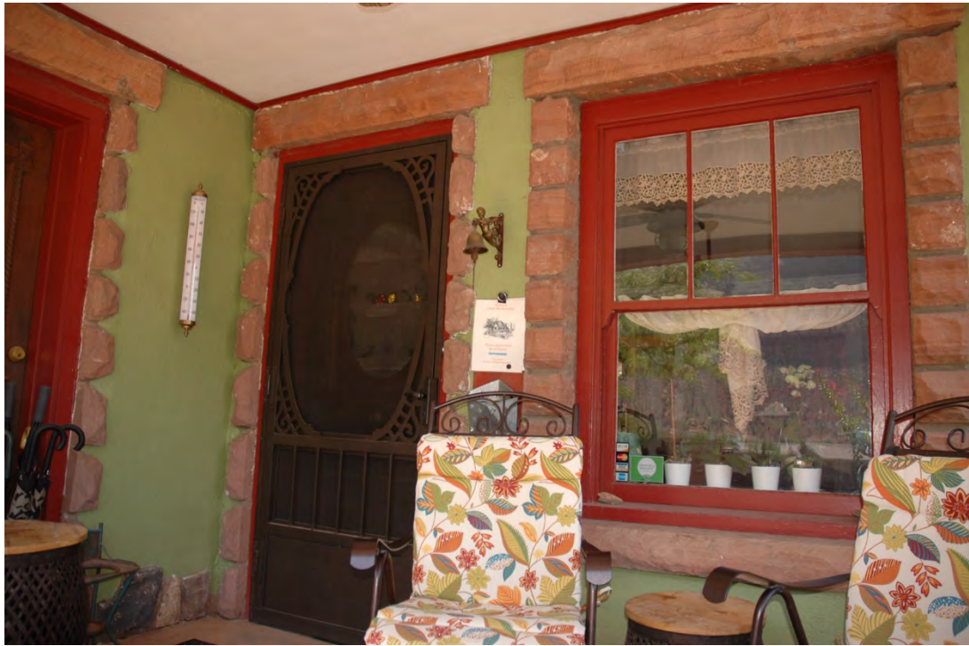
Photograph 9 East elevation, door and window detail. Camera facing north.
