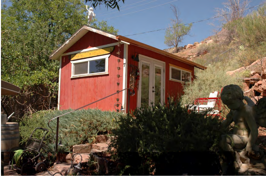
Photograph 21 South and east elevations of cabin. Camera facing west.
