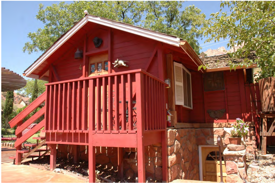
Photograph 17 West elevations of cottage. Camera facing west.
