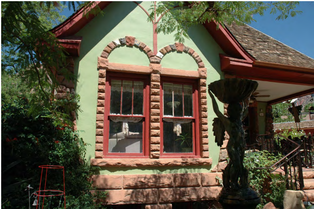
Photograph 8 East elevation of residence, window detail. Camera facing north.
