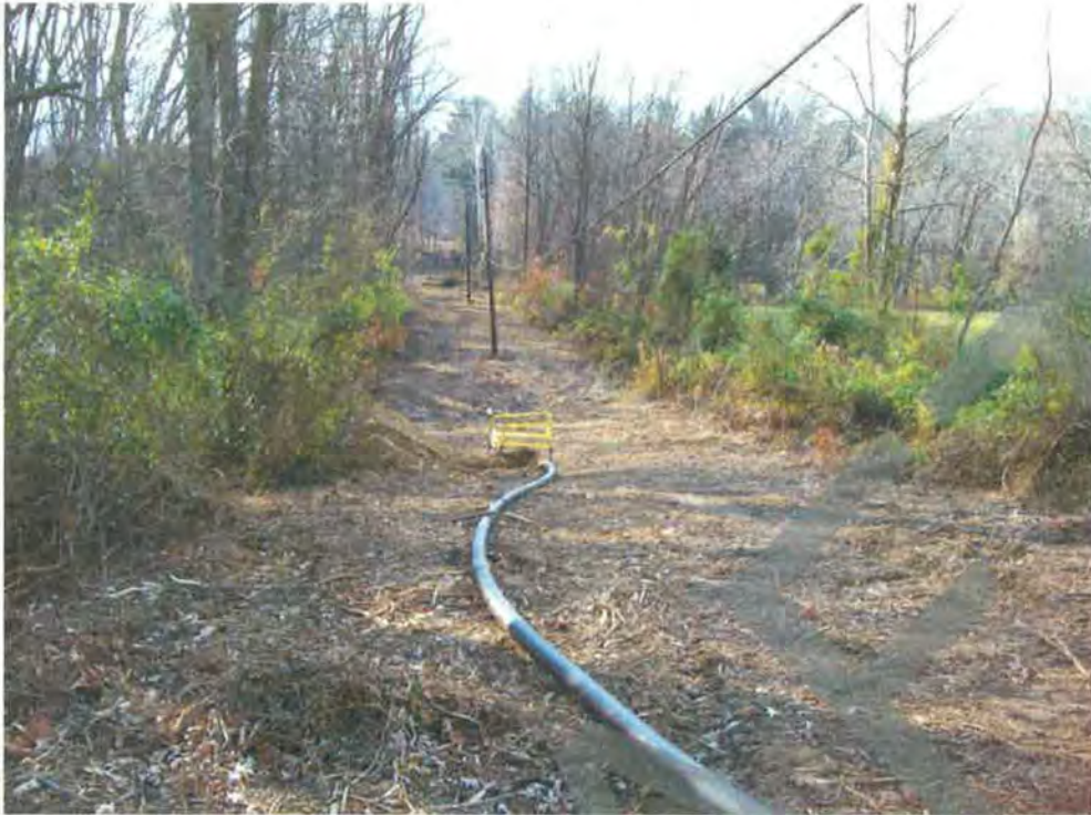
Photo 15: Looking south down utility easement and portions of Wetland 3 (November 11, 2014)
