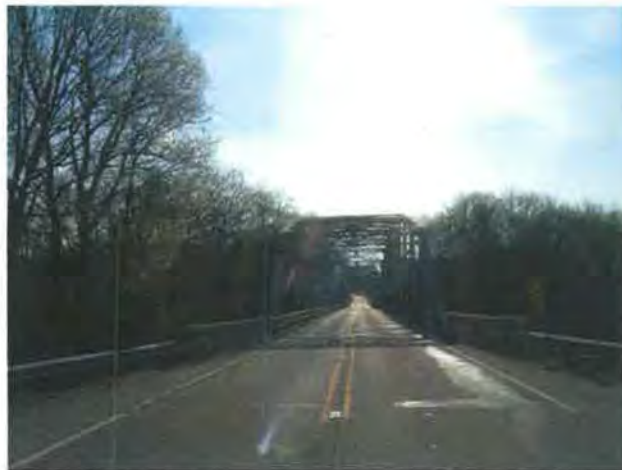
Photo 11: Standing on SR 46 looking east at the bridge.
