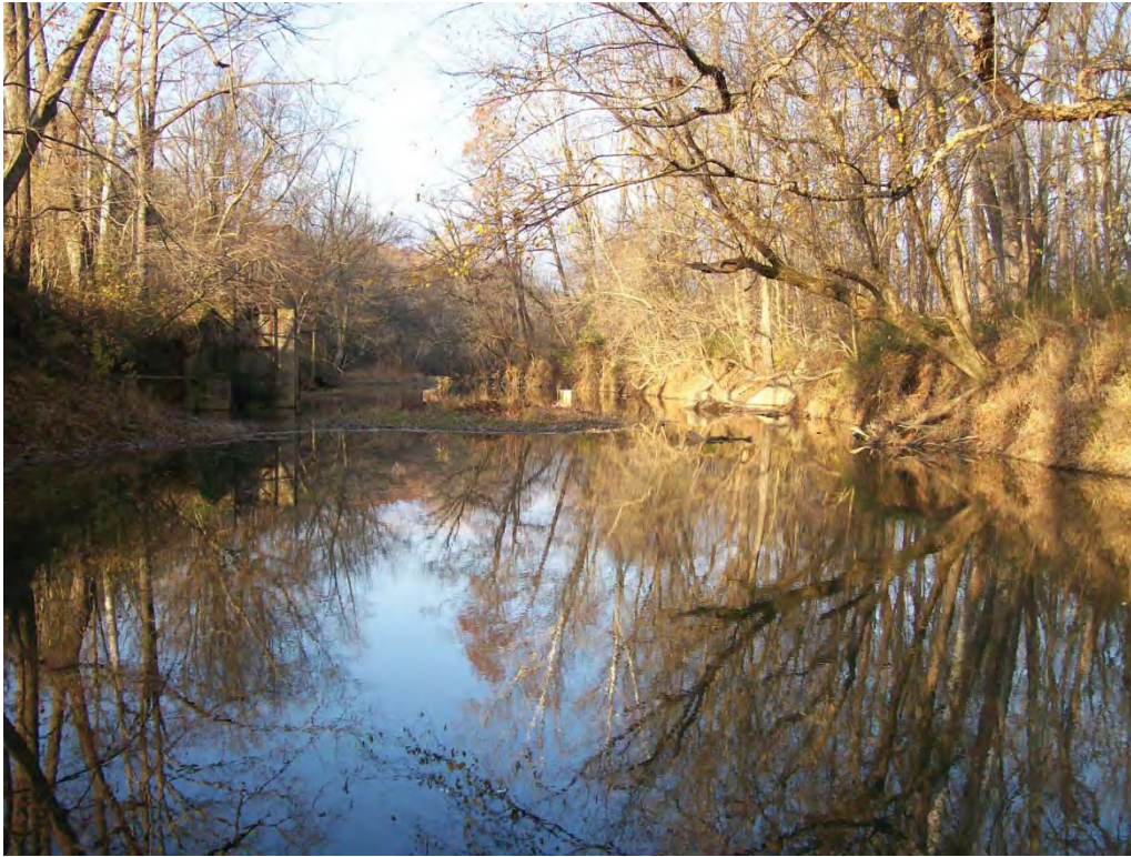
Photo 14: East bridge looking downstream (west) at old dam
