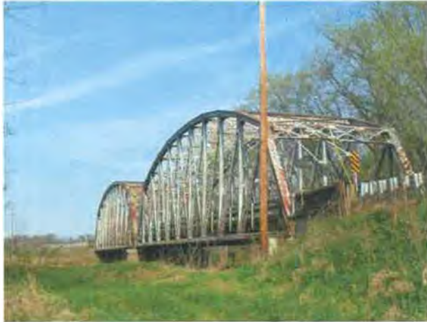
Photo 25: Standing in the floodplain, looking northwest at the bridge.
