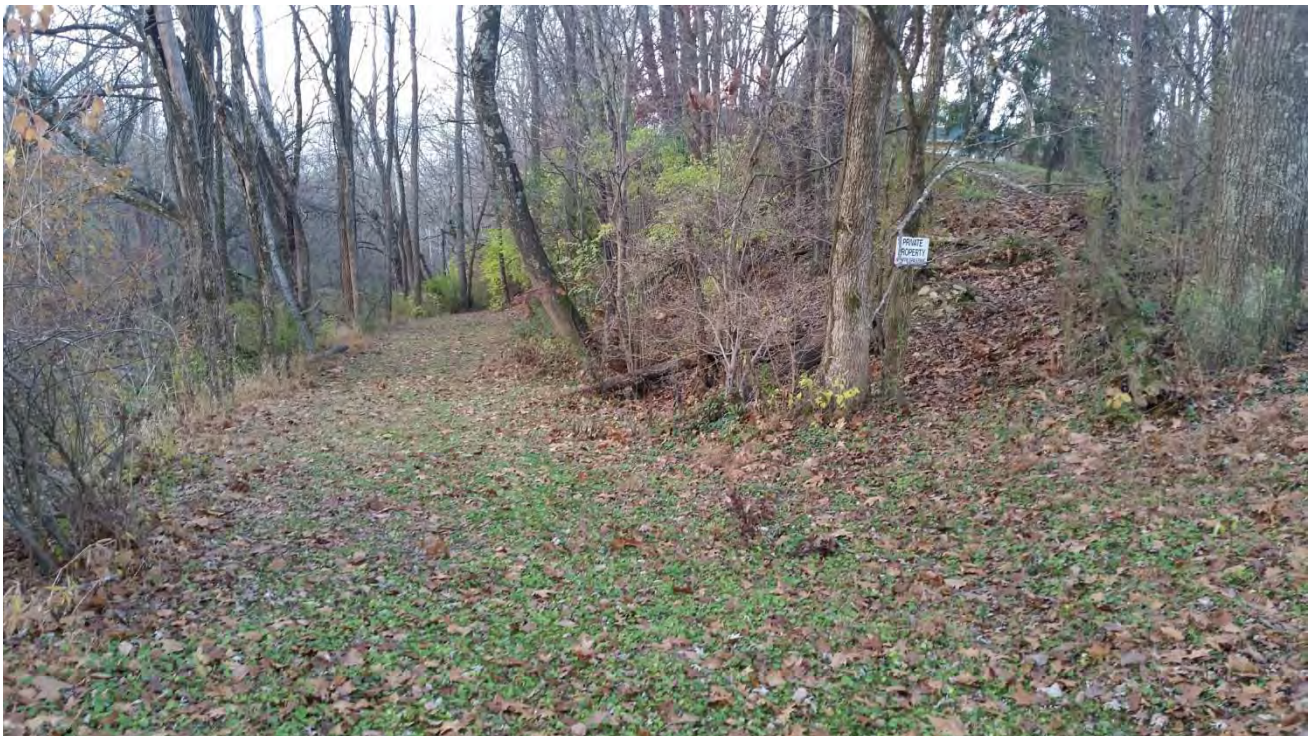
Photo 2: West bridge looking south just north of west abutment.
