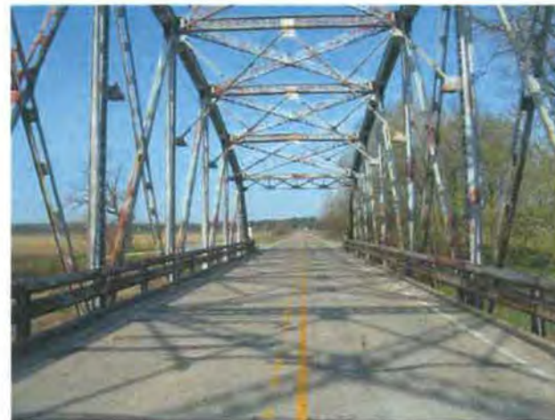
Photo 12: Standing on the bridge looking west.
