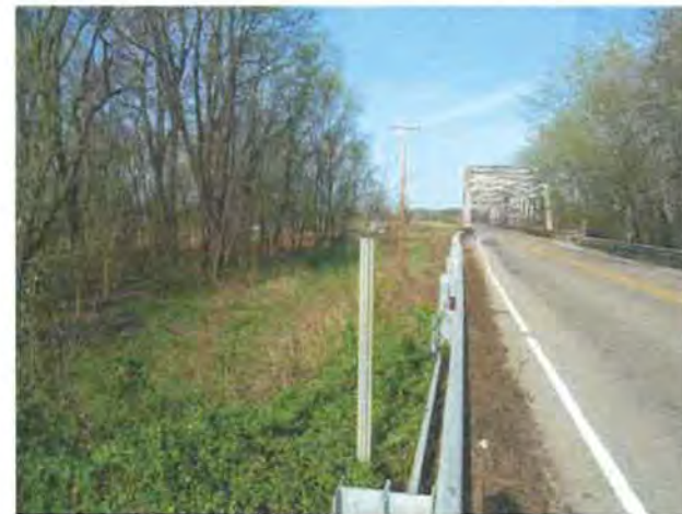
Photo 24: View of the SE shoulder.
