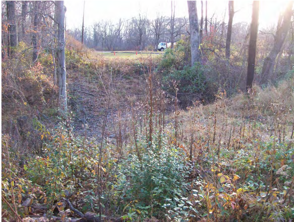
Photo 12: East bridge looking east from south bank
