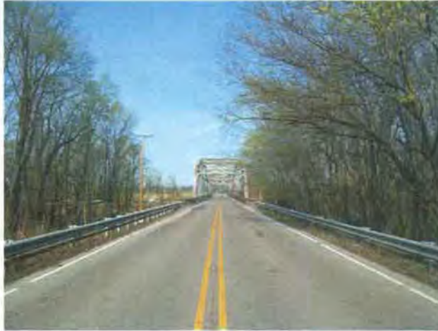
Photo 21: Standing on SR 46 facing west towards the bridge.
