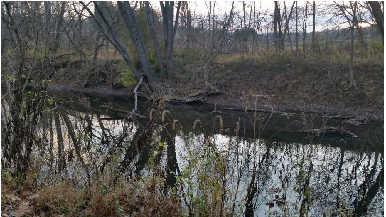
Photo 1: West bridge looking east from near west abutment.
