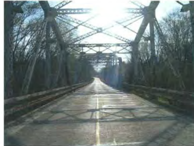
Photo 14: Standing on the bridge looking east.
