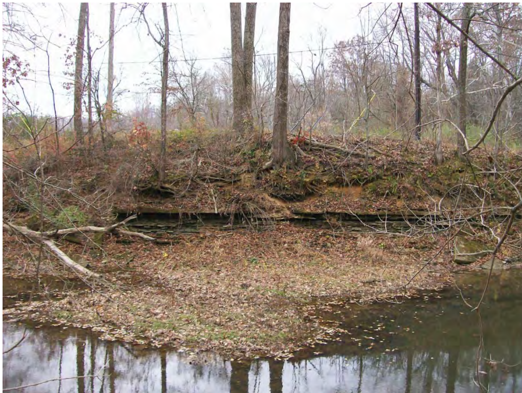
Photo 17: East bridge looking south at south bank from north bank
