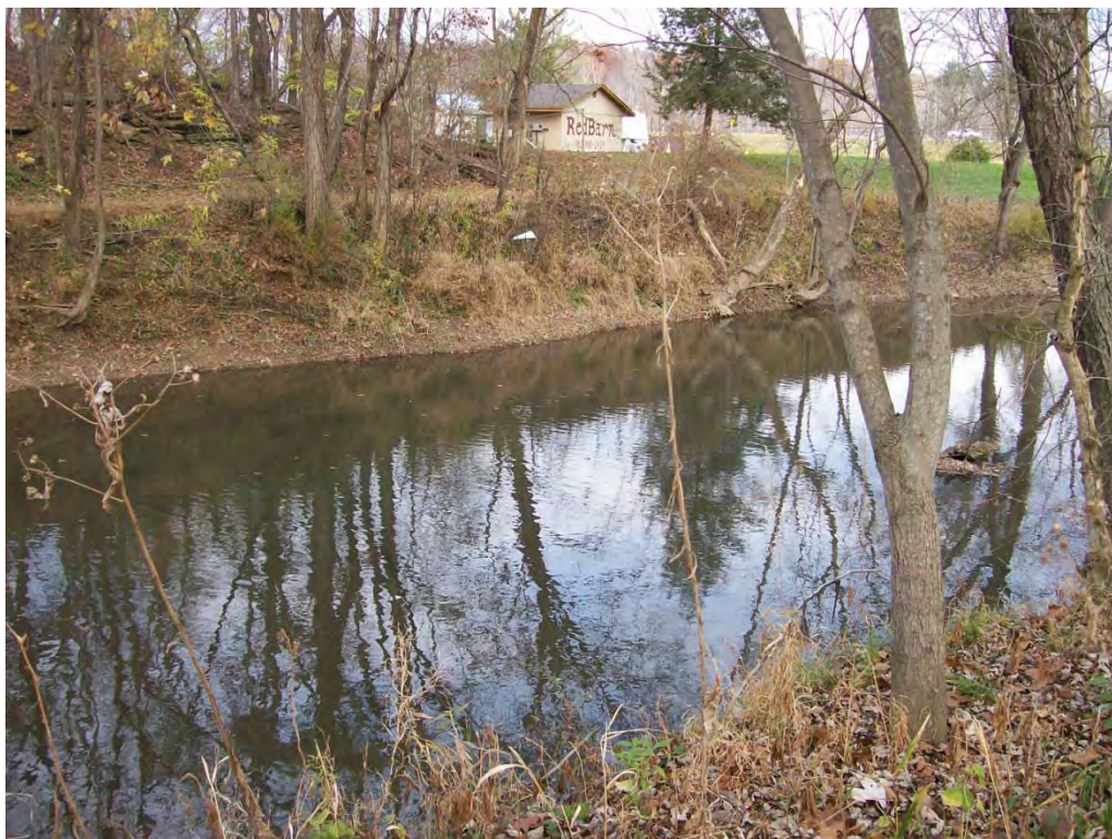
Photo 6: West bridge looking west from east bank at area of west abutment.
