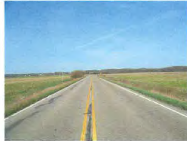
Photo 2: Standing on SR 46 facing west.
