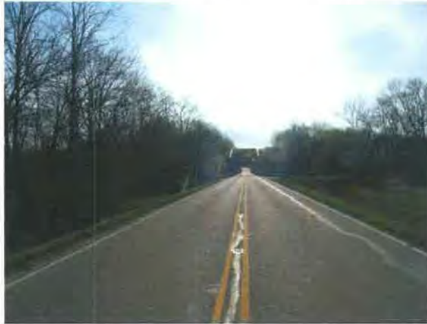
Photo 1: Standing on SR 46 facing east towards the bridge (Bridge # 046-11-01316A).
