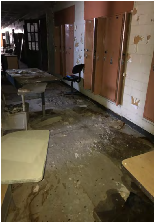
Photo 10: Interior, Second floor, Corridor
