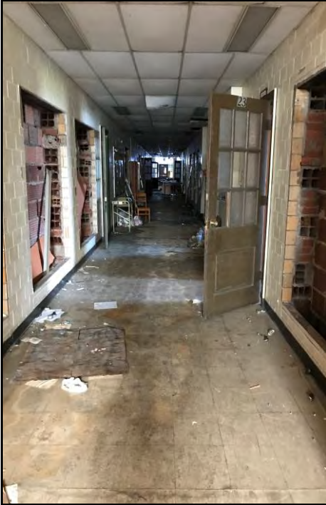
Photo 8: Interior, First floor, Corridor
