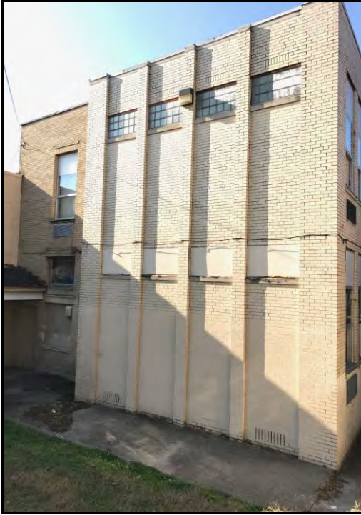
Photo 6: South Elevation (rear), 1953 addition
