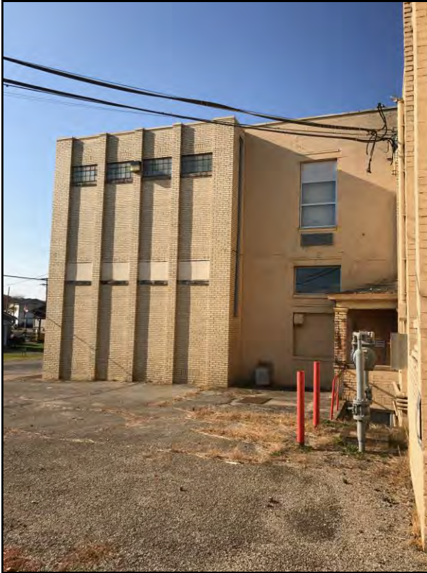
Photo 4: South Elevation, Showing rear of 1957 addition
