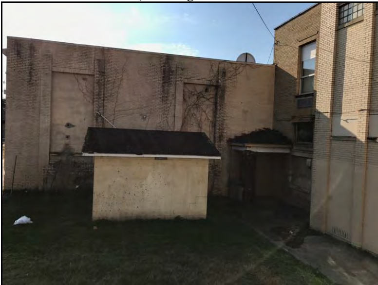
Photo 5: South and East Elevations, Showing east elevation of gymnasium
