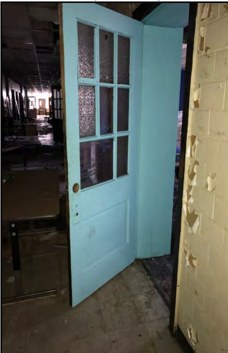
Photo 9: Interior, First floor, Classroom entrance door
