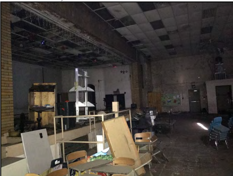
Figure 13: Interior, First floor. Gymnasium/Auditorium, Stage shown on left
