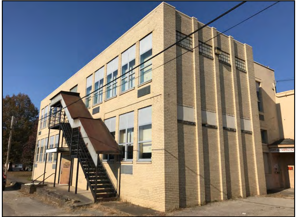
Photo 2: West Elevation, 1957 addition
