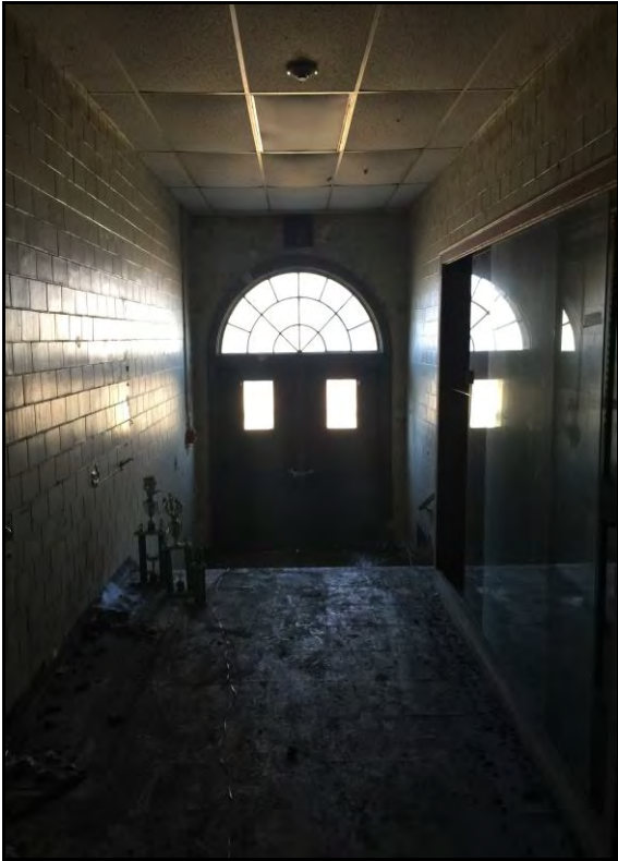
Photo 14: Interior, First floor, Entry door and fanlight
