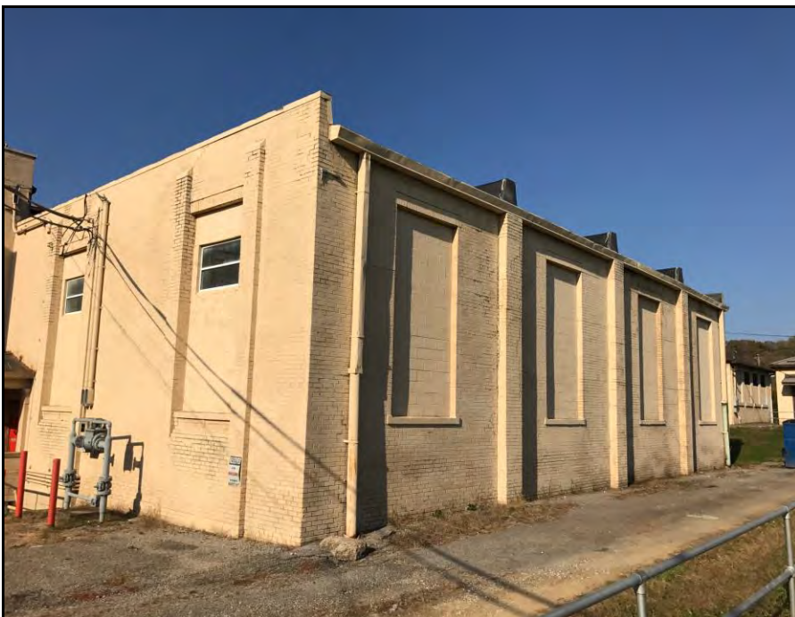
Photo 3: South Elevation, showing rear elevation of gymnasium
