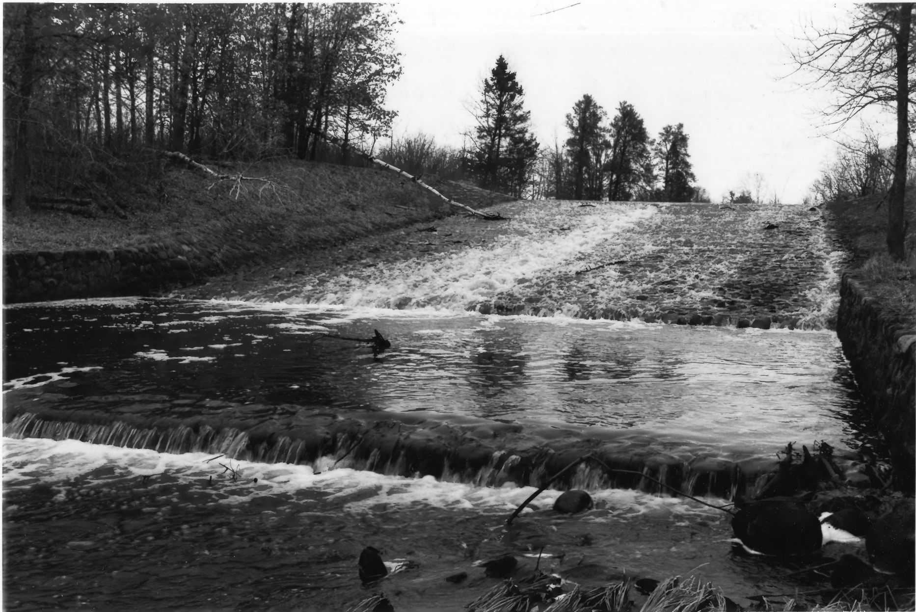
ST. CROIX STATE PARK PINE CO. MN STRUCTURE #73 PHOTO I.D. 09580#6
