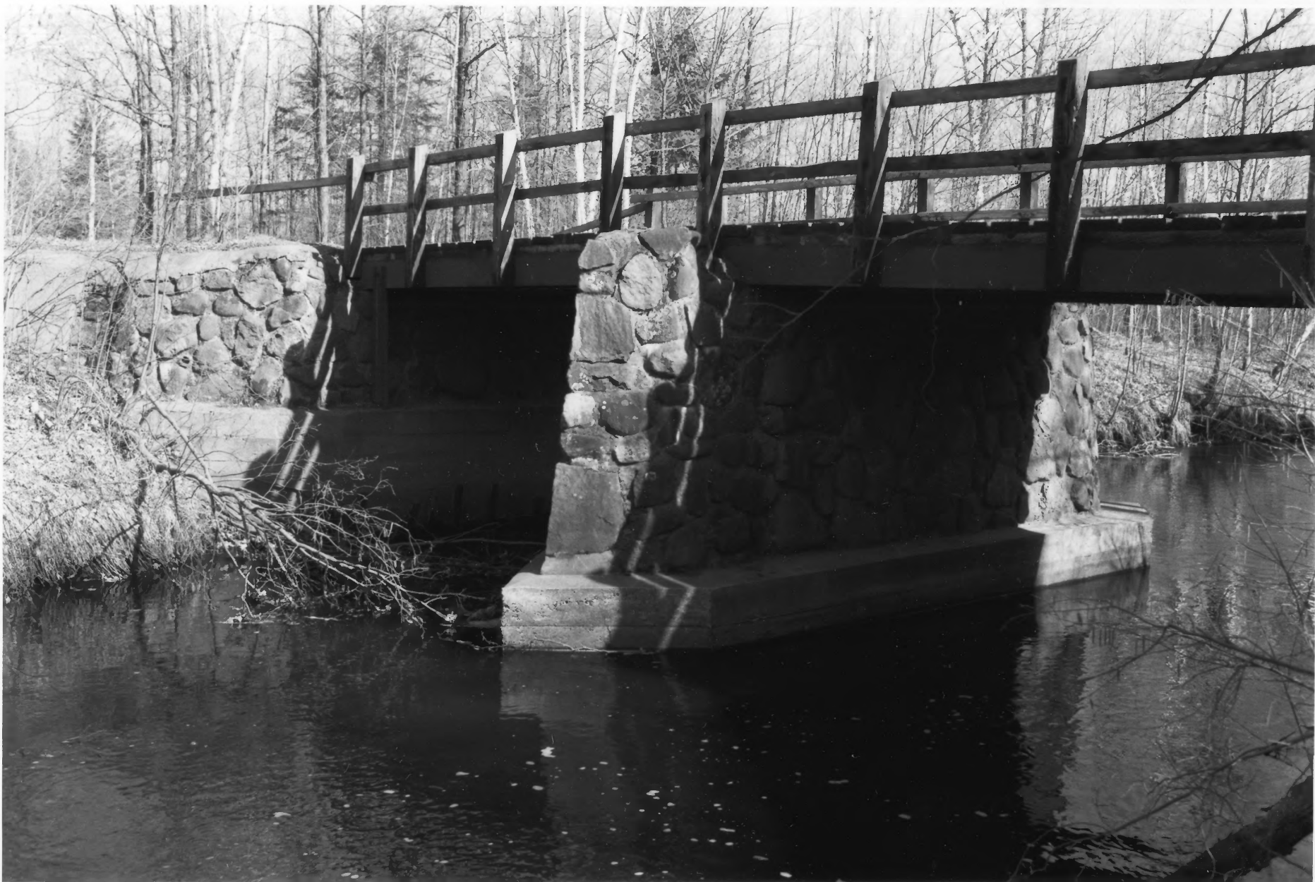
ST. CROIX STATE PARK PINE CO. MN STRUCTURE # 80 PHOTO I.D. 09585 # 25
