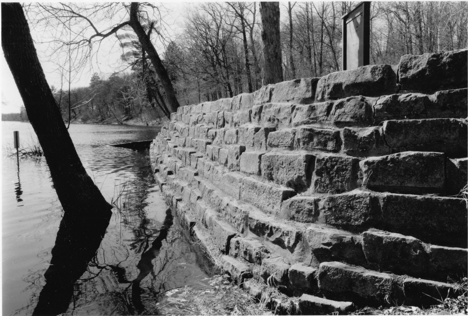
Retaining Wall #27 St. Croix Recreational Demonstration Area Pine Co., Mn 012211-1
