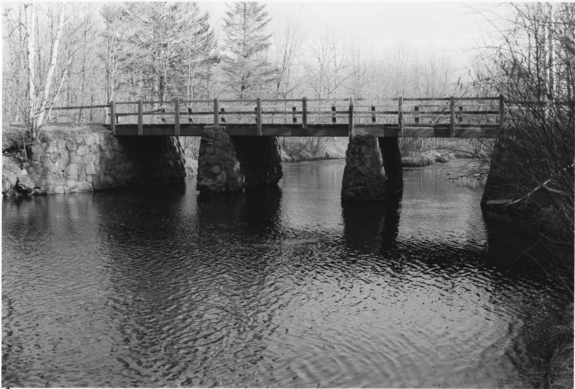
Sand Creek Bridge #77 St. Croix Recreational Demonstration Area Pine Co., Mn 09584-5
