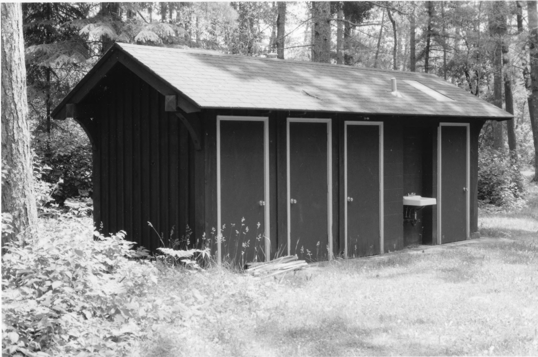
Unit Latrine #48 St. Croix Recreational Demonstration Area Pine Co., Mn 012610-13
