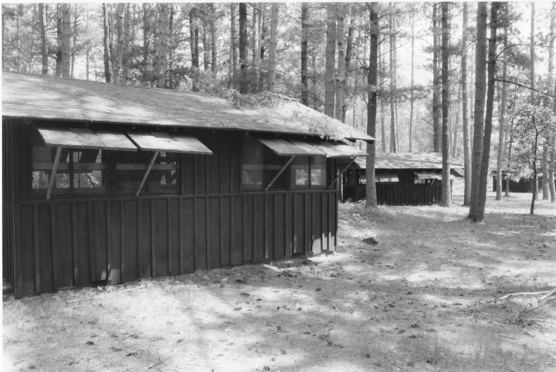
Unit Cabins # 46 St. Croix Recreational Demonstration Area Pine Co., Mn 012610-6
