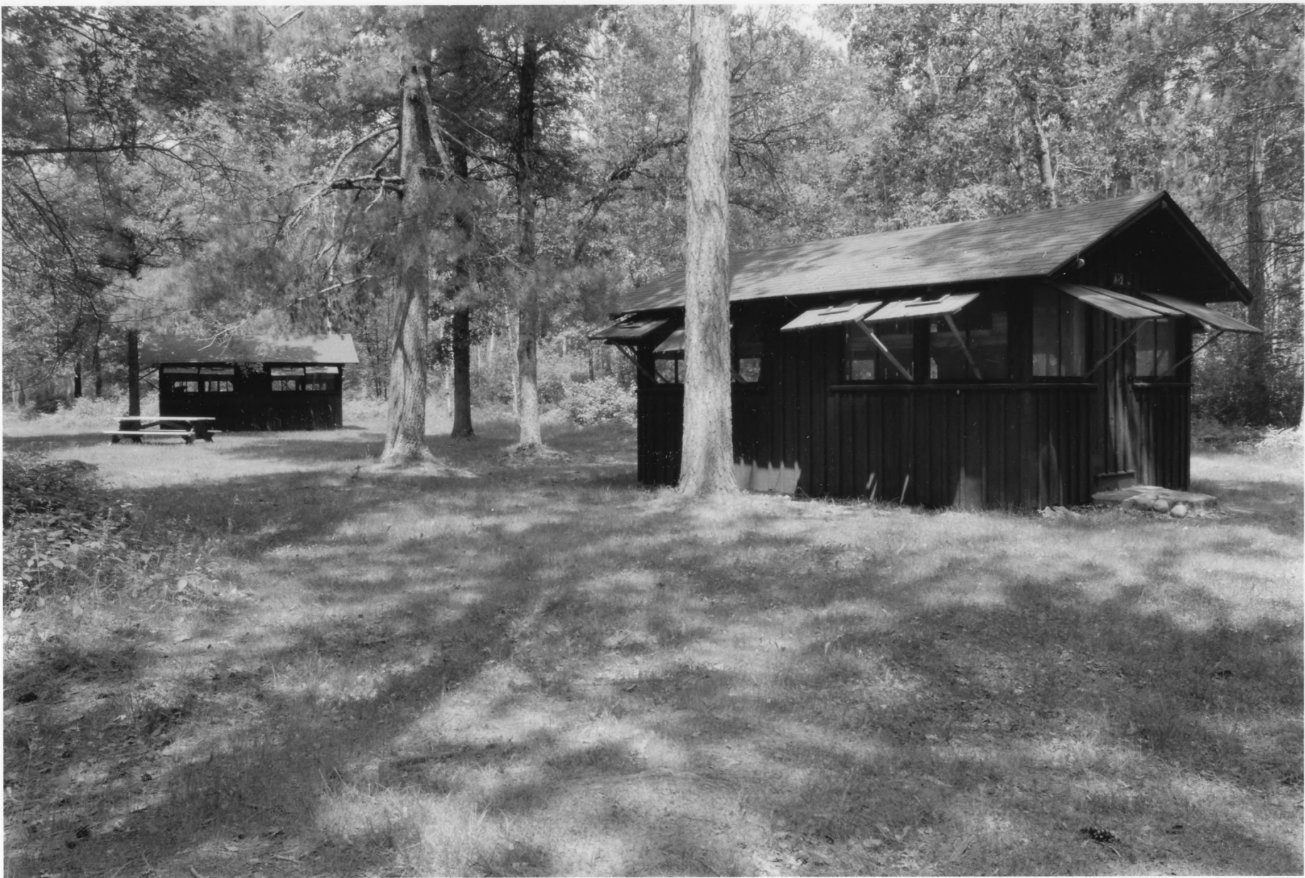
Unit Cabin #46 St. Croix Recreational Demonstration Area Pine Co., Mn 012610-2
