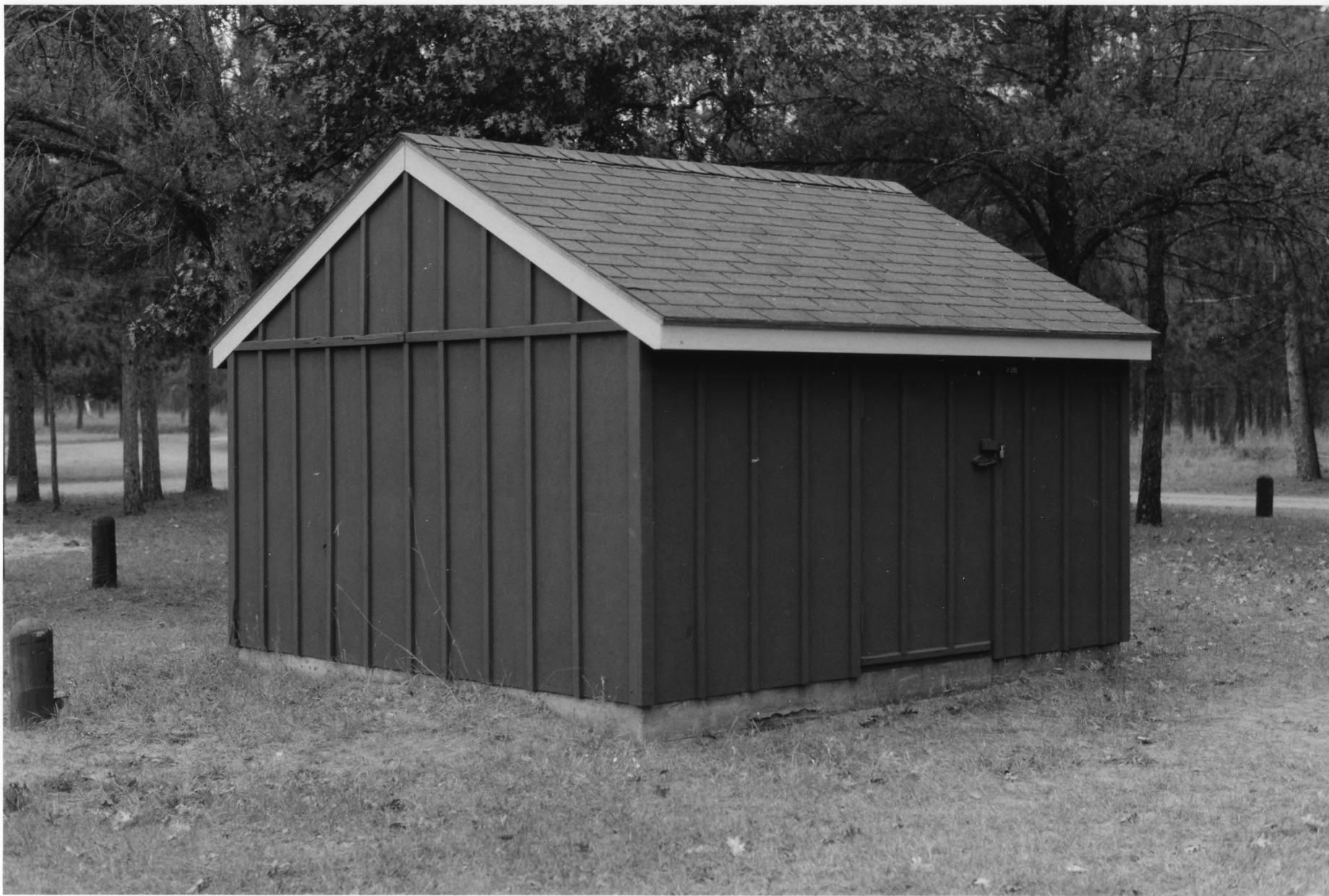
PUMPHOUSE (NON-CONTRIBUTING) ST CROIX RECREATIONAL DEMONSTRATION AREA PINE CO., MN 012213 - 2
