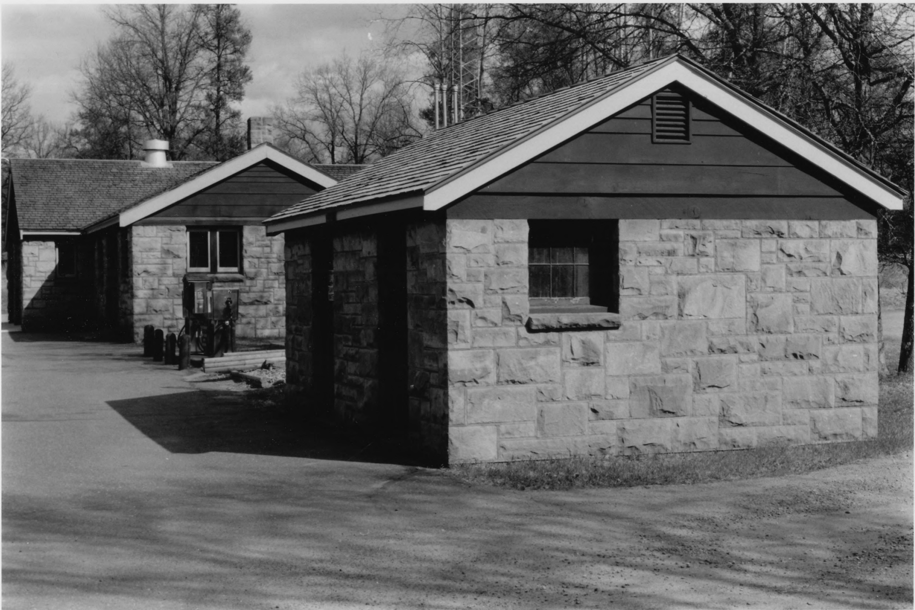
Shop Building and Oil and Paint Building #13 & 14 St. Croix Recreational Demonstration Area Pine Co., Mn 012211-12
