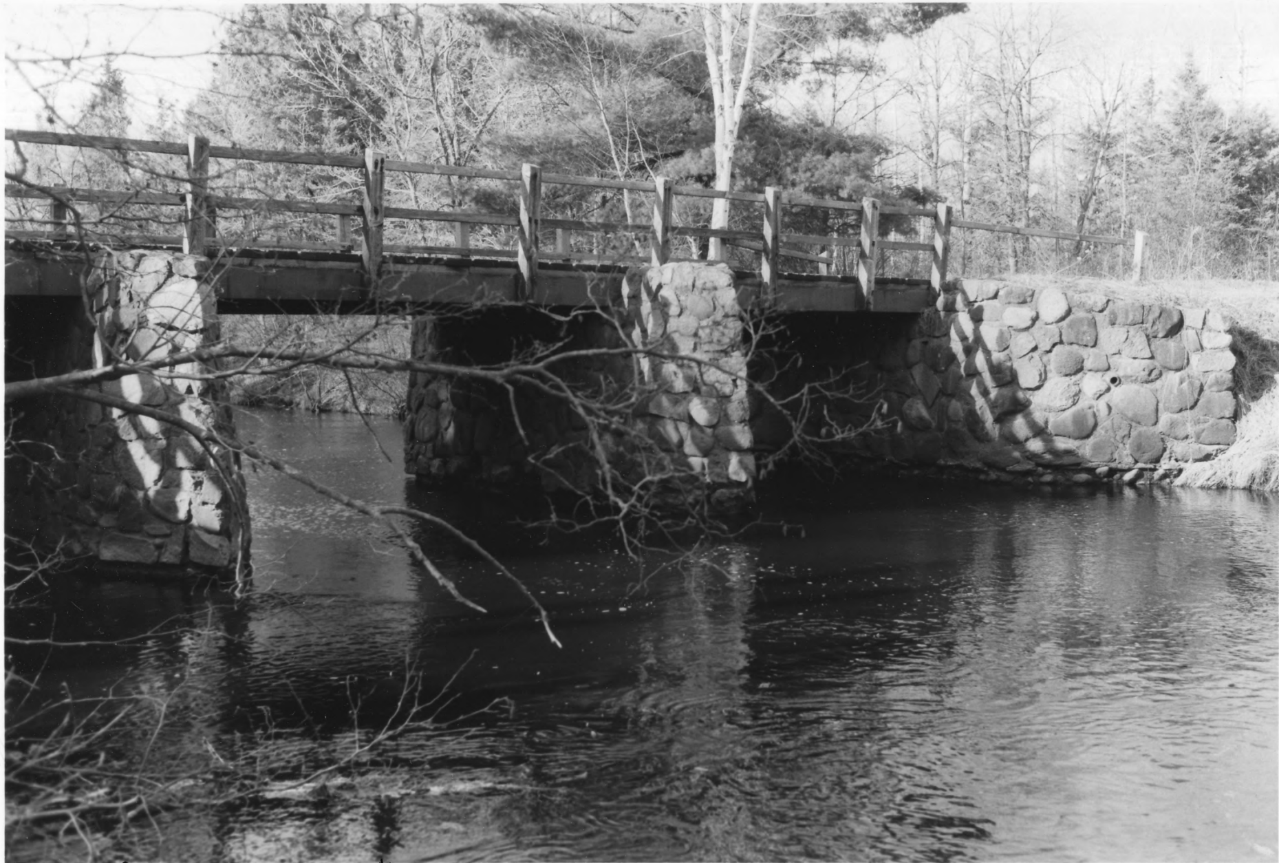
Sand Creek Bridge #77 St. Croix Recreational Demonstration Area Pine Co., Mn 09584-6
