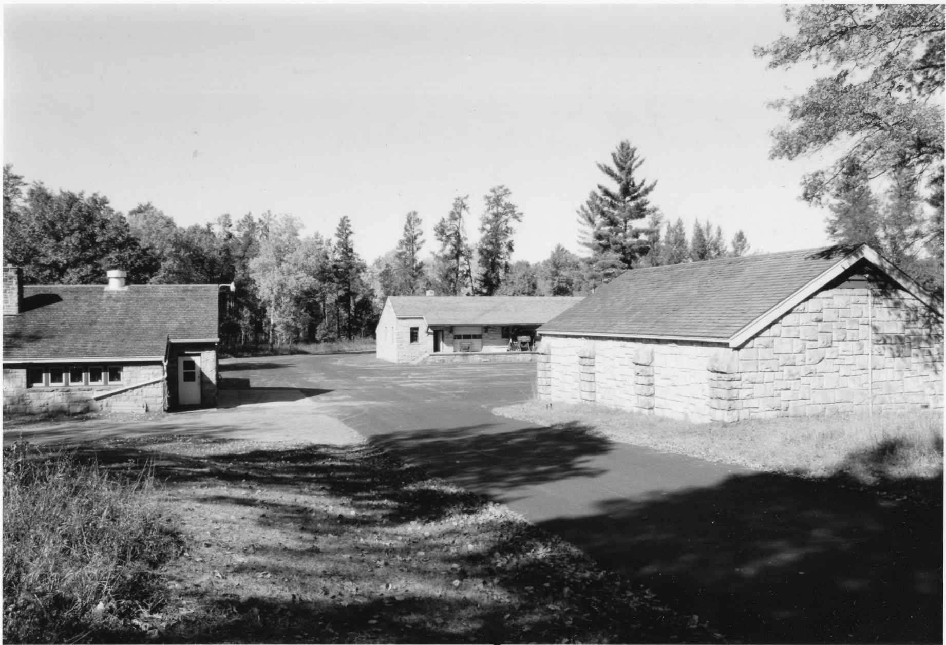
Ice and wood house, warehouse, Shop Building; #10, #12, & #13 St. Croix Recreational Demonstration Area
