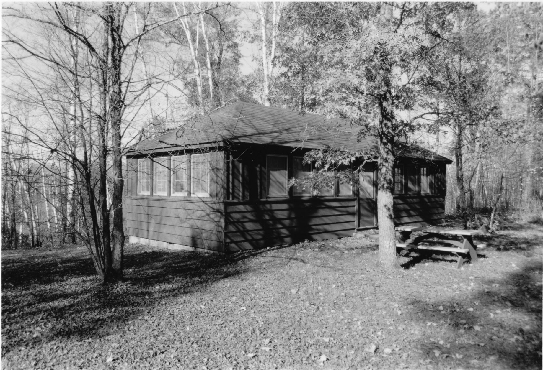
Unit Cabin #93 St. Croix Recreational Demonstration Area Pine Co., Mn 012663-11
