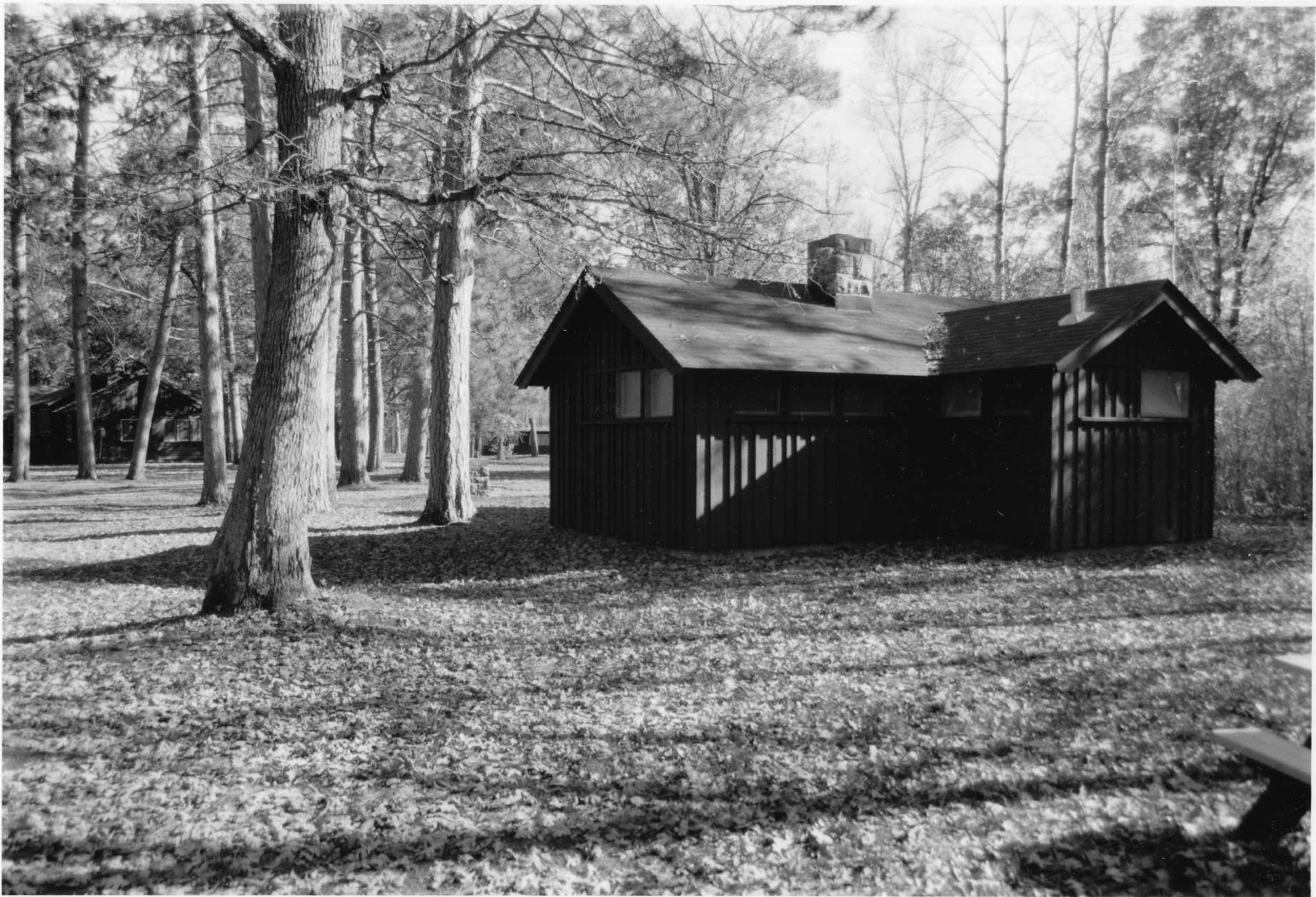
Central Unit Latrine #90 St. Croix Recreational Demonstration Area Pine Co., Mn 012663-12
