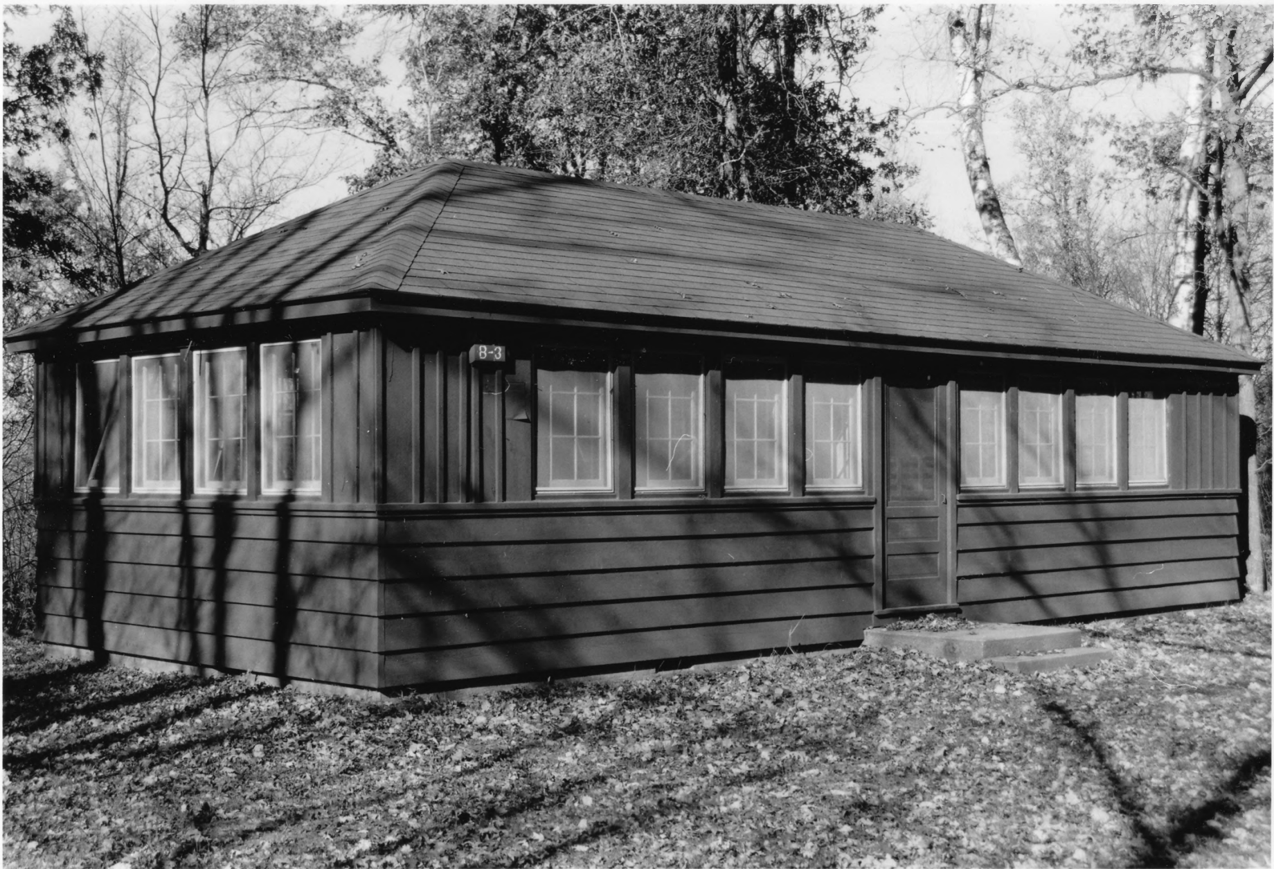
Unit Cabin #93 St. Croix Recreational Demonstration Area Pine Co., Mn 012663-13
