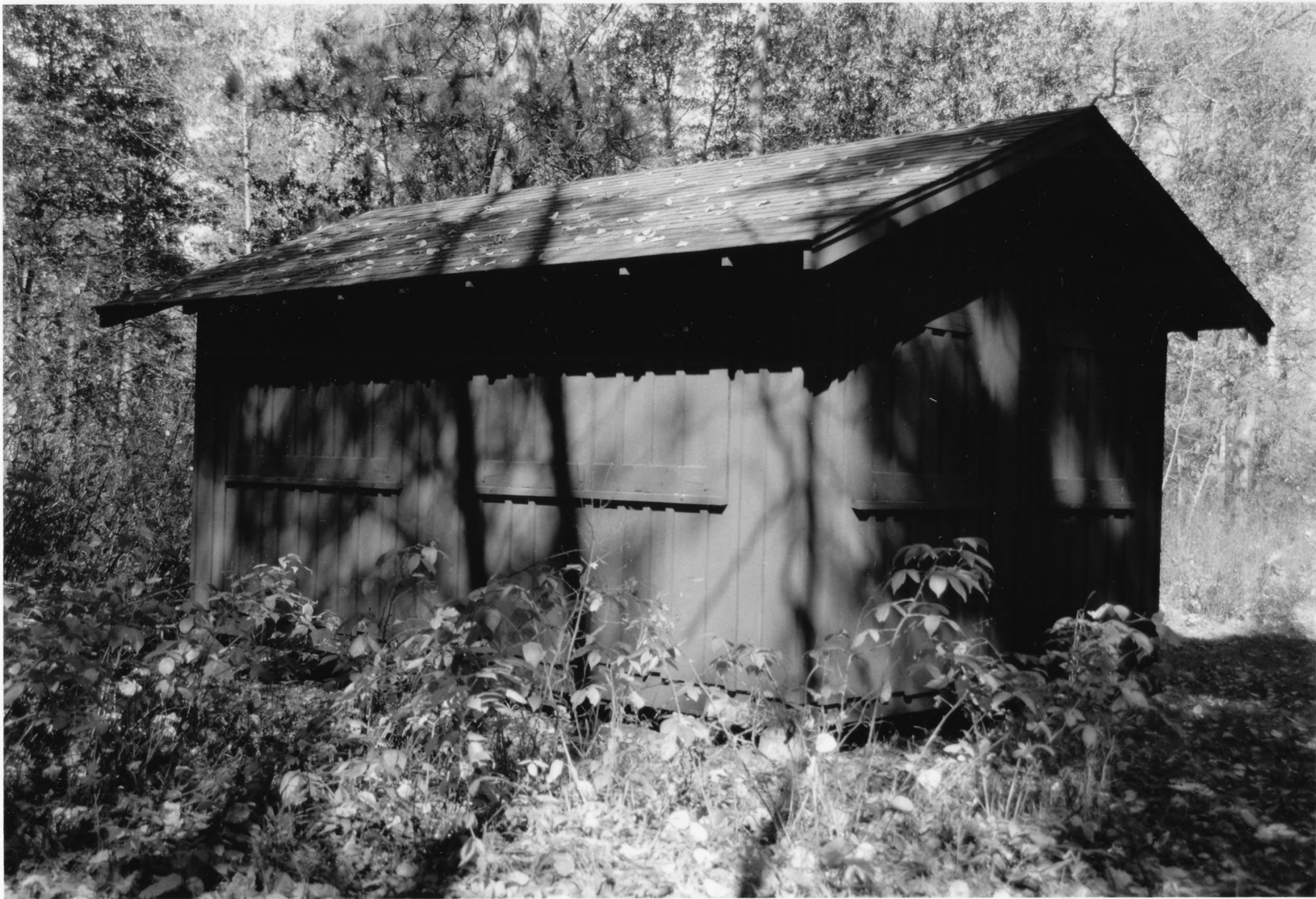
Unit Cabin #66 St. Croix Recreational Demonstration Area Pine Co., Mn 012662-23
