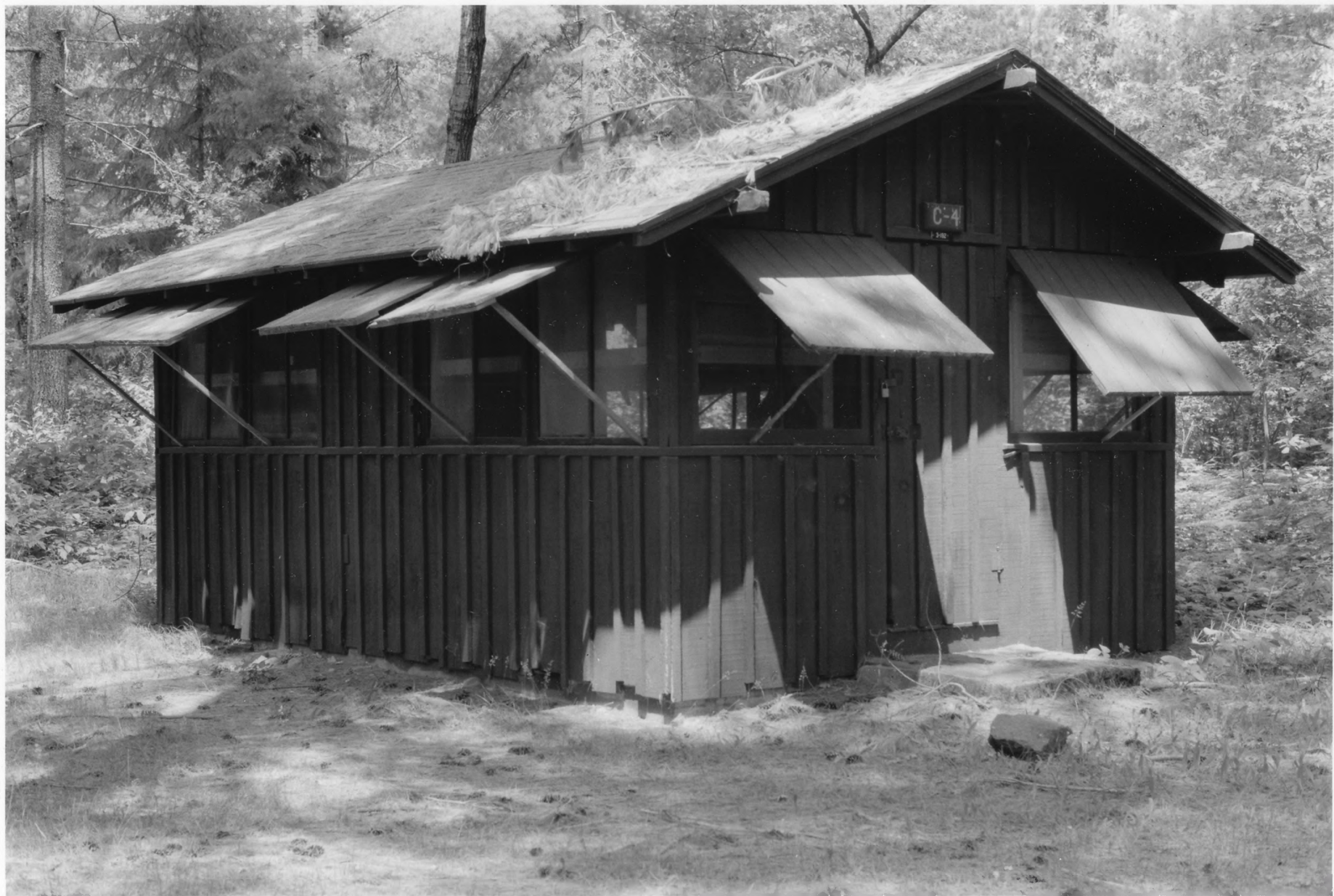
Unit Cabin #46 St. Croix Recreational Demonstration Area Pine Co. Mn 012610-7
