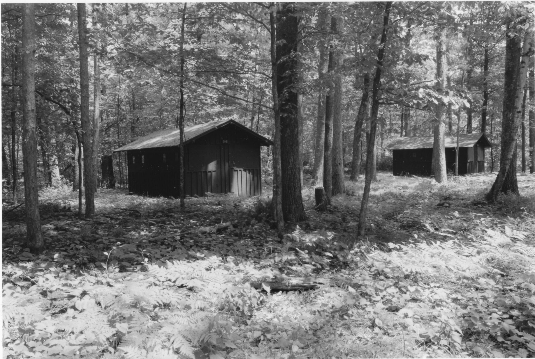
Unit Cabins # 46 St. Croix Recreational Demonstration Area Pine Co., Mn 012610-9
