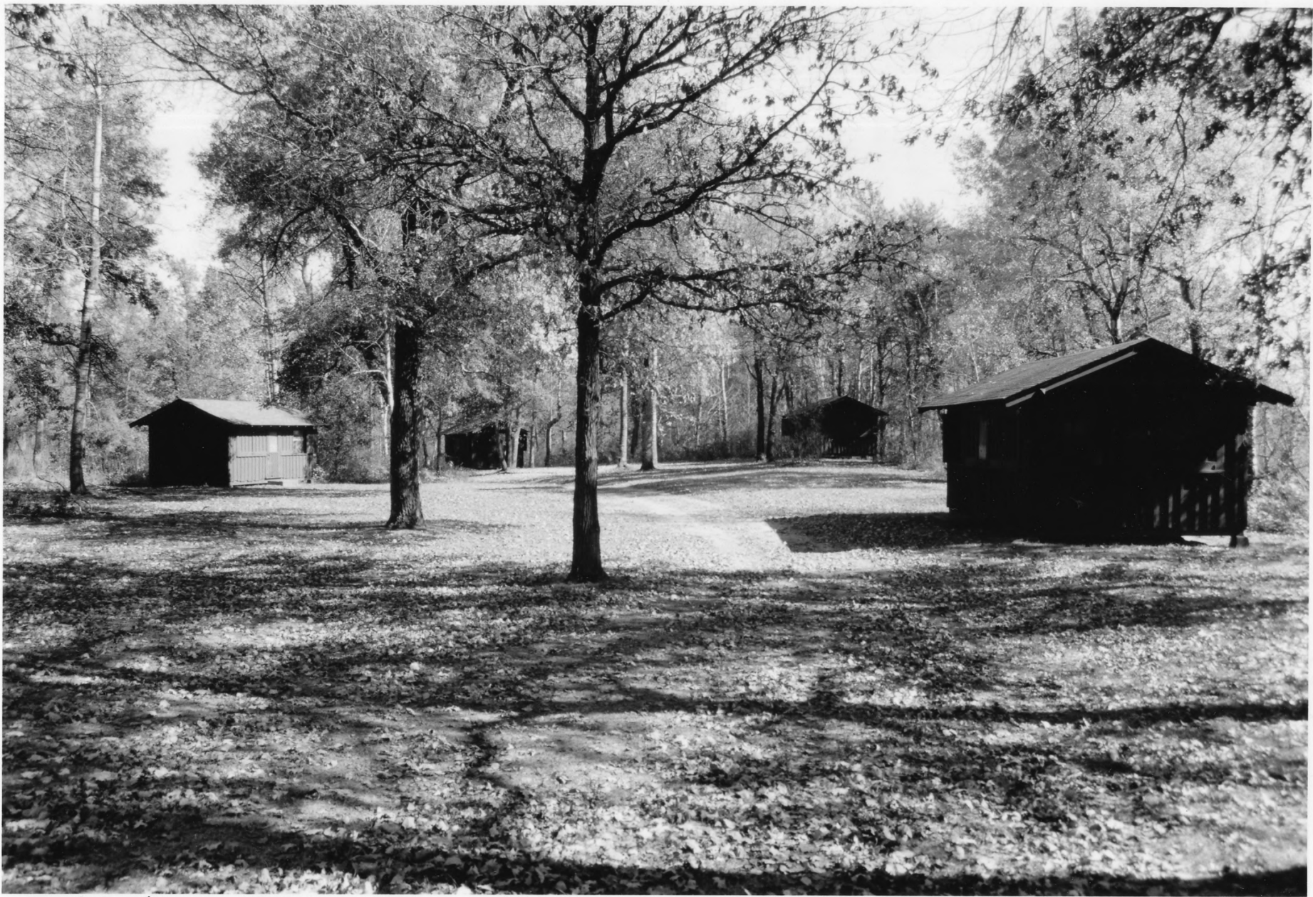
Unit Cabins #66 St. Croix Recreational Demonstration Area Pine Co., Mn 012662-18
