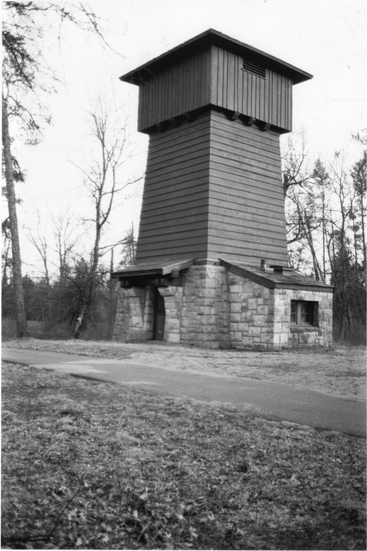
ST. CROIX STATE PARK PINE CO. MN STRUCTURE # 9 PHOTO I.D. 09581 # 6
