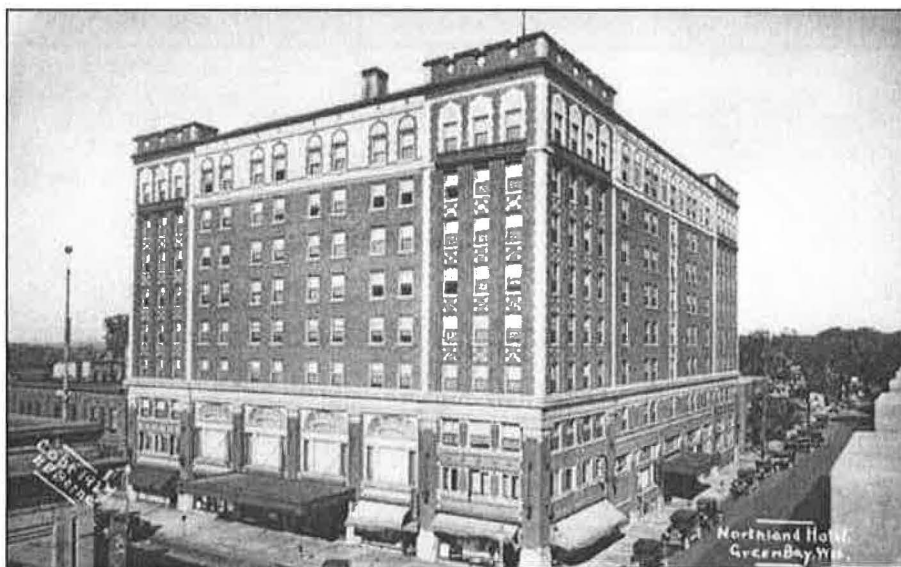
Figure 2: Hotel Northland, west and south elevations, c. 1924 (Neville Public Museum)
