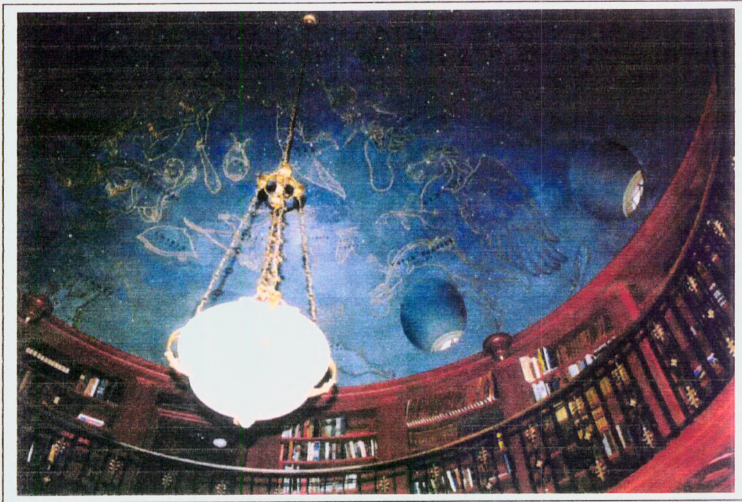
Photo 10 Library rotunda before installation of sprinklers.
