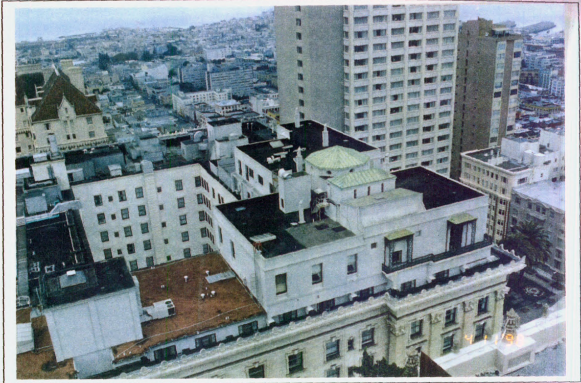
Photo 11 Fairmont Hotel viewed from above, looking northeast (photo taken from Mark Hopkins Hotel).
