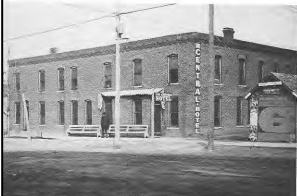
The Central Hotel, built in the 1920s was located north of the Municipal Building. It was closed in August 1941 and demolished in the early 1970s to make way for First National Bank parking.
