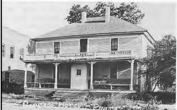
The Cottage Hotel was located on South Jackson, east of the present library building.
