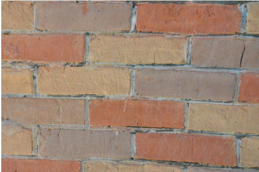
Photograph 15 of 17. Detail of exterior painted brick. Camera facing south.
