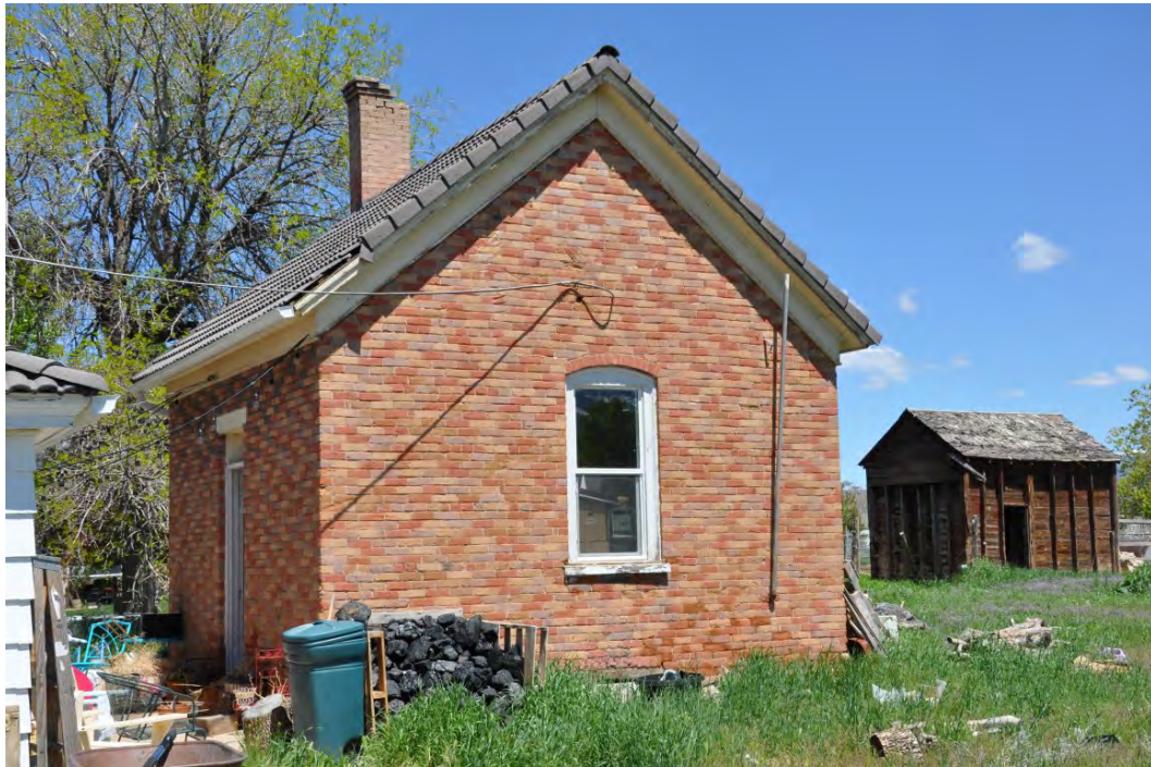
Photograph 16 of 17. Boiler house west and south elevations. Camera facing northeast.
