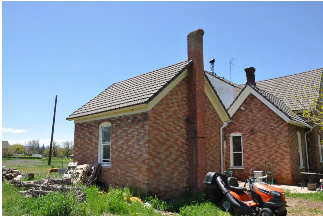
Photograph 17 of 17. Boiler house, east and north elevations. Camera facing southwest.
