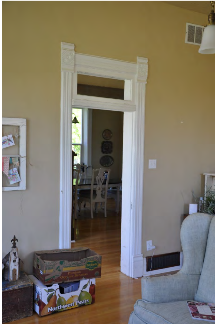
Photograph 10 of 17. Detail of interior door/transom and wood trim in parlor. Camera facing north.
