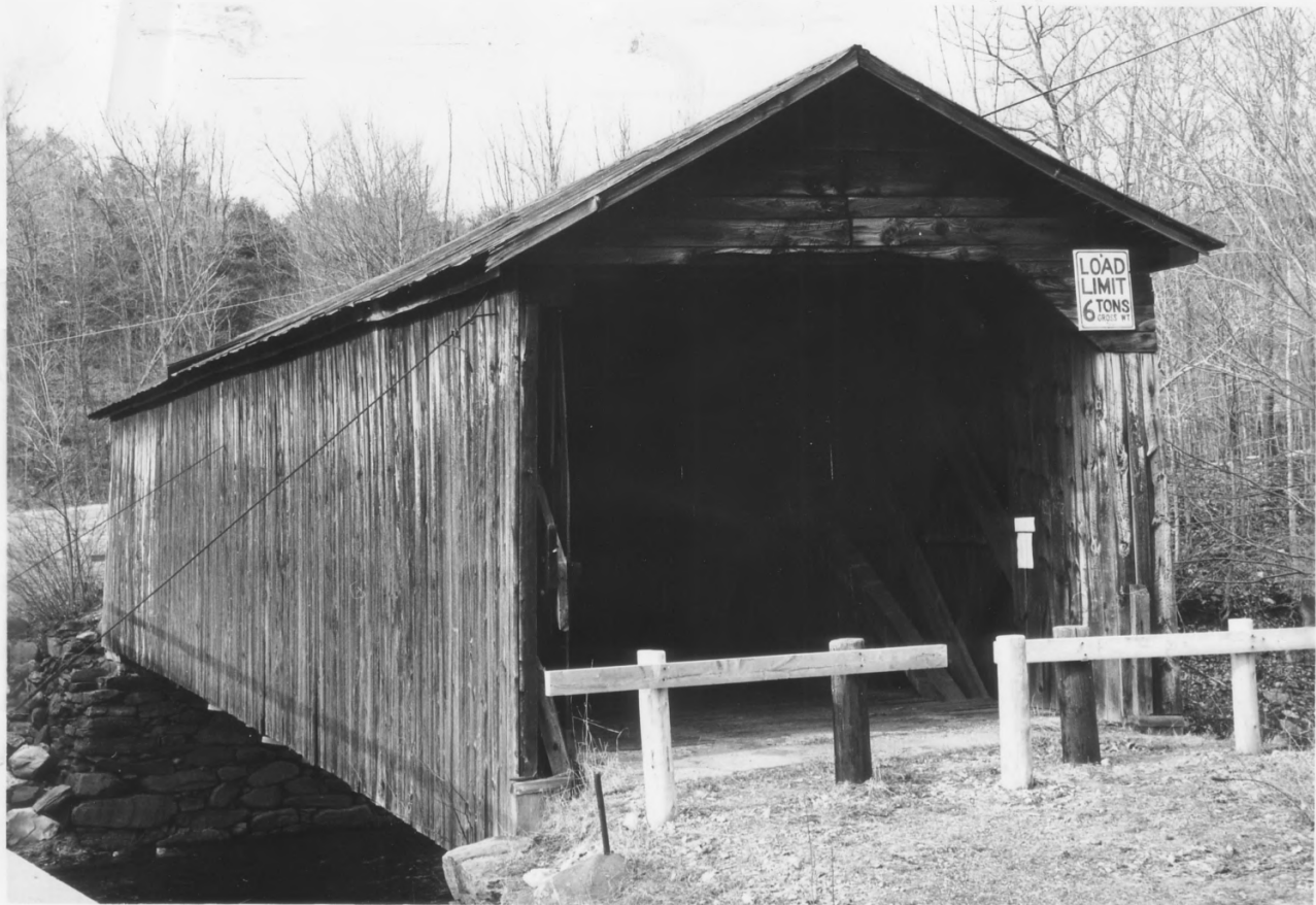
Old River Bridge
