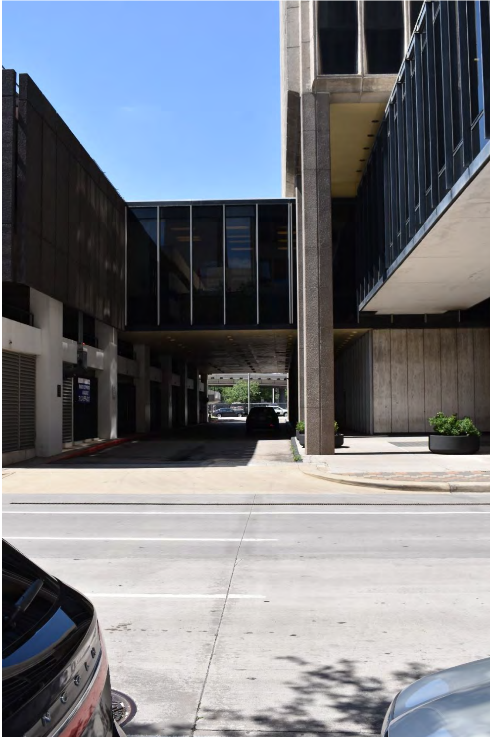
Photo 4 (TX_HarrisCounty_500Jefferson_0004) Connection between office tower and garage, view west
