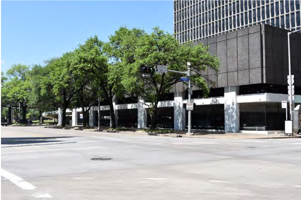
Photo 6 (TX_HarrisCounty_500Jefferson_0006) South (rear) elevation of garage, view northwest
