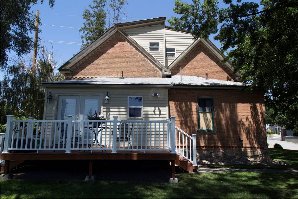
5 of 15. View of south (rear) façade. Camera facing north.
