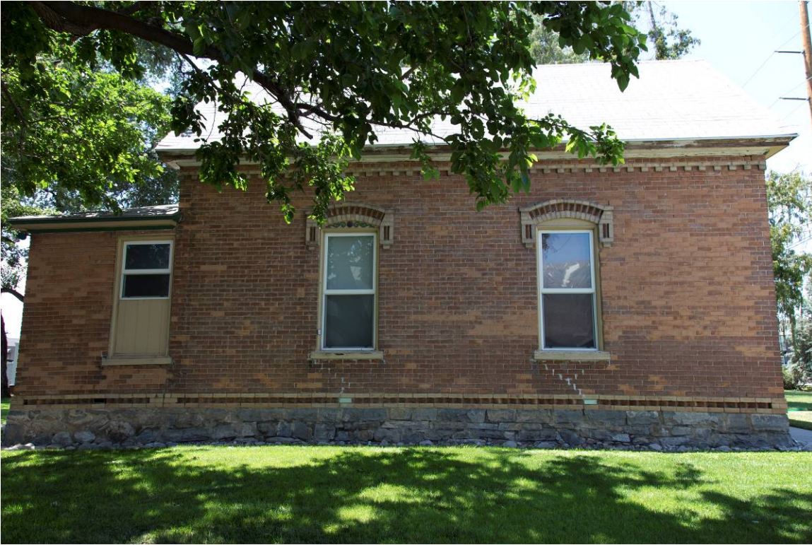
7 of 15. View of east façade. Camera facing west.
