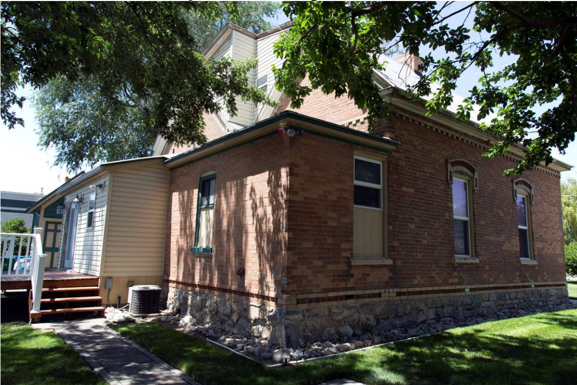
6 of 15. View of southeast façade. Camera facing northwest.
