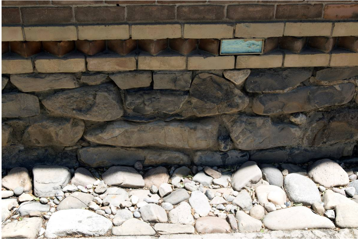
13 of 15. Foundation and lower decorative brick course detail. Camera facing north.
