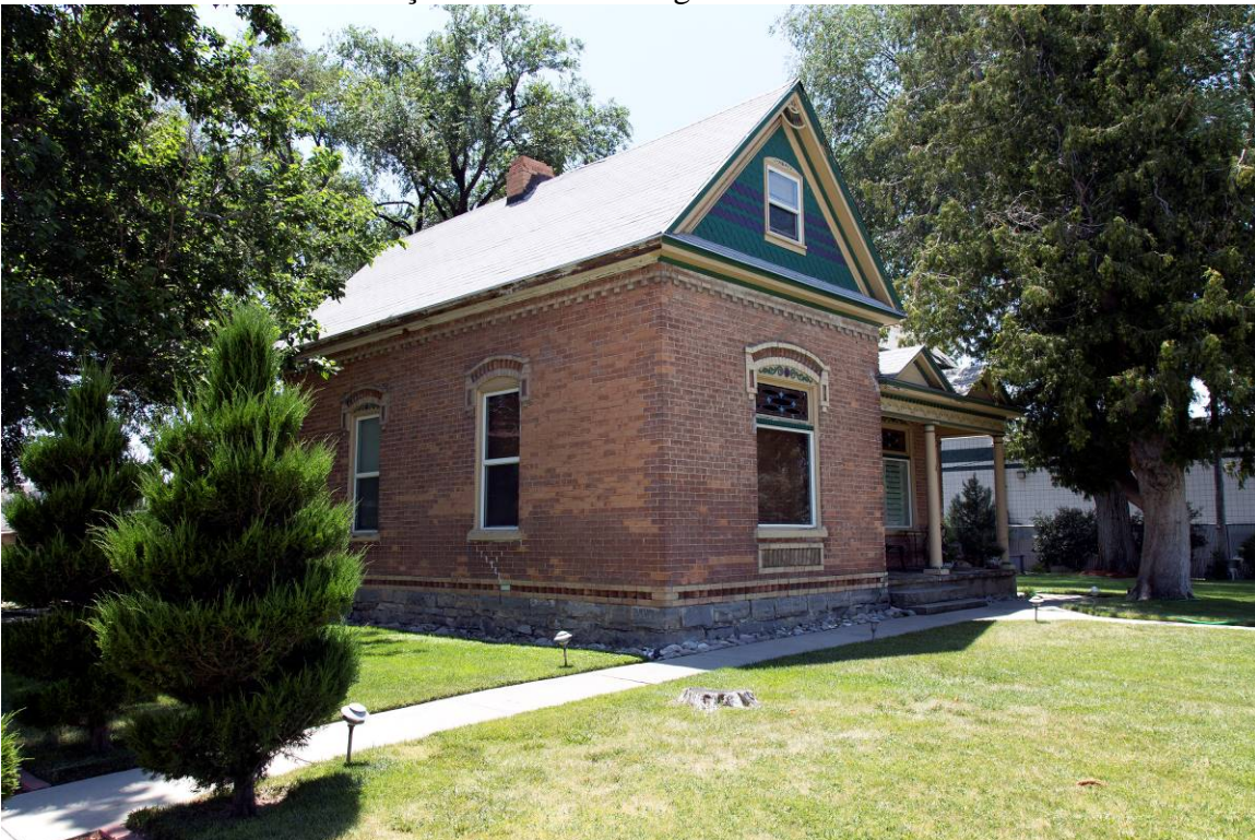
8 of 15. View of northeast façade. Camera facing southwest.
