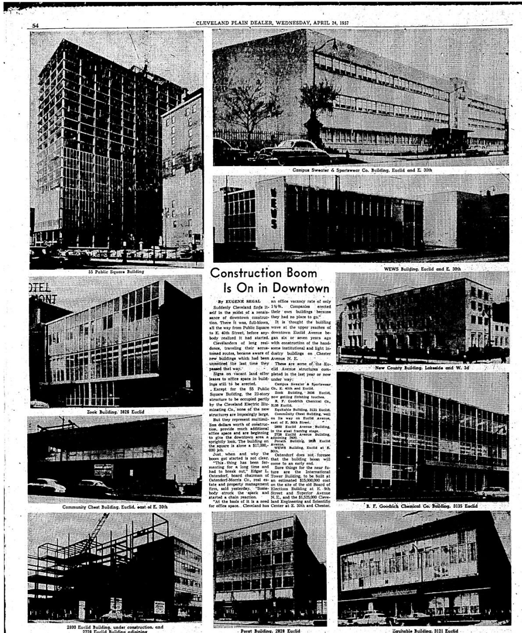
Figure 4. 1955-1959 Construction Boom on Euclid Avenue to the east of the I-90 Inner Belt
