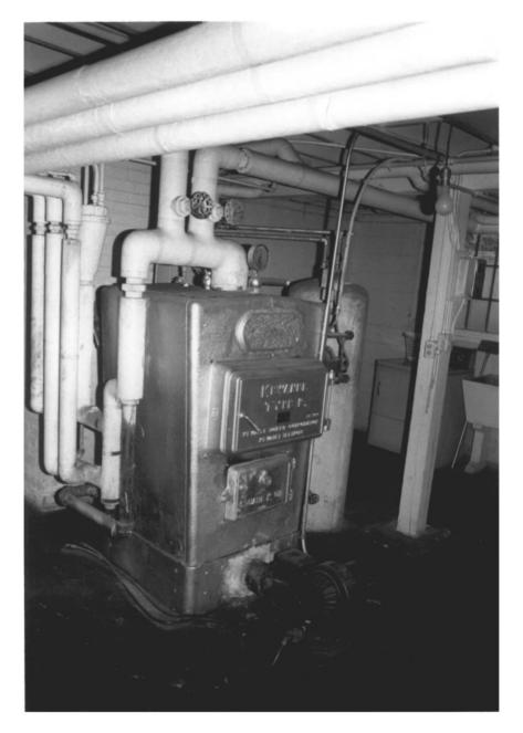
20 of 20 Deisel-powered heating plant, basement.
