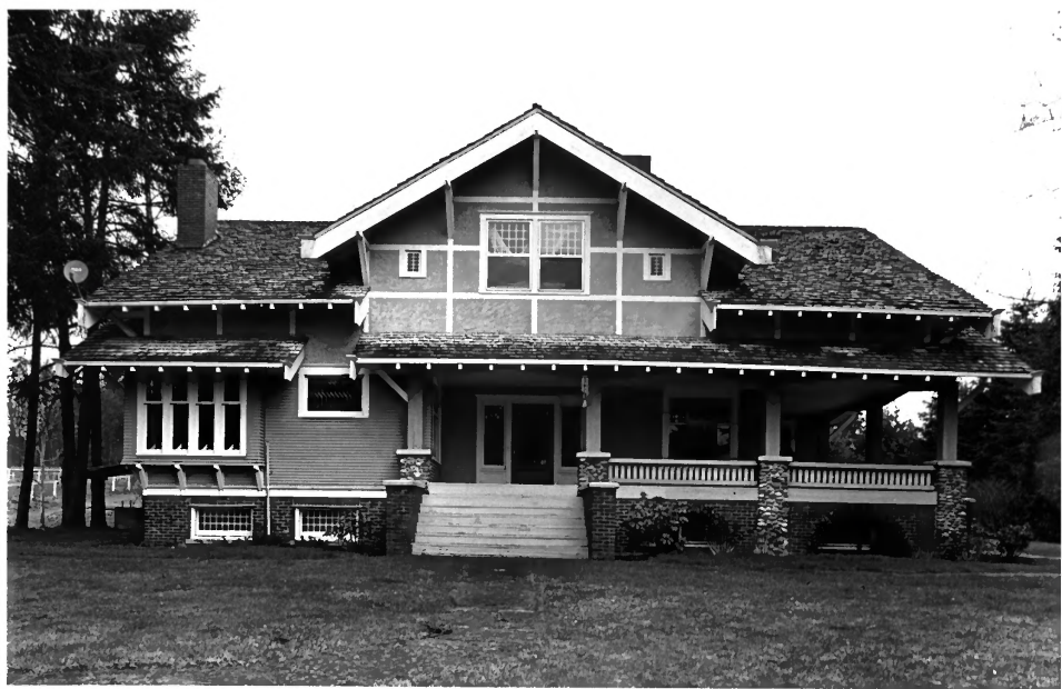
HELMER + SELMA STEEN HOUSE VASHON, WA
