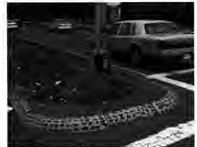
Quarter-round Belgian-block curbing along the median strip at Spring Street, Everett (ca. 1955).
