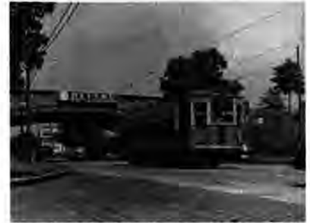
Broadway Bridge, Revere, looking north, ca. 1950. 7
