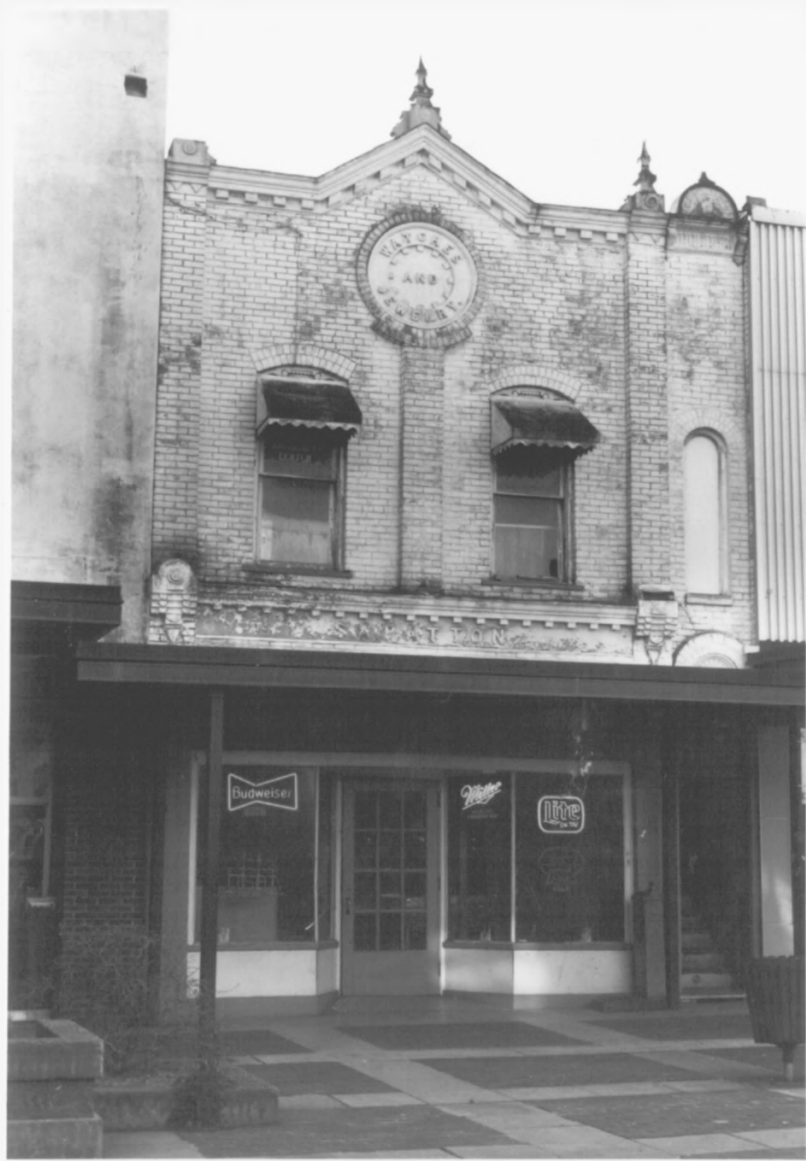
Patton, Samuel A., Building, Blount Co., TN, Photo 1 of 2
