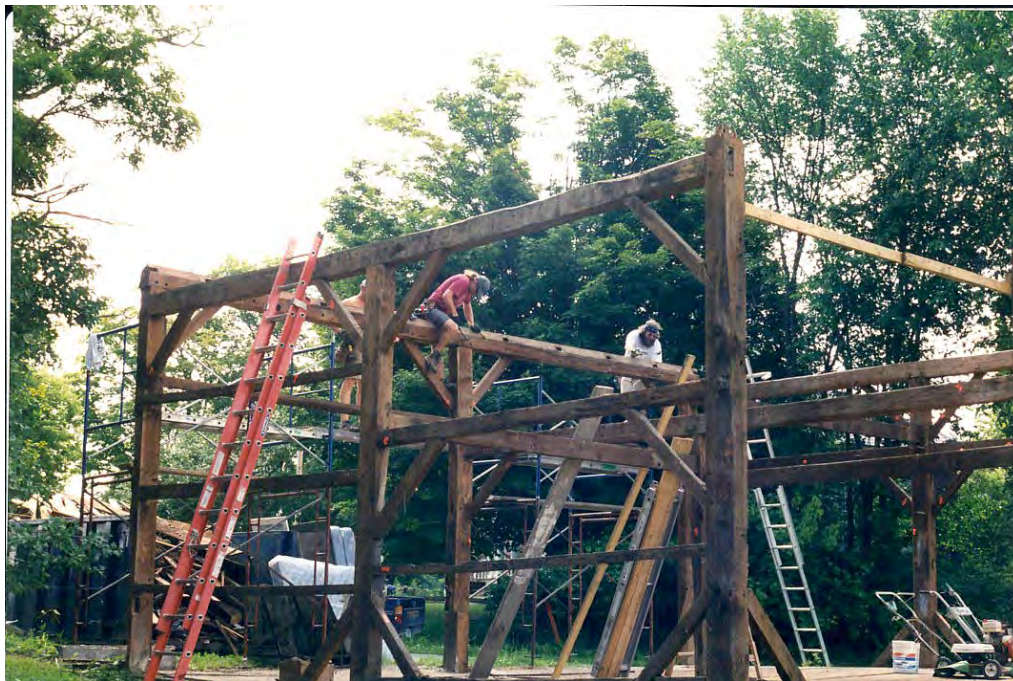
Figure 3. Barn during deconstruction (owner's personal collection).
