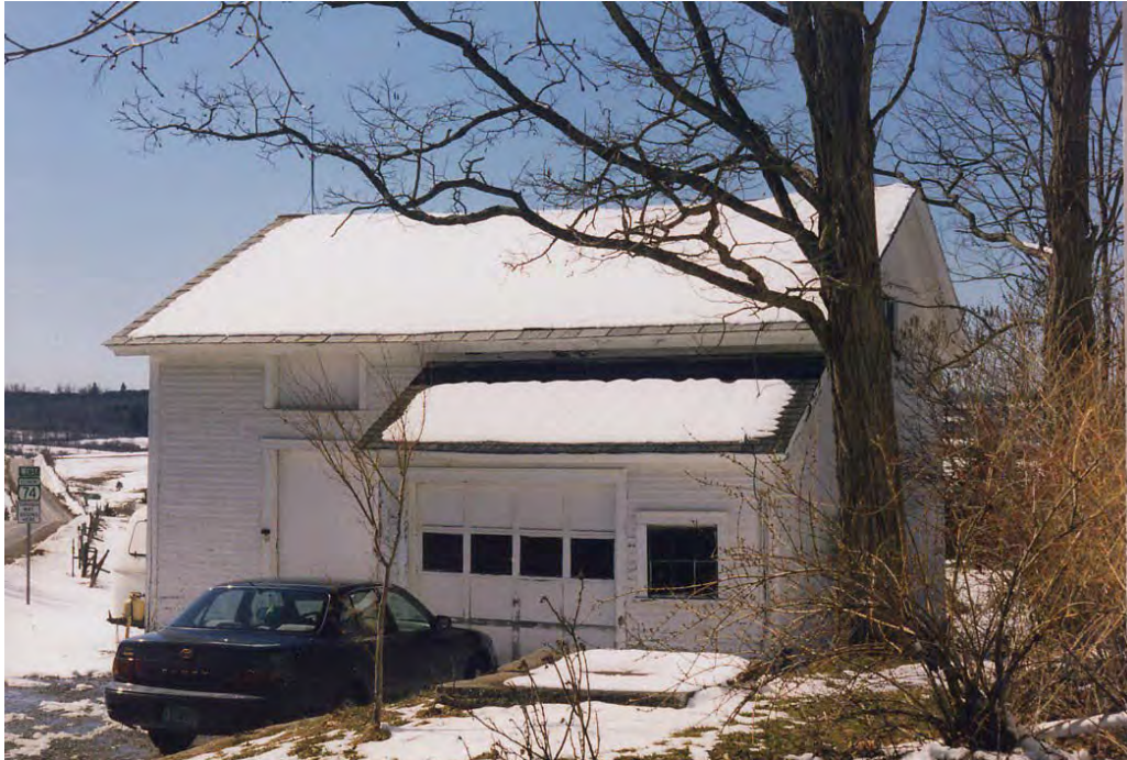
Figure 1. Barn prior to deconstruction, view southwest, c.2000 (owner's personal collection).
