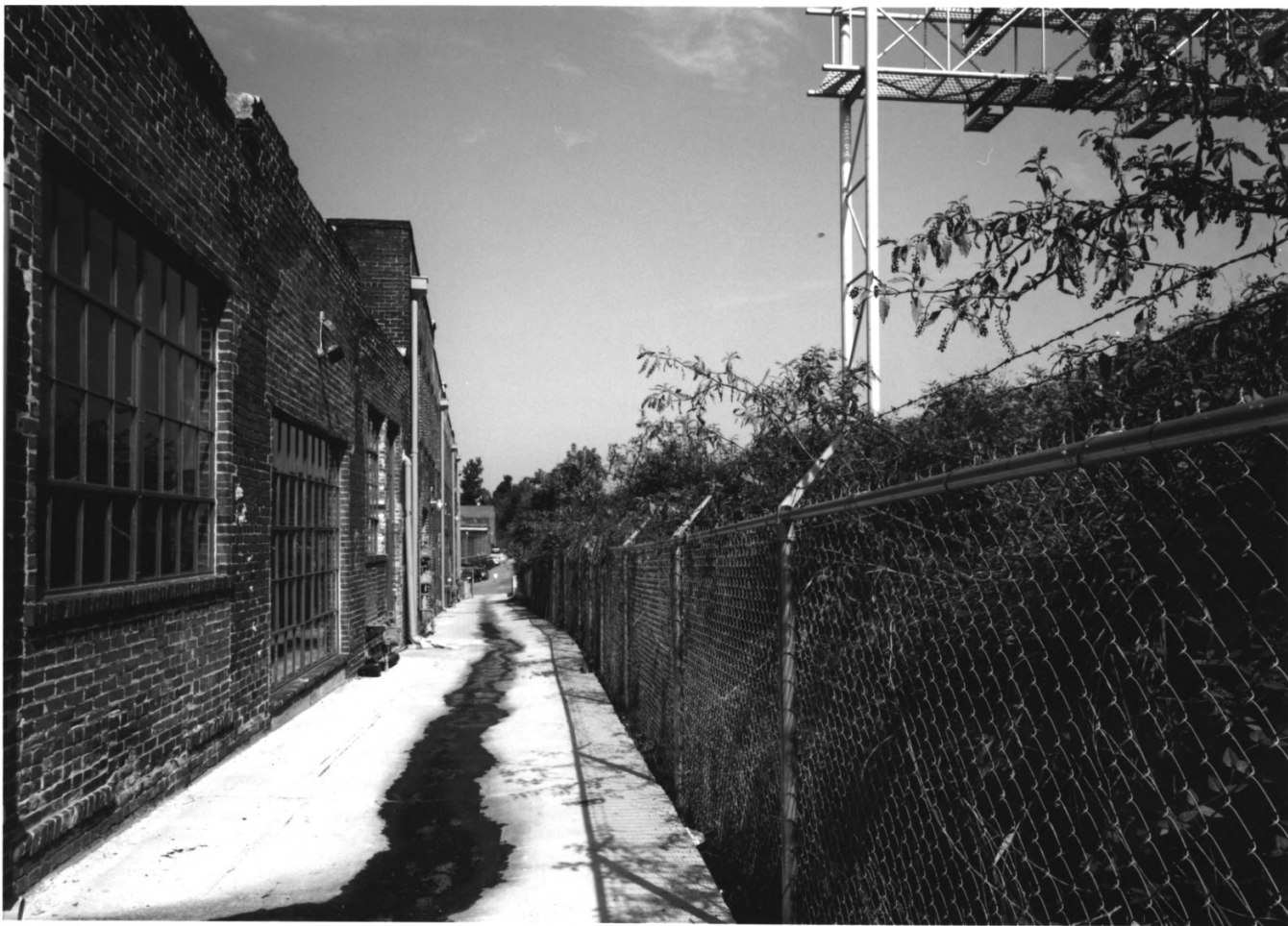
King Plow Company, Atlanta, Fulton County, Georgia 10 of 18
