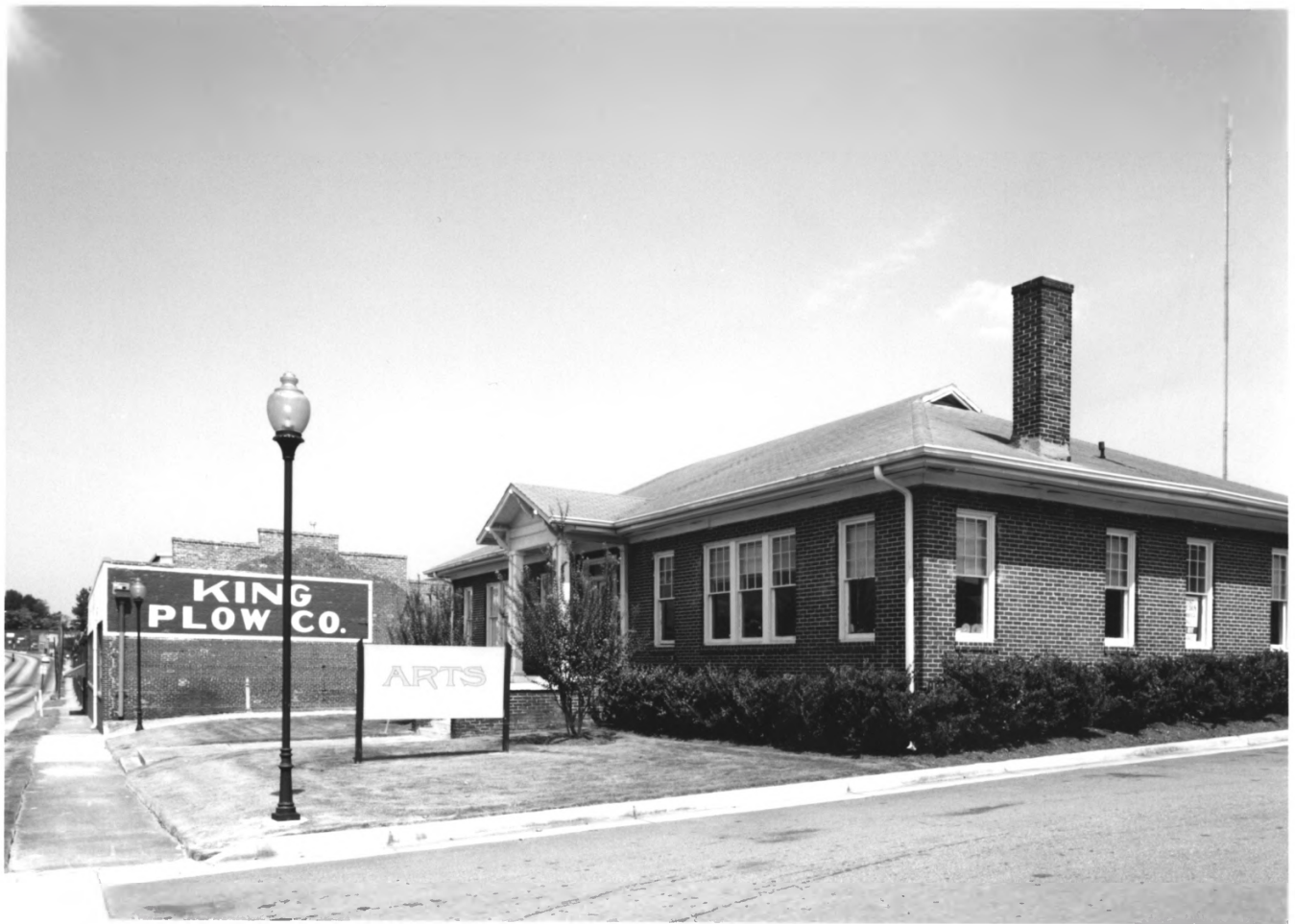
King Plow Company, Atlanta, Fulton County, Georgia 3 of 18
