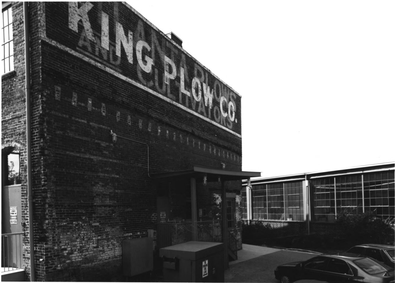
King Plow Company, Atlanta, Fulton County, Georgia 4 of 18
