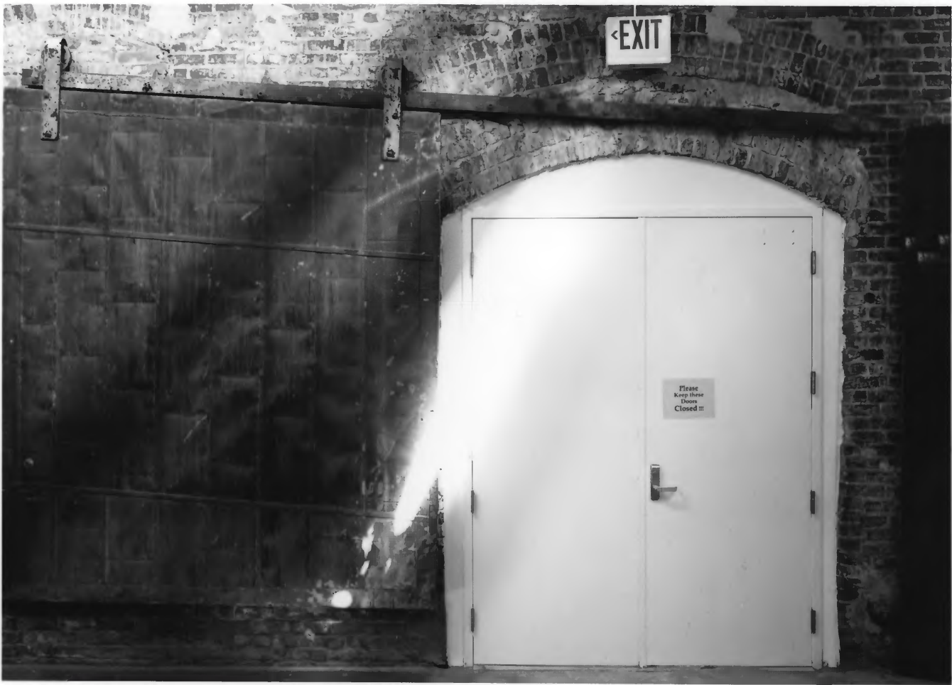
King Plow Company, Atlanta, Fulton County, Georgia 17 of 18
