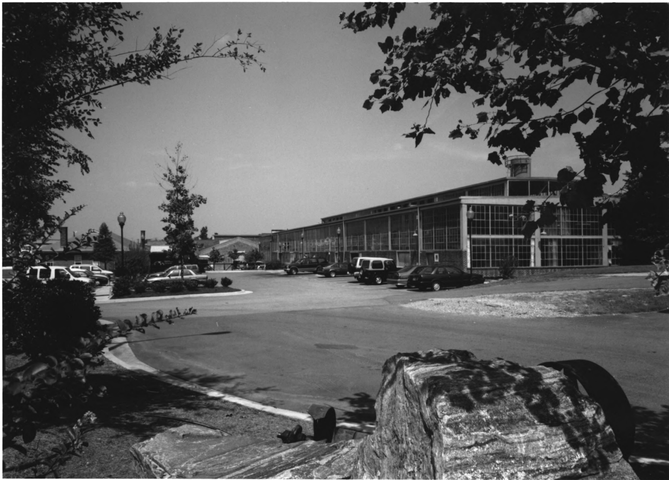
King Plow Company, Atlanta, Fulton County, Georgia 11 of 18
