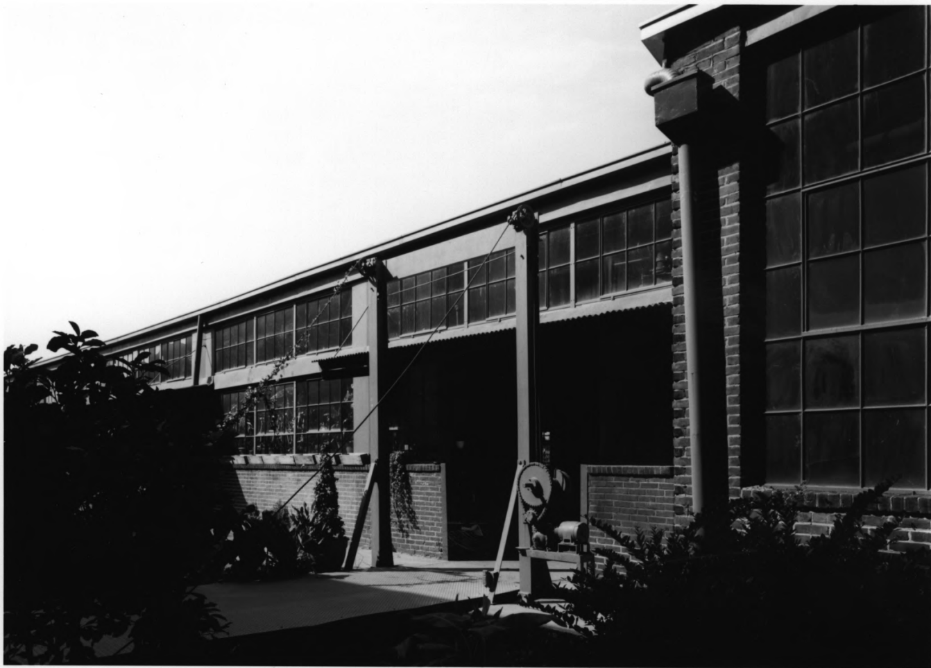
King Plow Company, Atlanta, Fulton County, Georgia 5 of 18
