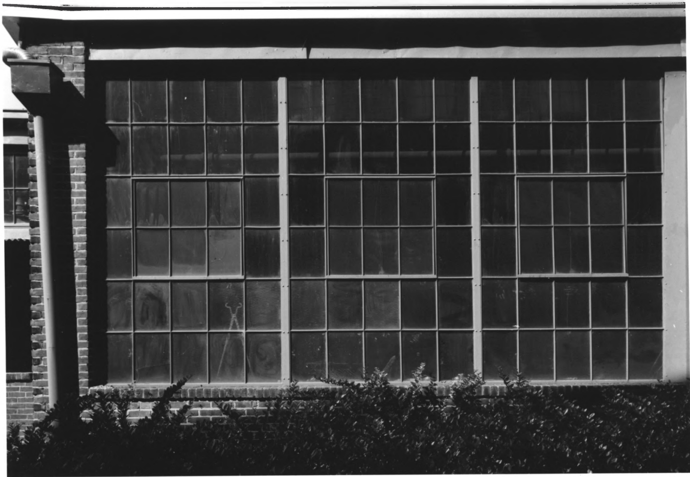
King Plow Company, Atlanta, Fulton County, Georgia 6 of 18
