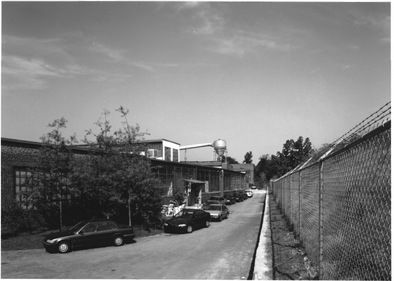
King Plow Company, Atlanta, Fulton County, Georgia 9 of 18
