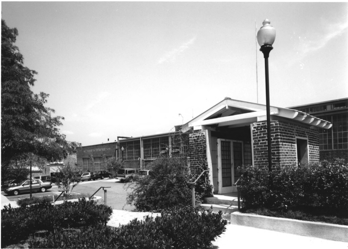
King Plow Company, Atlanta, Fulton County, Georgia 12 of 18
