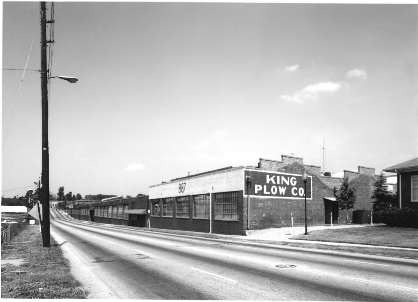
King Plow Company, Atlanta, Fulton County, Georgia 2 of 18
