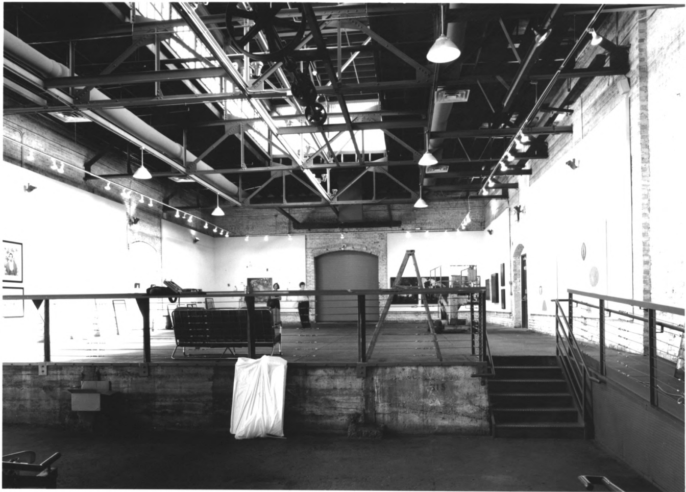
King Plow Company, Atlanta, Fulton County, Georgia 16 of 18
