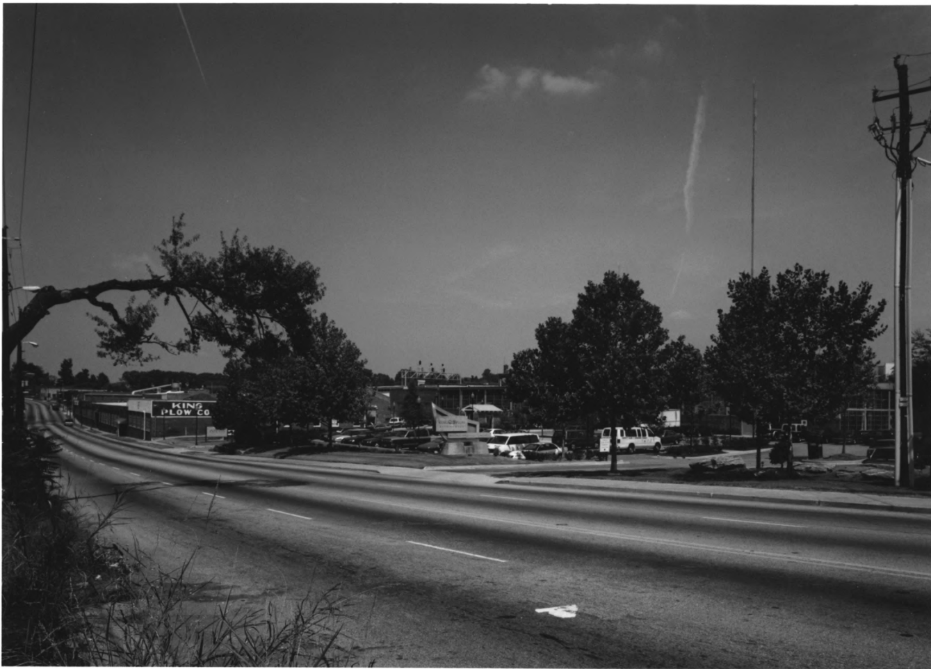
King Plow Company, Atlanta, Fulton County, Georgia 1 of 18
