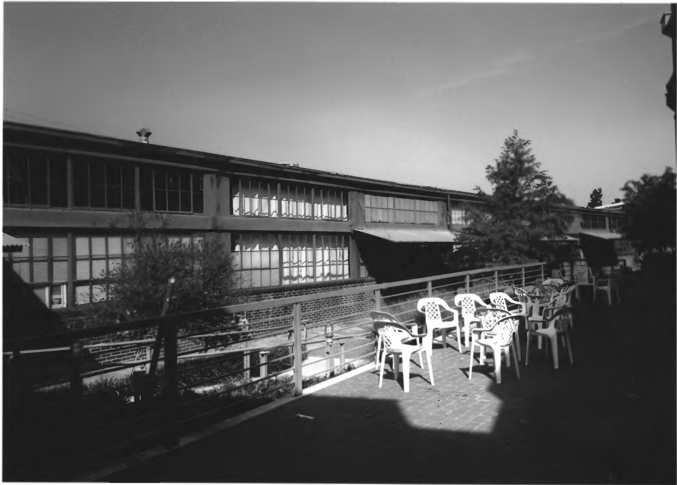
King Plow Company, Atlanta, Fulton County, Georgia 8 of 18
