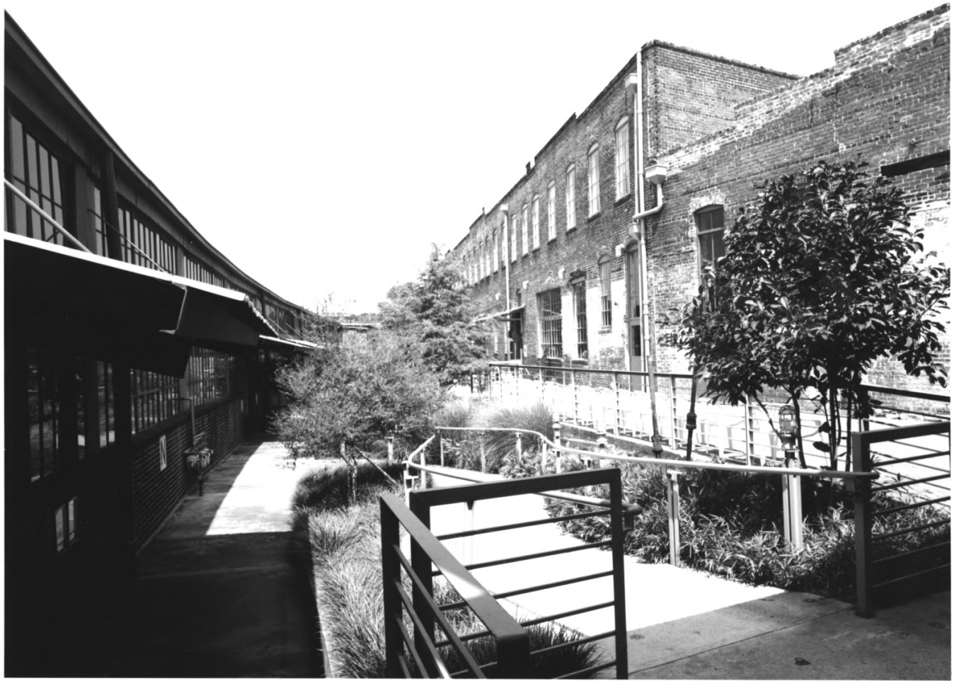
King Plow Company, Atlanta, Fulton County, Georgia 7 of 18
