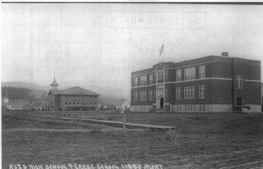
Libby High School (right) and grade school prior to the construction on the auditorium wing of the high school, c. 1917. View to southeast.
