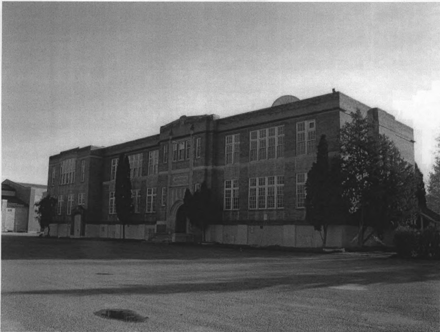
North and west elevations of Libby High School, view to southeast. Photo by Chere Justo, 2006.
